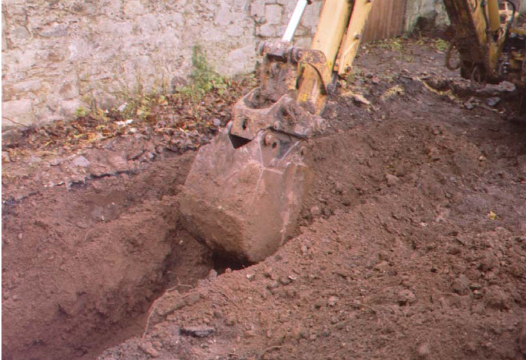
Figure 4: The digging of the footing trenches
