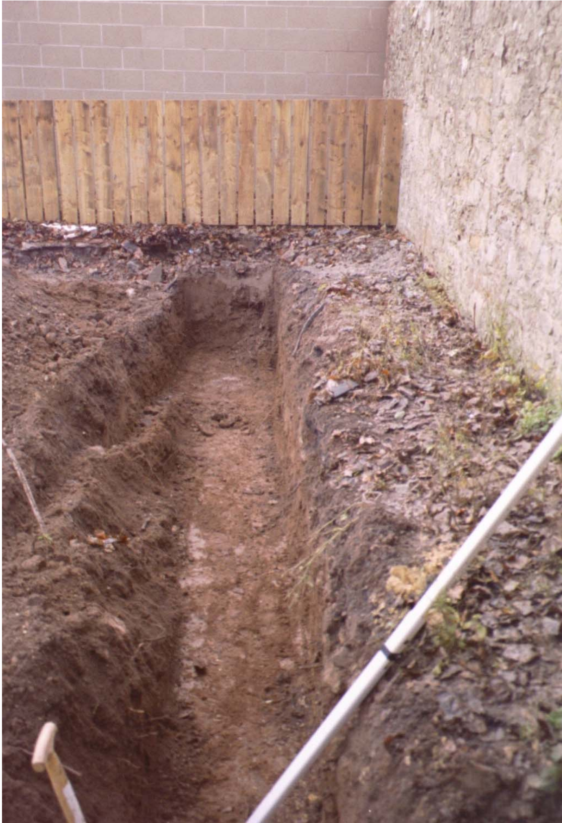
Figure 6: The westernmost footing trench
