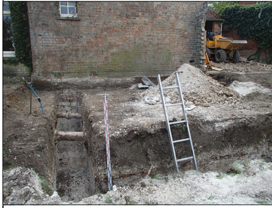
Foundation trenches to the new garden room, view south-east
