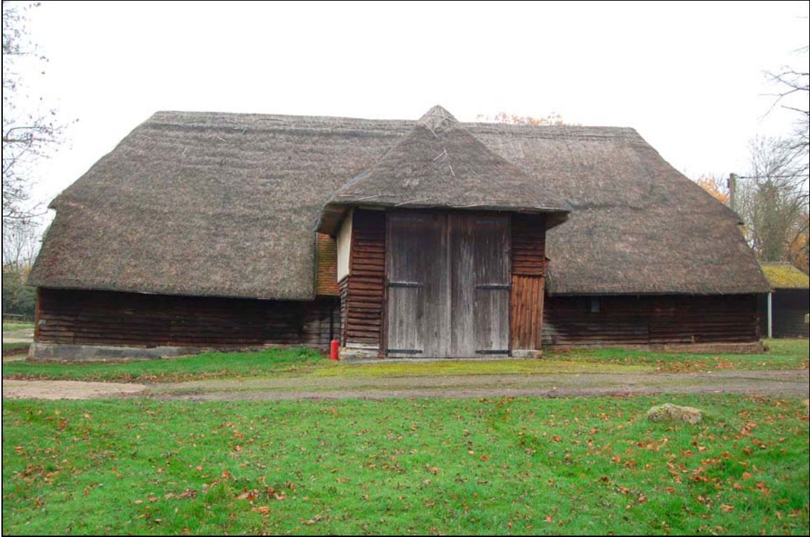
Plate 1 South elevation of barn
