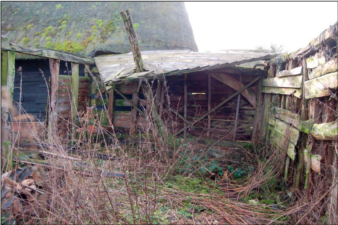
Plate 26 North part of byre viewed to south
