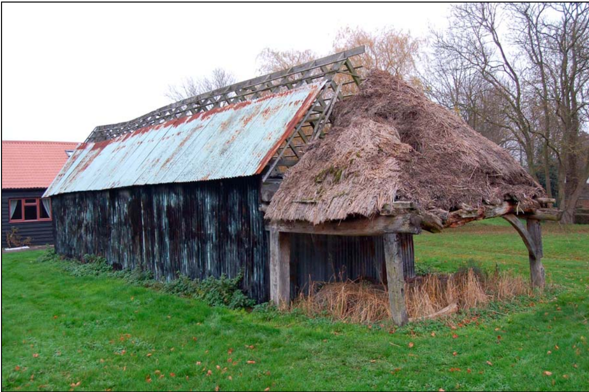
Plate 20 Cart lodge viewed to north-east
