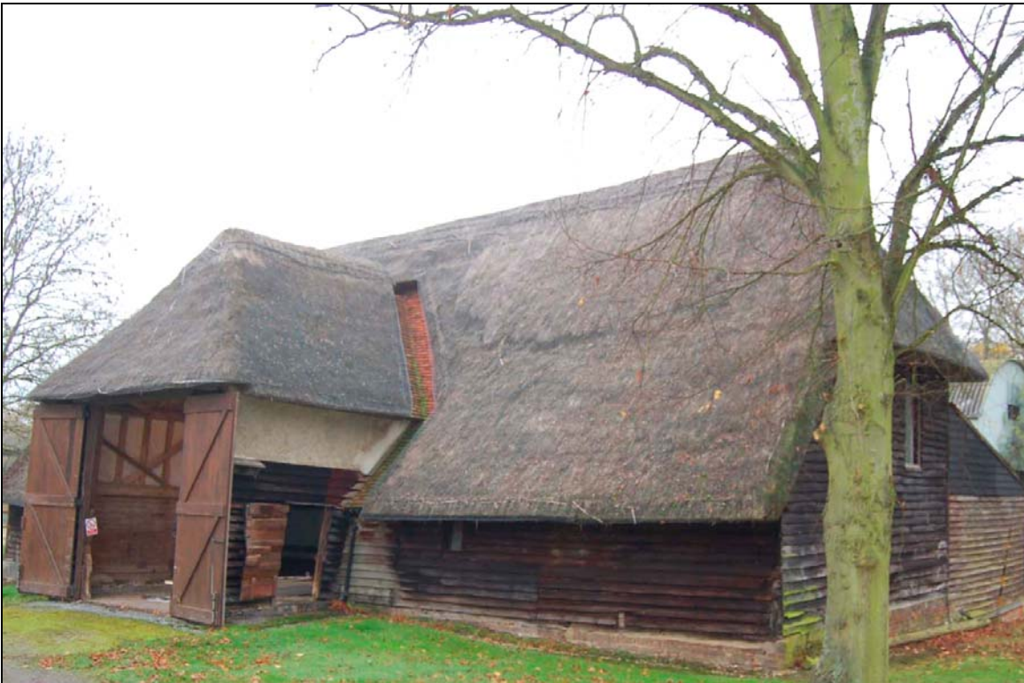
Plate 2 Barn viewed to north-west
