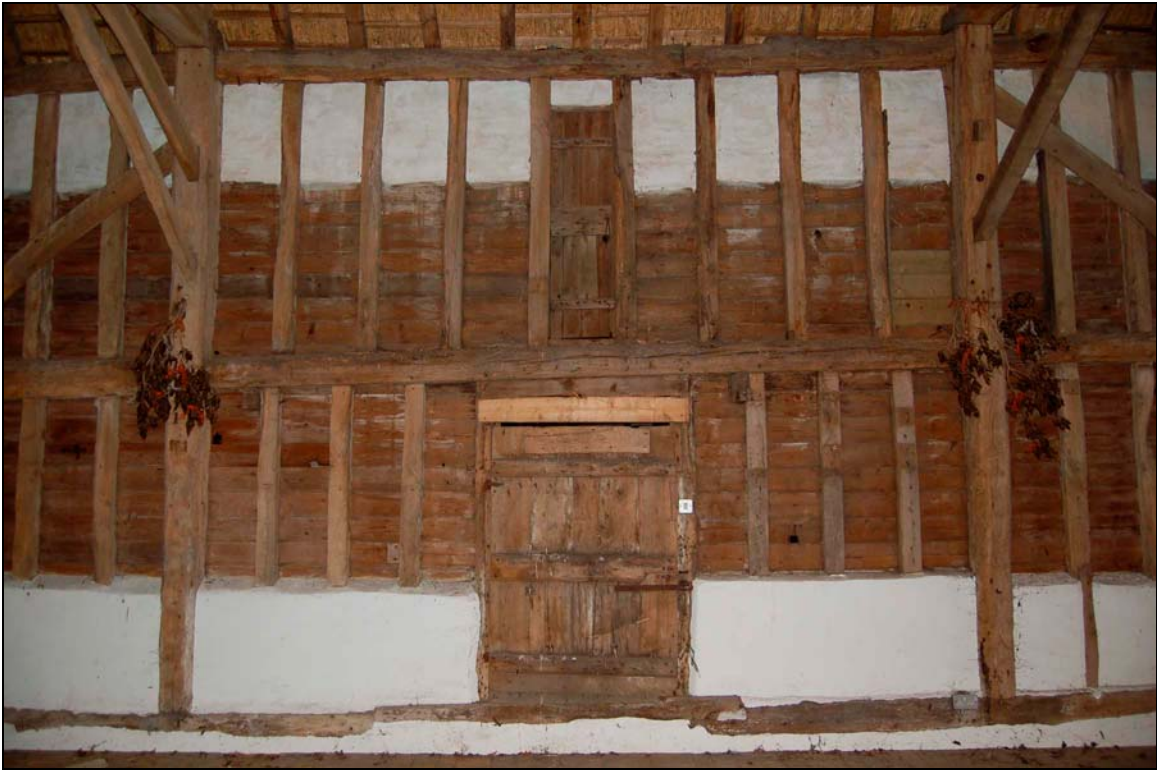
Plate 13 North door and pitching hatch
