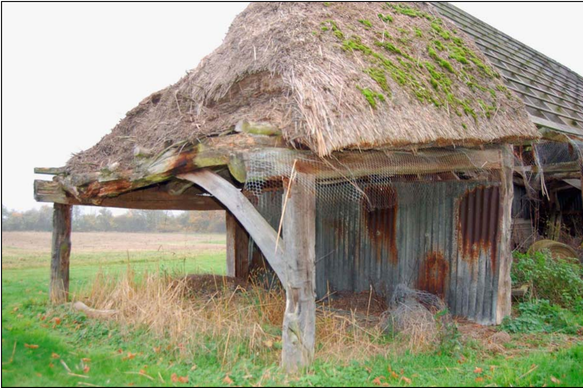
Plate 23 Hipped bay on south side of cart lodge
