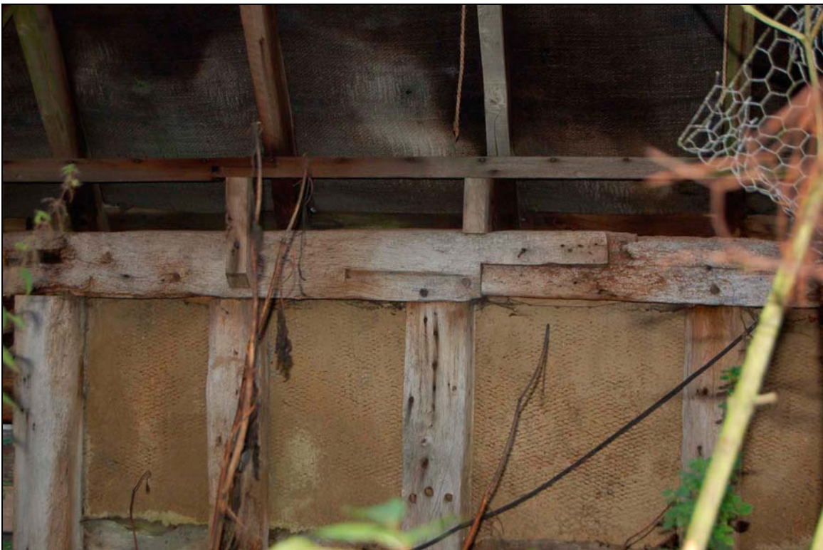
Plate 28 face-halved and bladed scarf joint along east wall of byre
