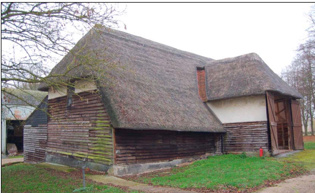
Plate 6 Barn viewed to north-east
