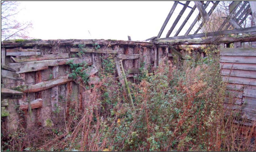
Plate 29 Close-studding along west wall of byre
