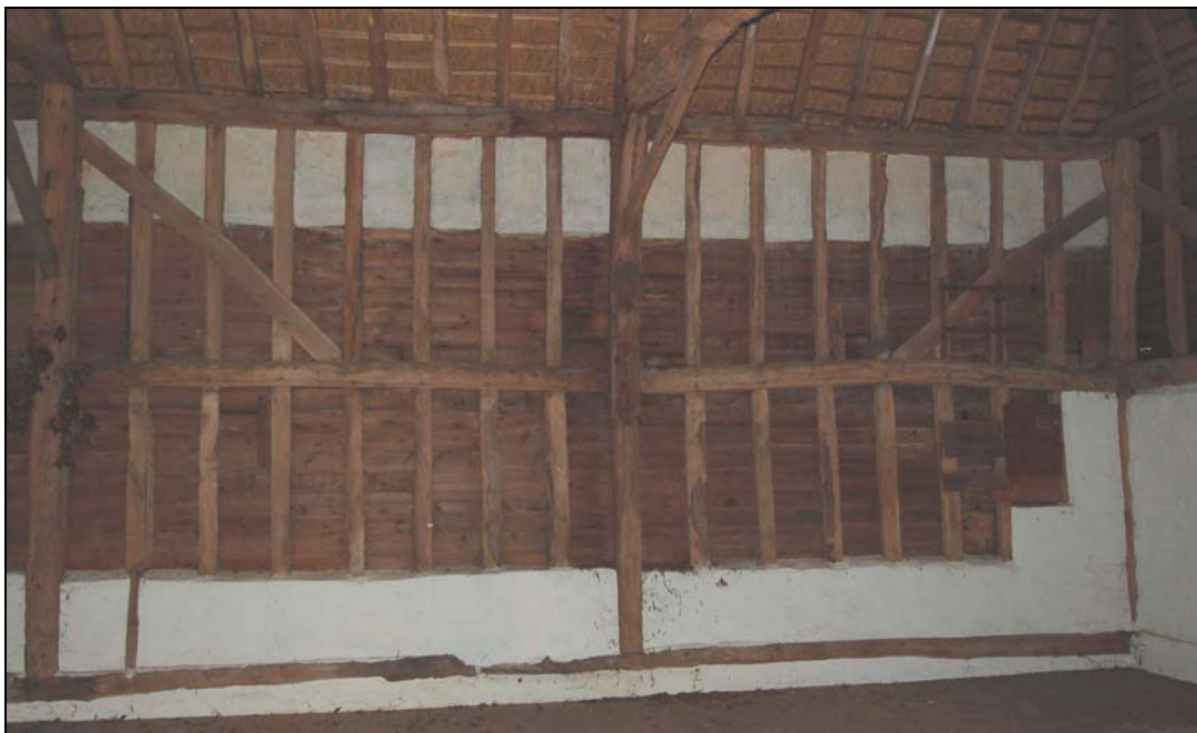
Plate 12 Typical internally-braced studwork in barn
