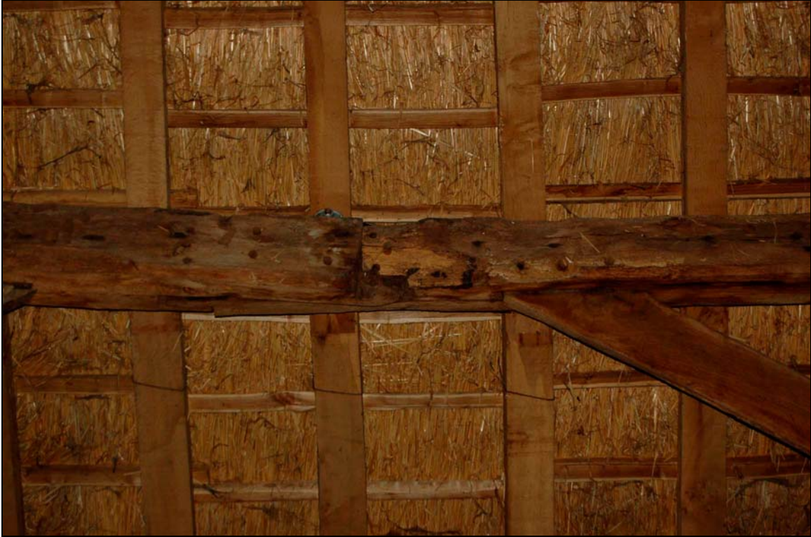
Plate 9 Six-pegged edge-halved and bladed scarf joint along aisle plate
