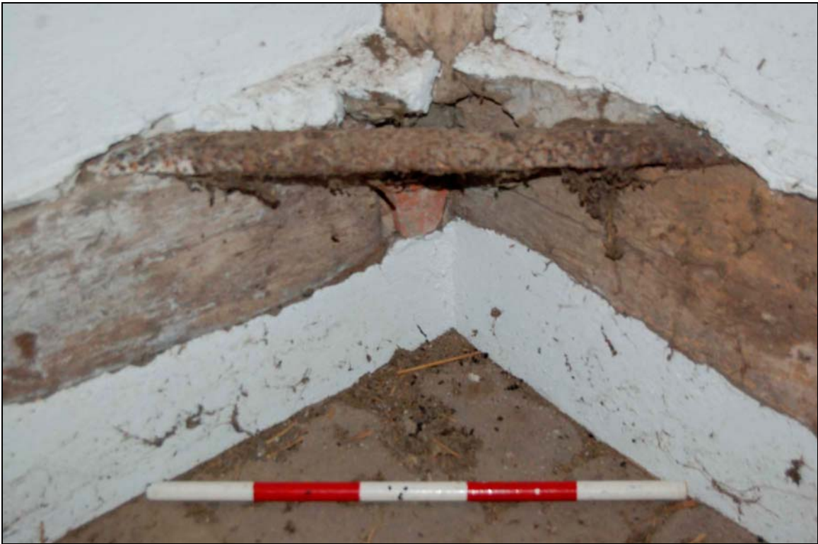
Plate 10 Iron strap in connecting sill plates in north-west corner of barn
