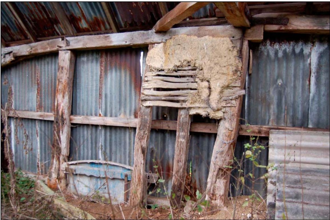
Plate 22 Daub walling inside cart lodge
