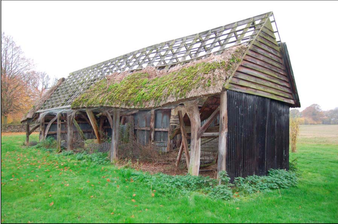
Plate 19 Cart lodge viewed to south-west
