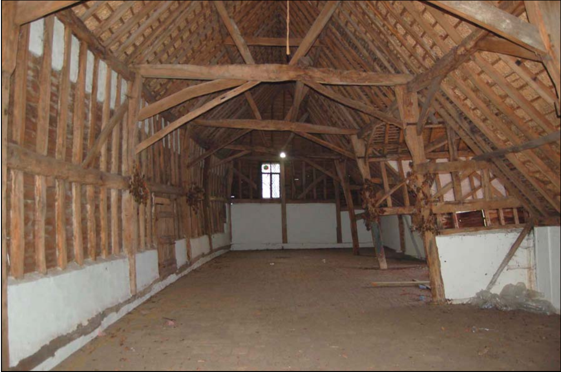
Plate 7 Interior of barn viewed to east
