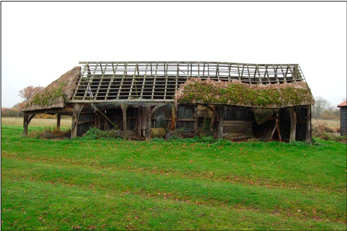
Plate 18 East elevation of cart lodge
