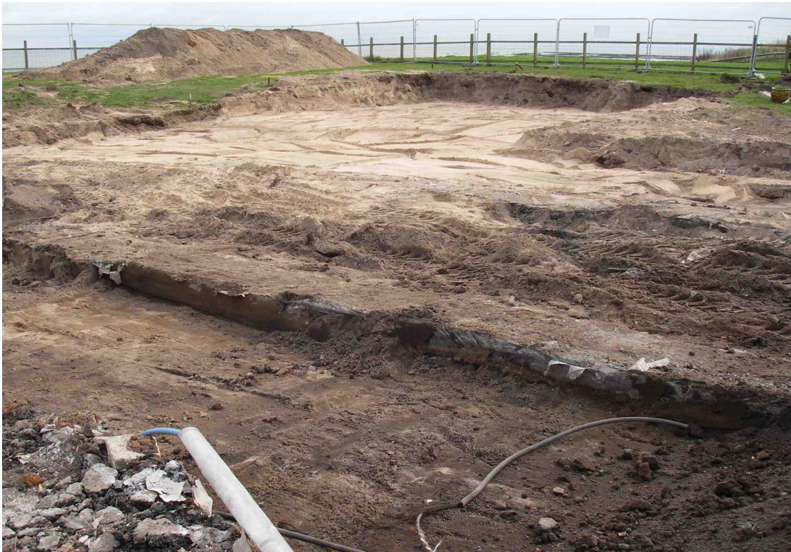
Plate 1: Development area stripped, facing south east
