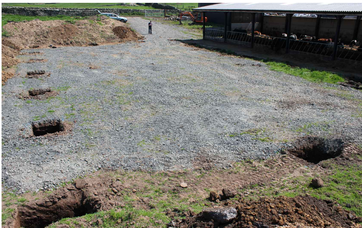
Plate 1: Foundation pits for the new building, facing east
