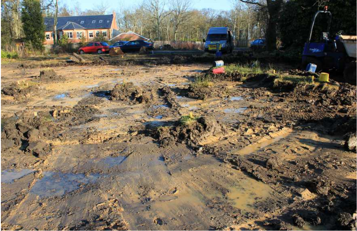
Plate 1: Topsoil stripping prior to foundation excavation, facing north
