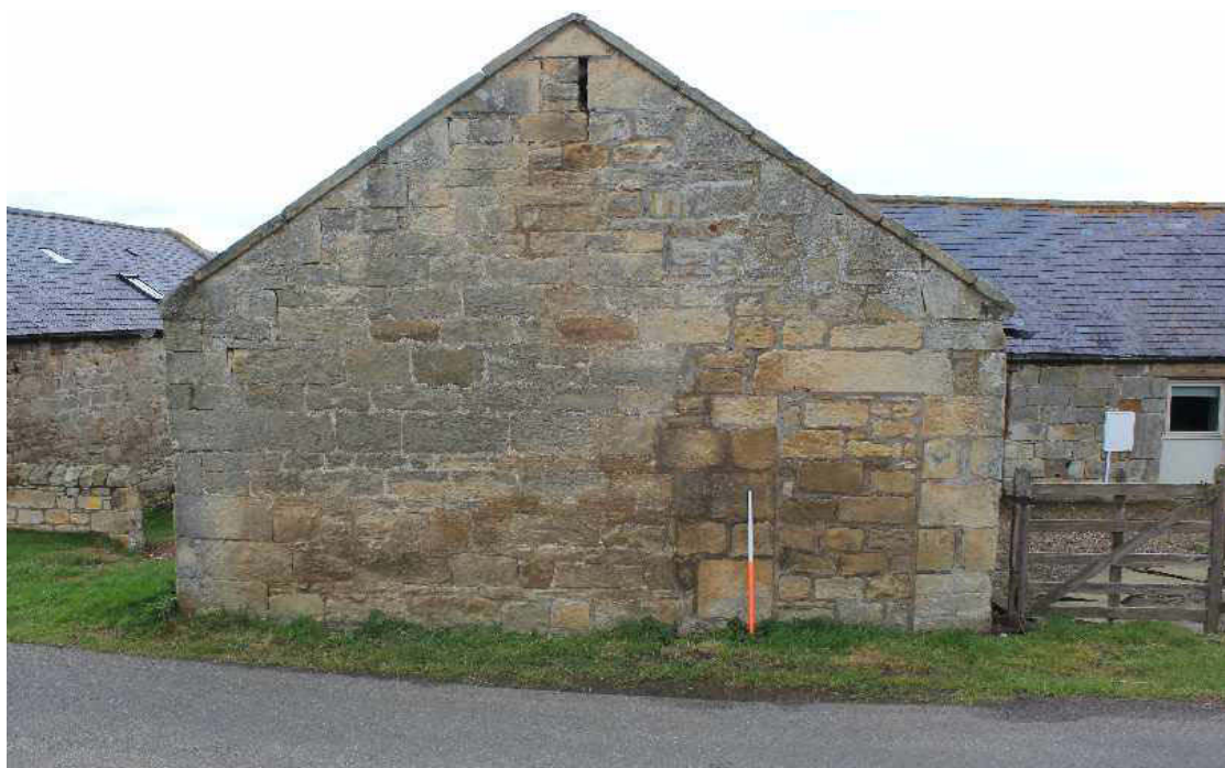
Plate 8: South end of Room E, showing blocked doorway, facing north
