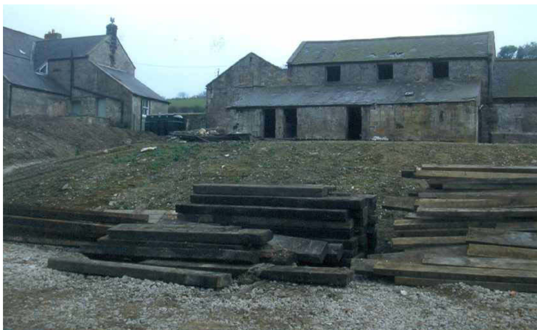
Plate 7: The north side of Room F with extensions I and L, facing south
