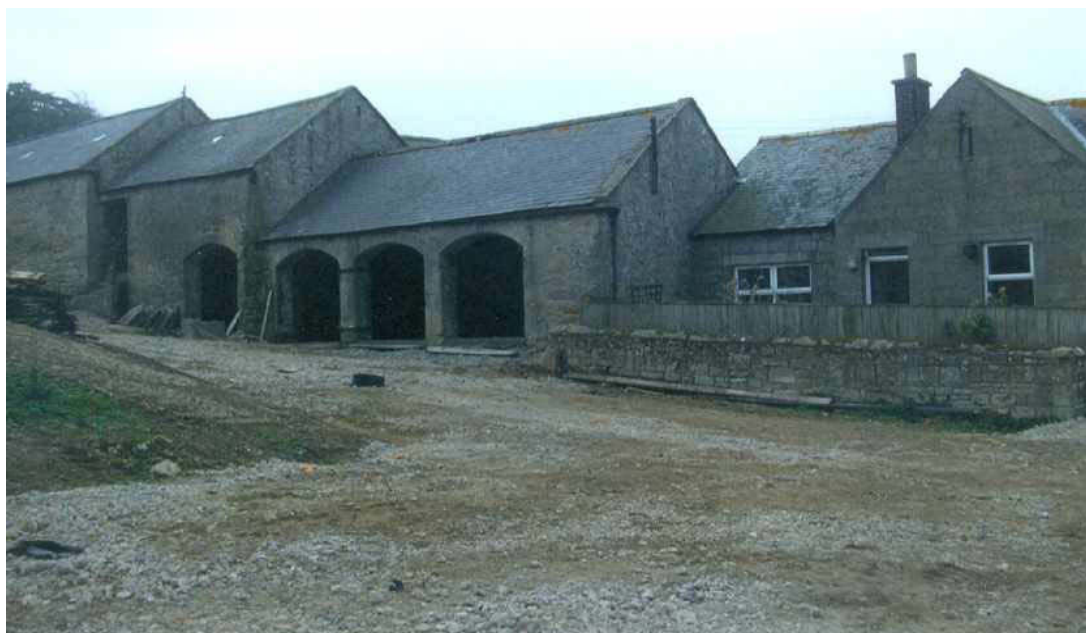
Plate 6: Rooms B, C and D, facing south-west
