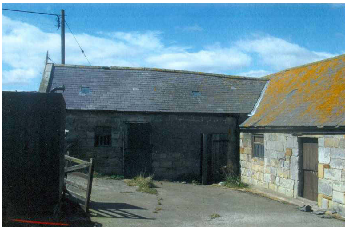
Plate 2: Rooms E and F from the south-east
