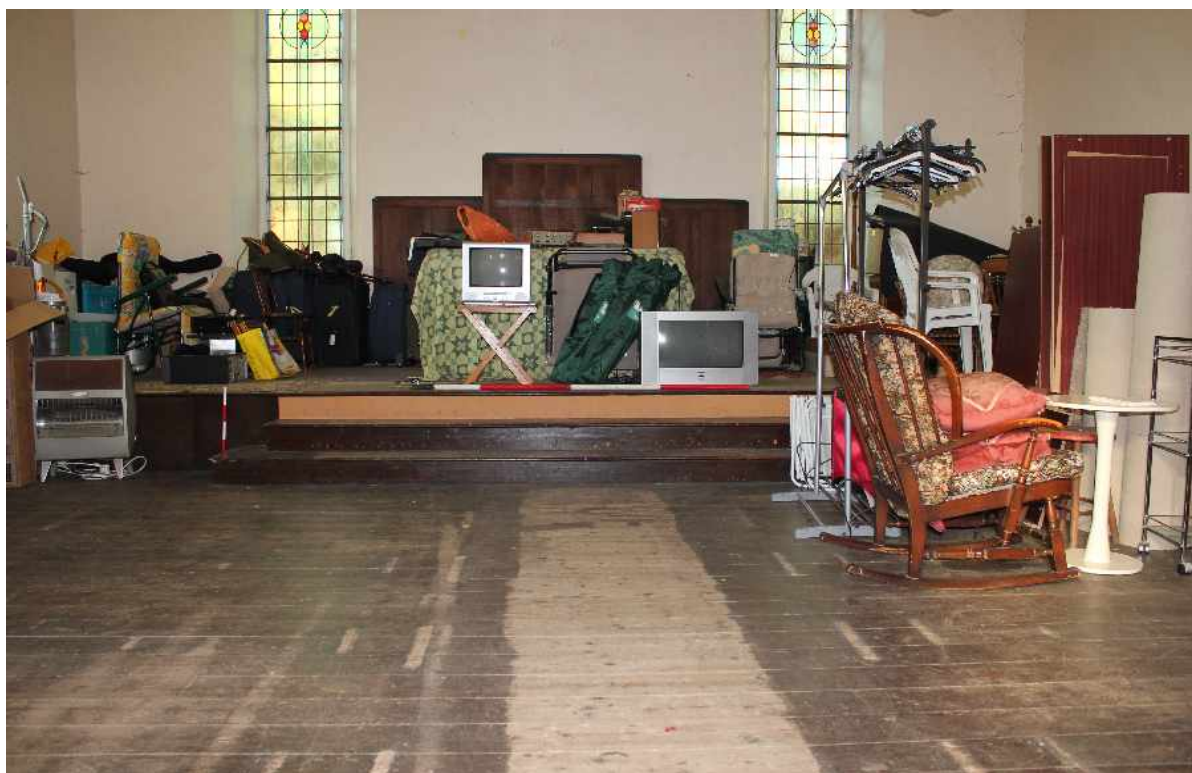
Plate 7: Internal view of north wall, showing dais end of the hall and the timber panelling
