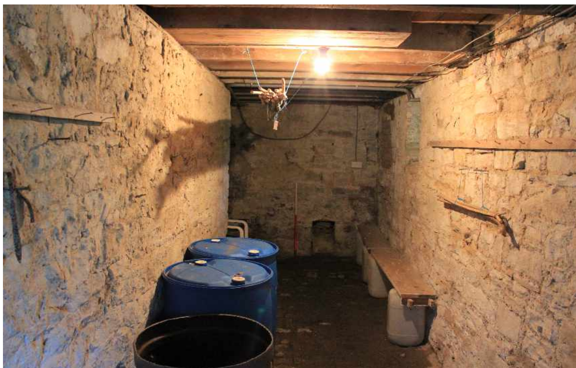
Plate 4: Internal view of the small cellar, facing east
