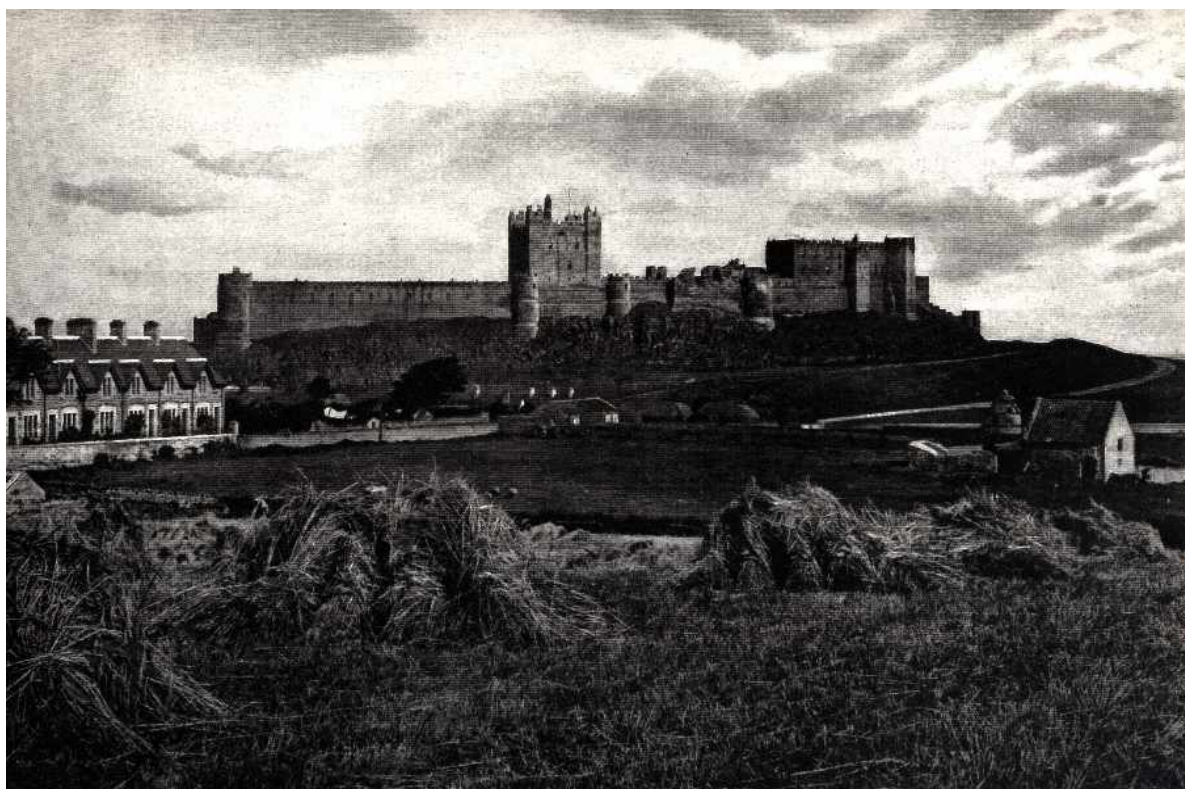
Plate 1: View of the putative hospital site, facing east
