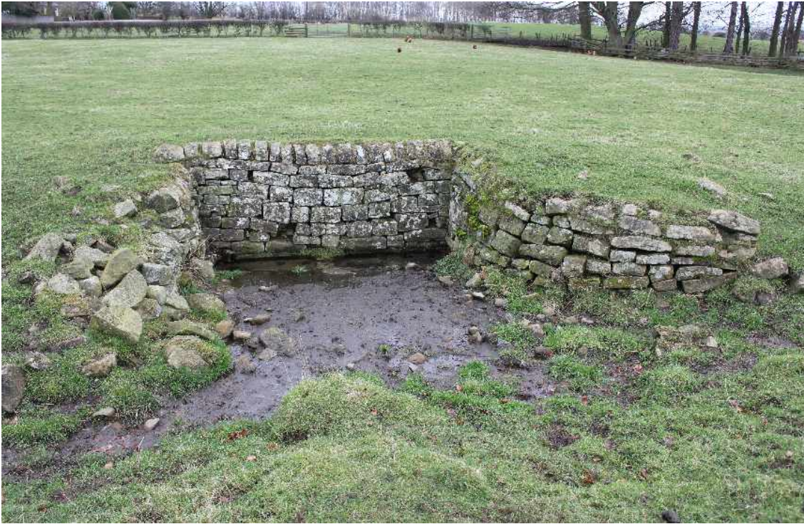
Plate 5: View of the dry stone spring trough in the upper western field facing east
