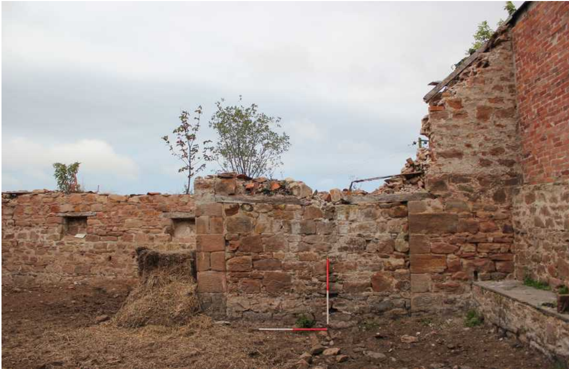
Plate 5: Blocked entrance in stub wall at the rear of Courtyard B, facing north
