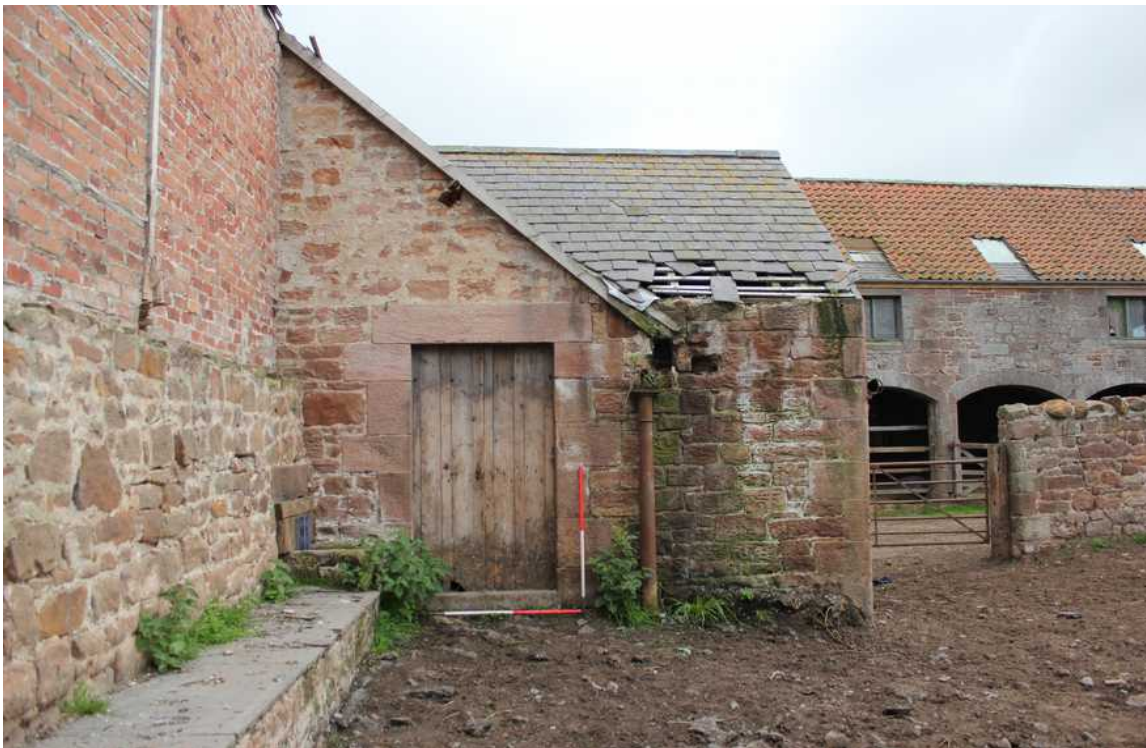
Plate 4: Rear, north side, of Building A, from within Courtyard B
