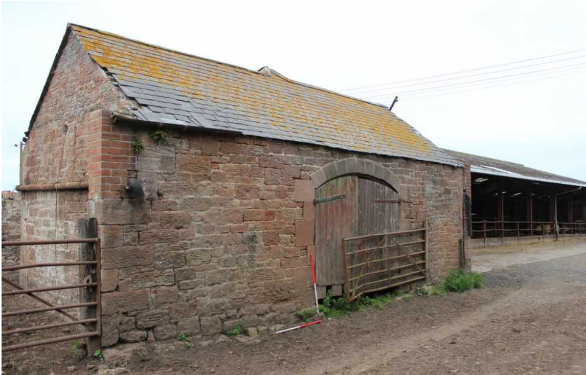
Plate 3: Building A, facing north-east, showing double door and later brick repair.
