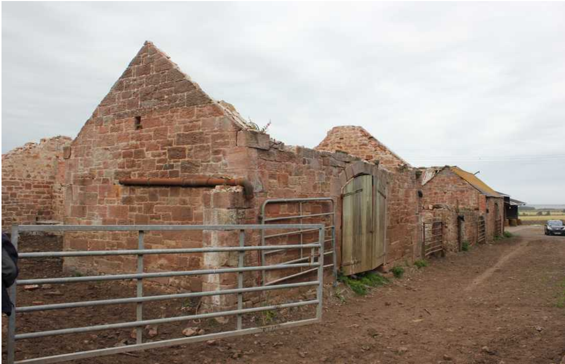
Plate 1: South side of range, facing east, north-east, Building B, foreground
