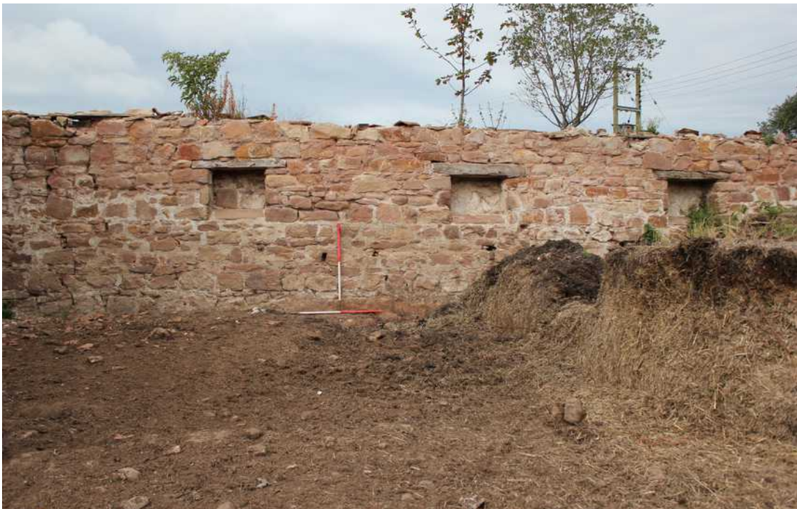
Plate 6: Blocked windows in the south facing wall of Courtyard B
