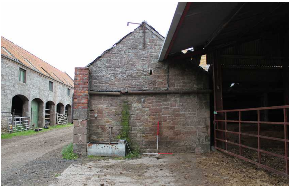
Plate 2: East side of Building A, listed building's in the background
