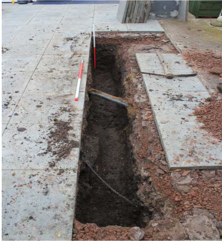
Plate 1: Main construction trench, facing south
