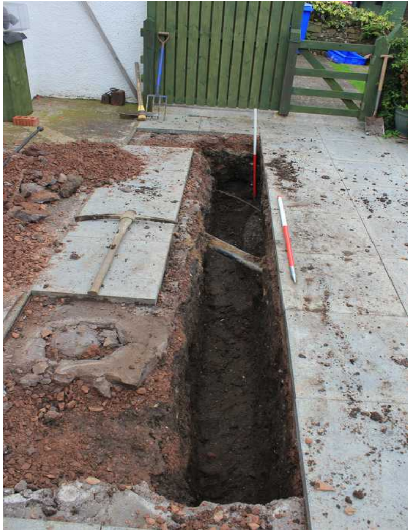
Plate 2: Main construction trench, facing north
