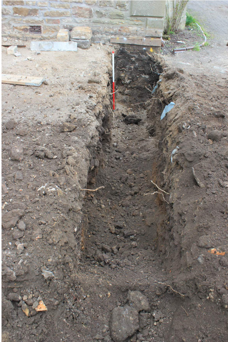
Plate 2: Orangery construction trench, facing north east
