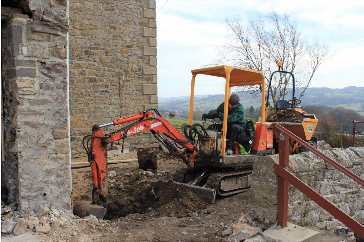
Frame 1: Machine excavation of the orangery foundation, facing east
