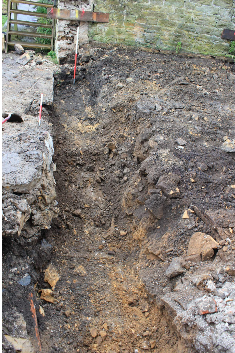
Frame 3: Southern boot room excavation trench, facing south west
