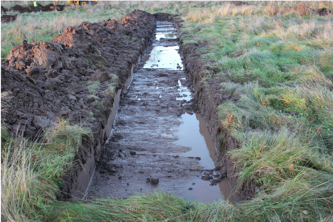
Plate 5: Trench 5, facing north
