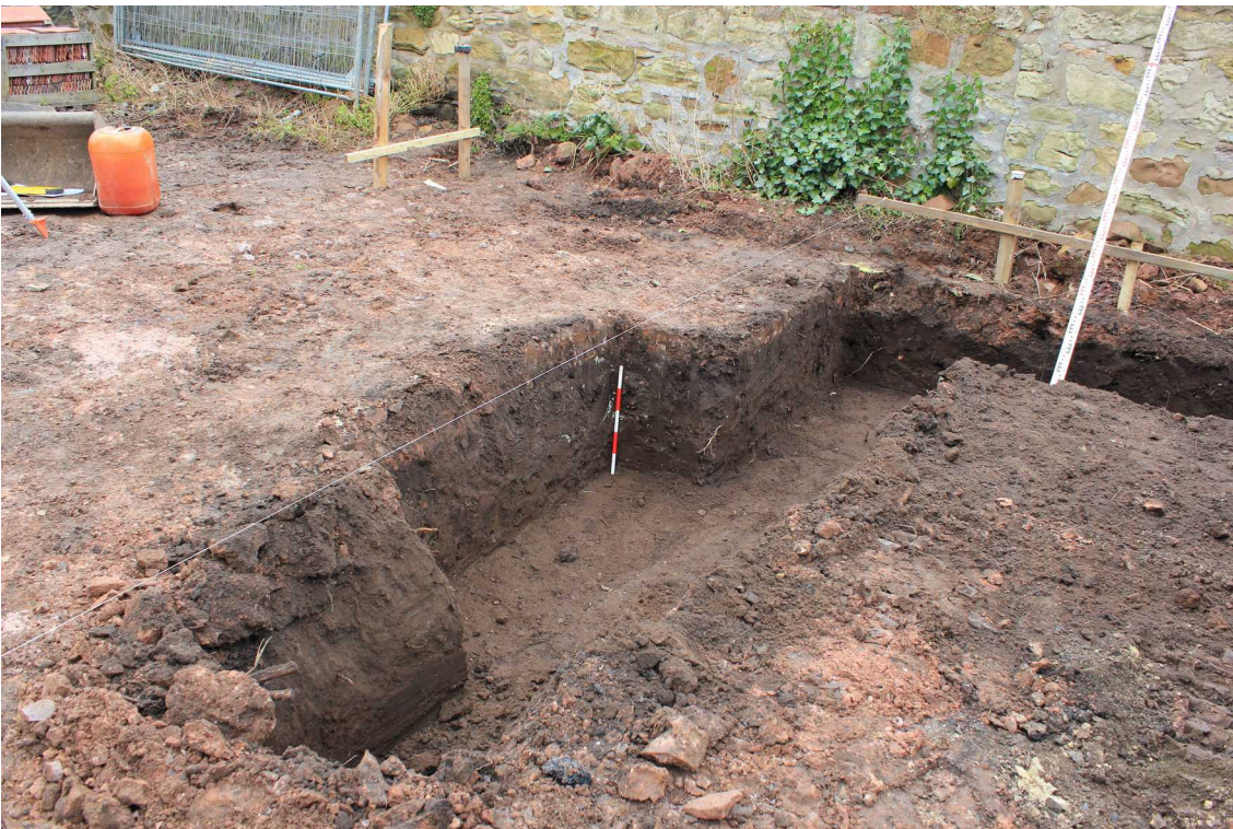
Frame 2: Annexe north construction trench, looking north-east
