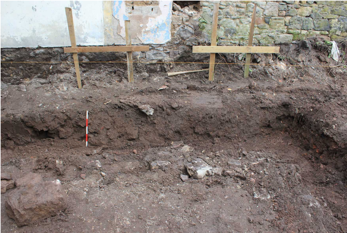
Frame 1: Building extension trench, looking east
