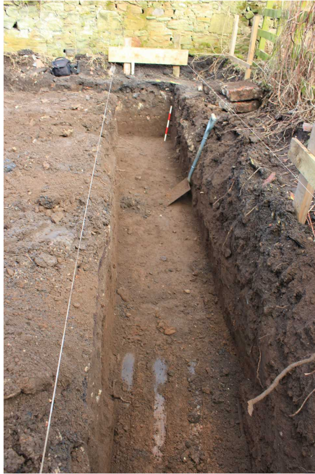
Frame 4: Annexe south construction trench, facing east
