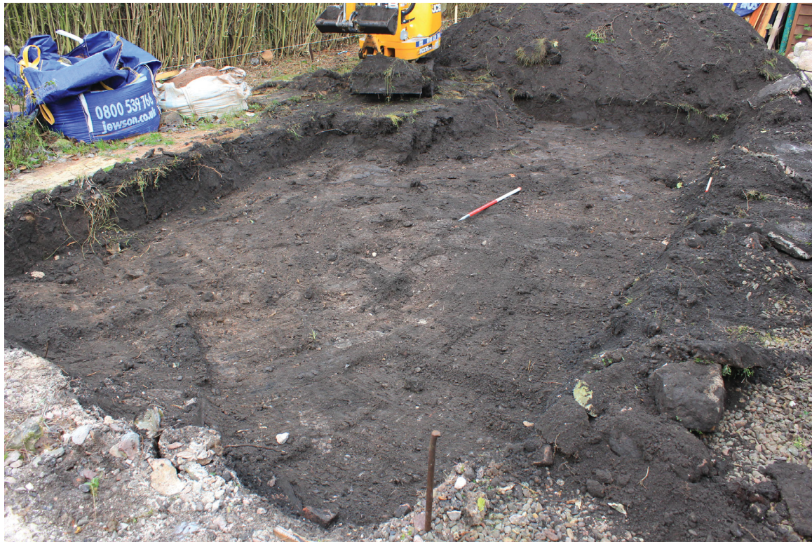
Plate 2: Excavated footprint of the new building, facing north-west
