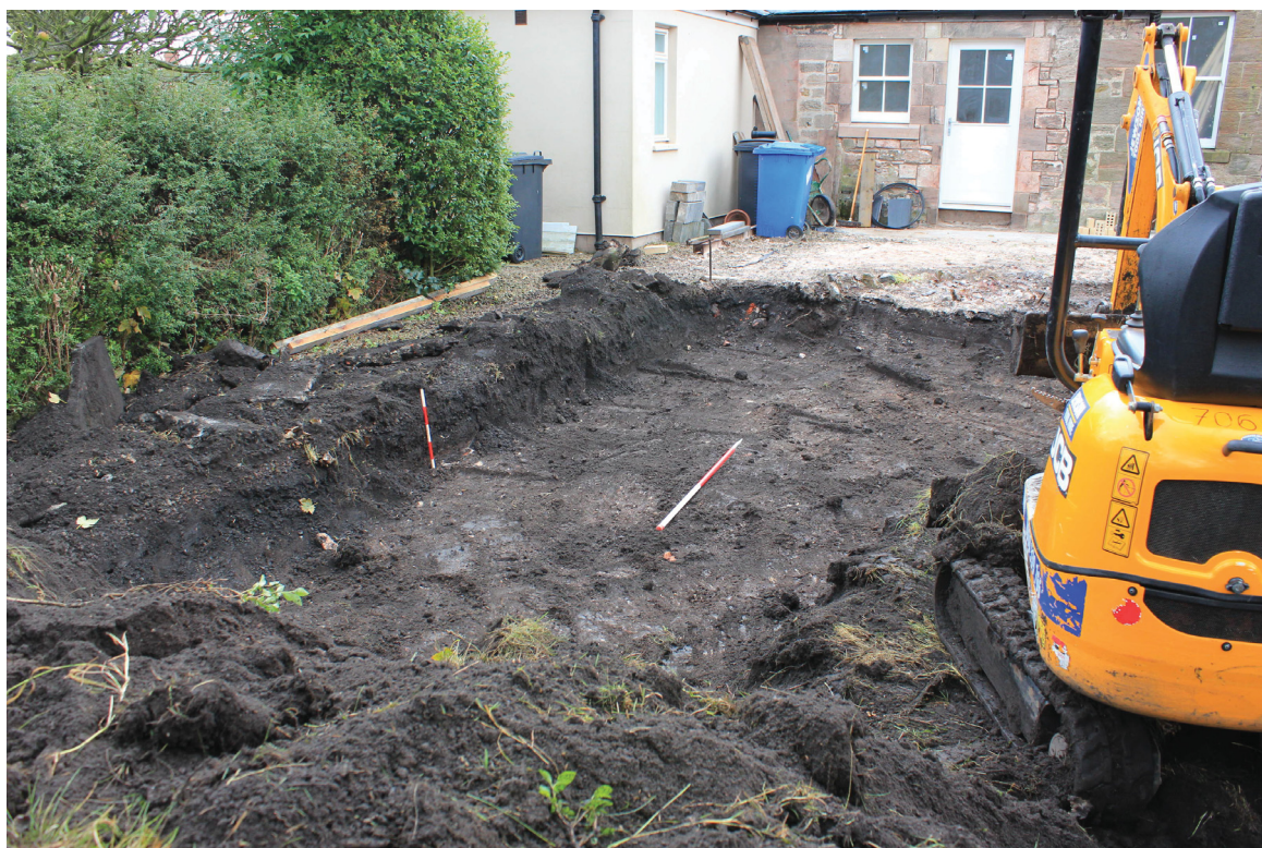
Plate 1: Excavated footprint of the new building, facing south-east
