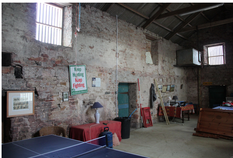
Plate 16 North wall of Room F
