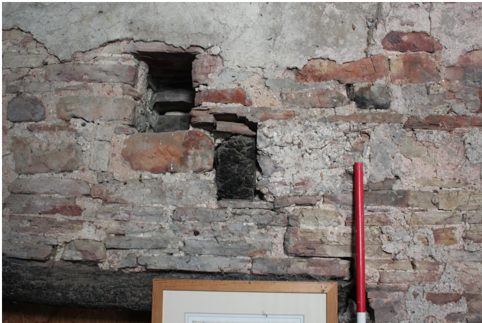
Plate 14 Wooden floor joist and niche, Room F, north wall, west end
