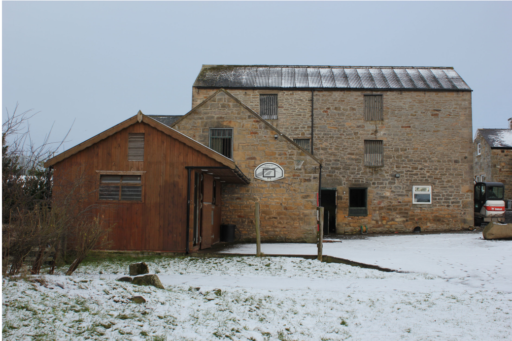
Plate 3: South elevation of the mill building
