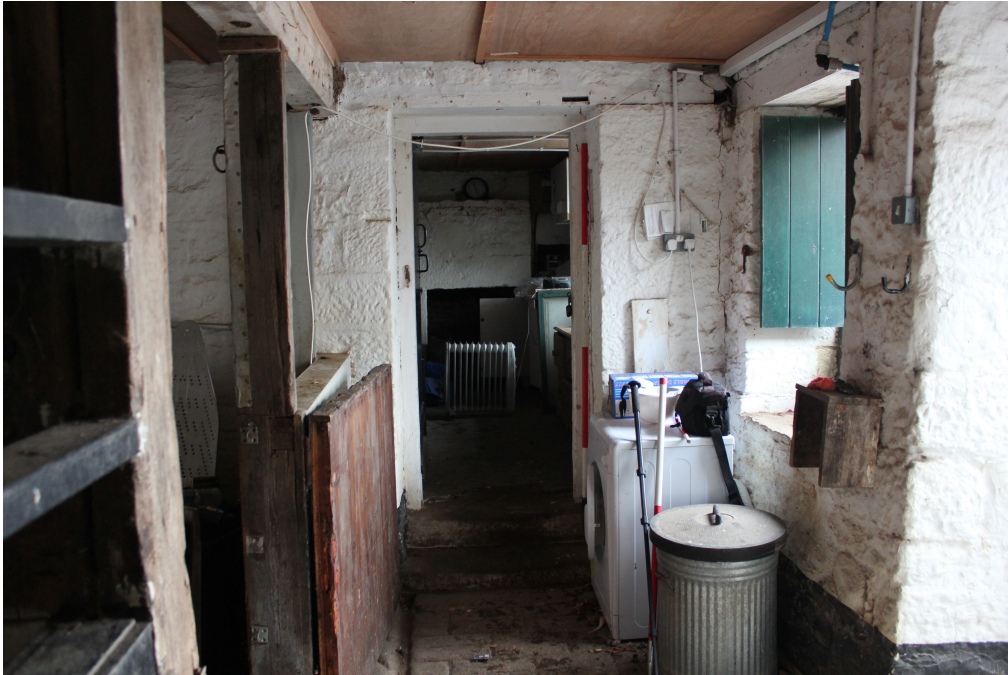
Plate 9: Doorway between Rooms A and B, facing east
