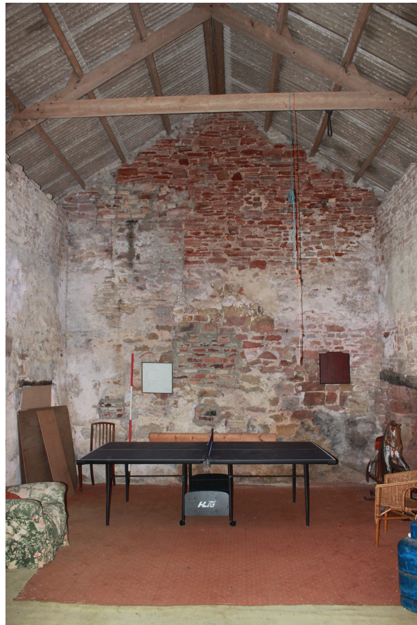
Plate 17 West wall of Room F
