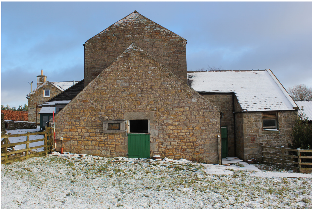
Plate 4: West elevation of the mill building
