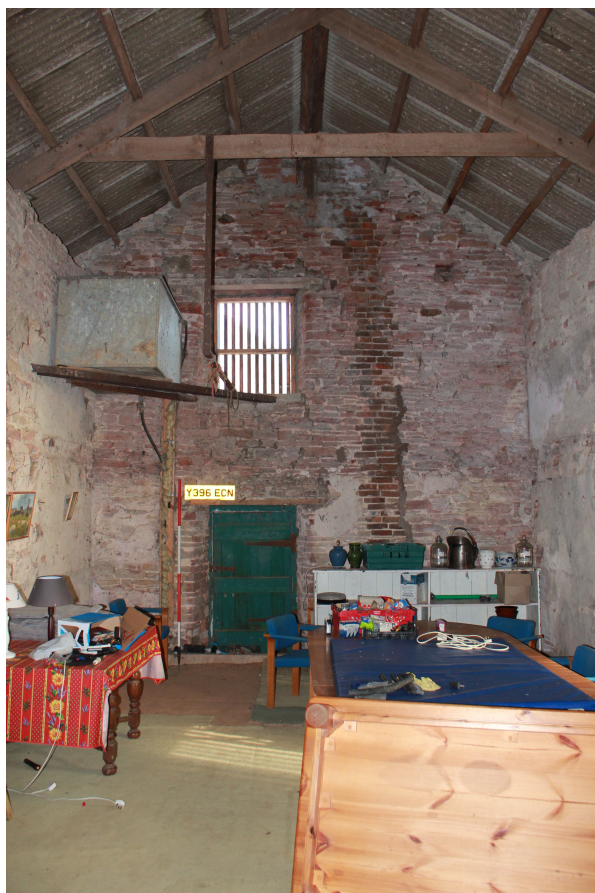
Plate 15 East wall of Room F, showing chimney patch
