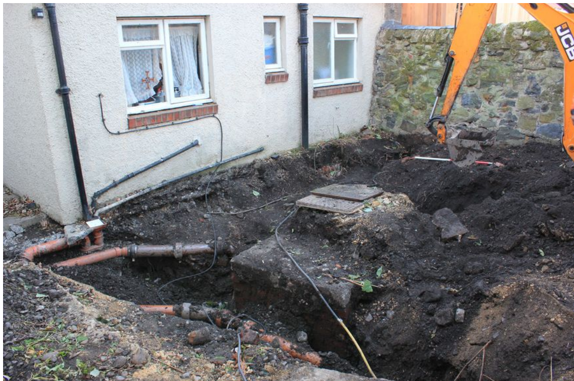
Plate 2: Excavation of the existing drain chamber and old drains, facing north-east
