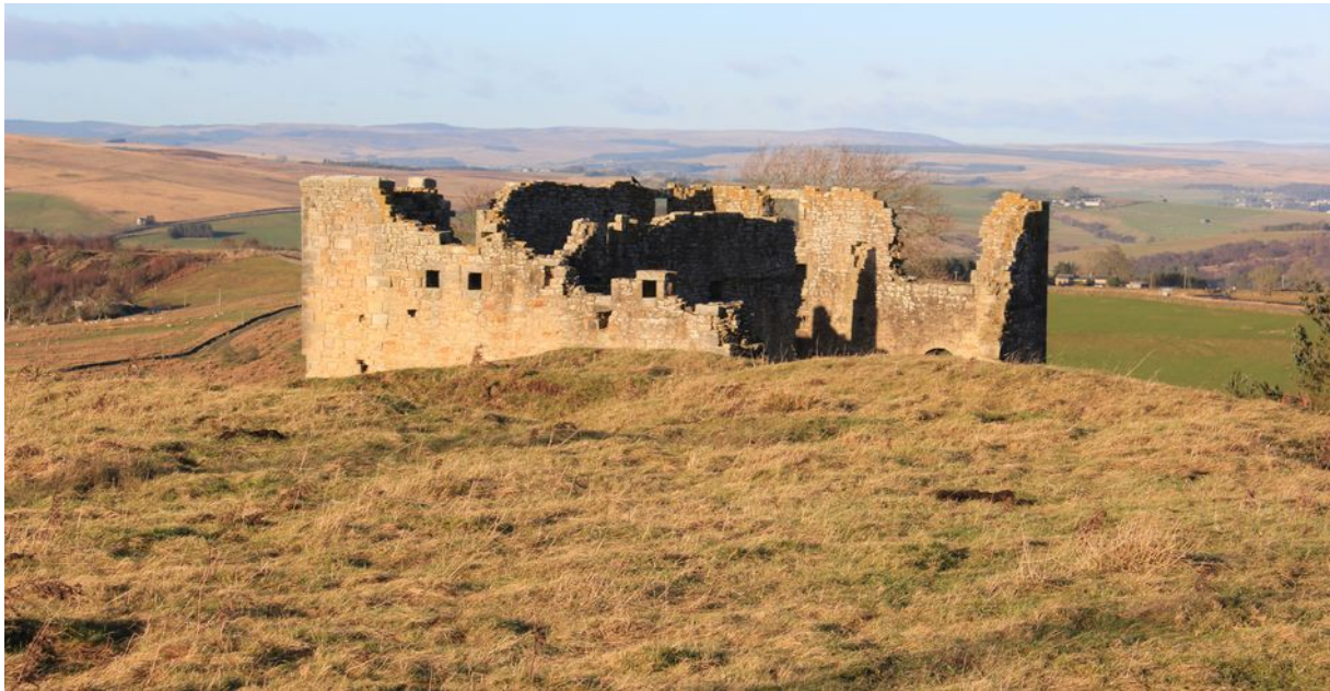
Plate 13: The Engine House at the Ridsdale Iron Works, facing north-west
