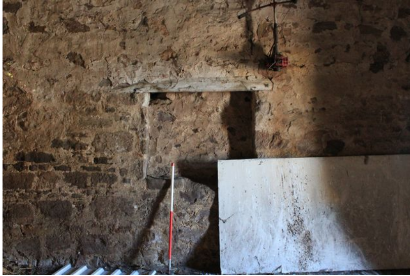
Plate 10: blocked window feature in the west wall of Room D, facing west
