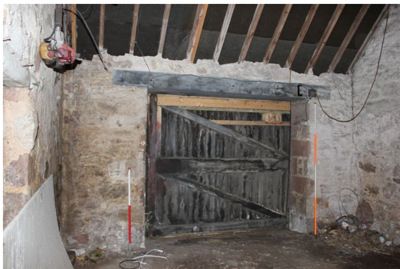
Plate 9: the double door leading from Room D, facing north
