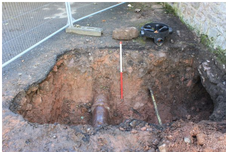
Plate 18: Trench 6 with existing sewer pipe, facing east
