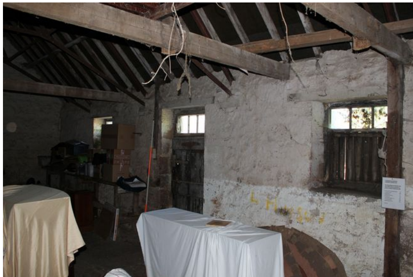
Plate 11: Room E south wall showing windows and door, facing north-west
