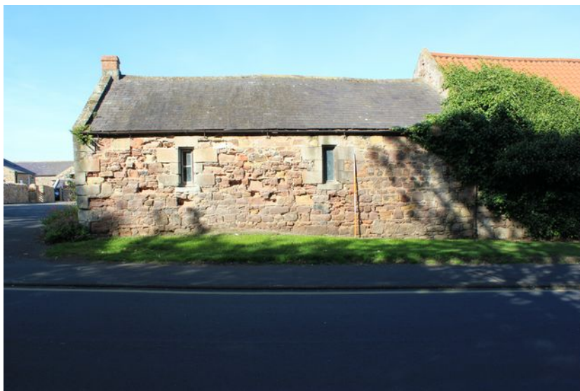
Plate 3: the western range of the buildings, facing north
