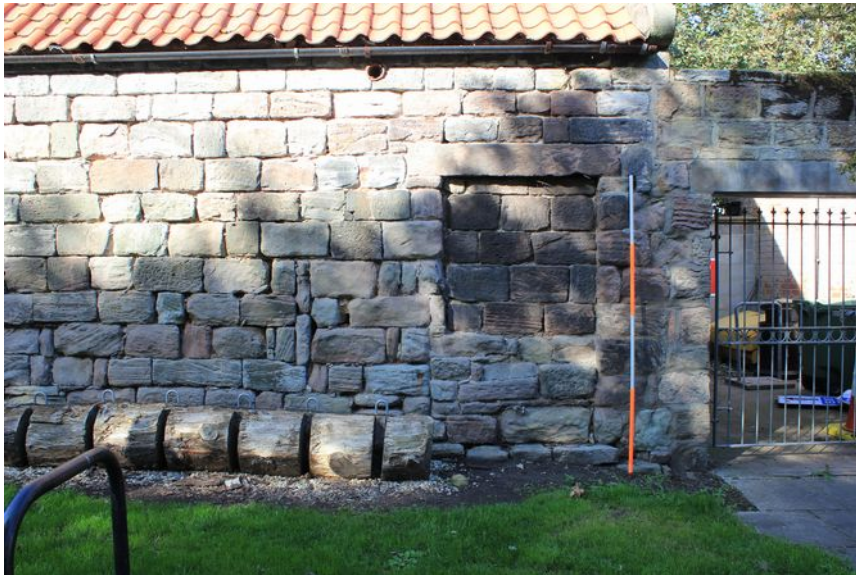
Plate 2: blocked window at the east end of the north facing exterior wall
