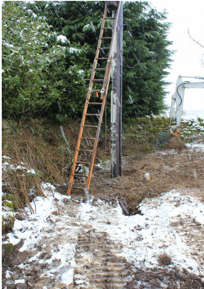
Plate 4: Electric pole installed, facing south
