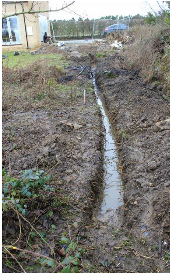
Plate 1: Service trench fully excavated, facing north
