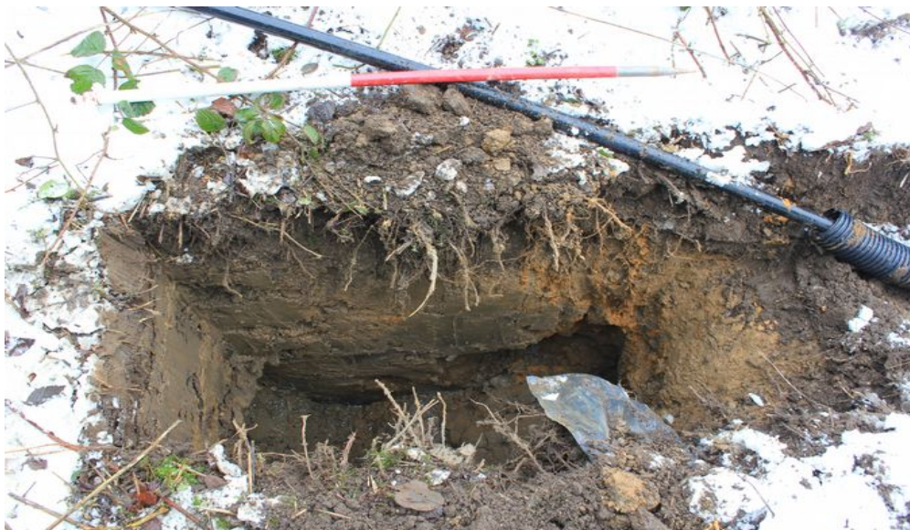
Plate 3: Trench for electric pole, facing west
