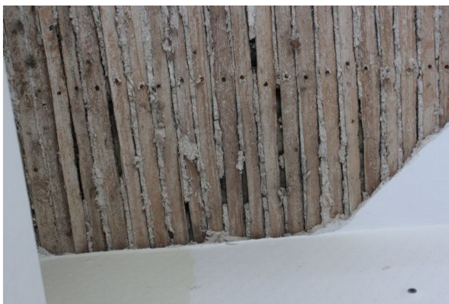
Plate 7: Earlier laths and plaster seen beneath the modern plaster board, hall ceiling first floor, facing west
