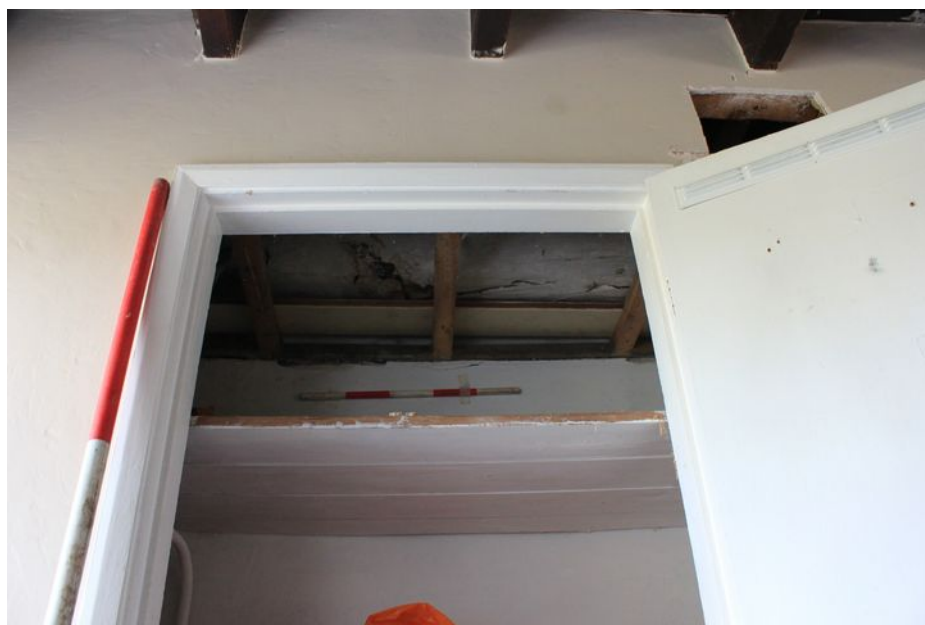
Plate 4: The old timber beam revealed above the plasterboard false ceiling within the cupboard, facing south
