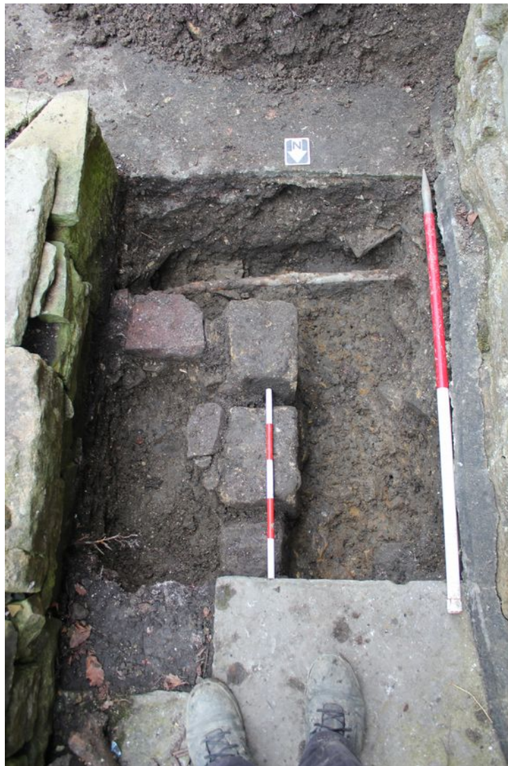
Plate 14: Trench 6 showing the stub wall (602), facing south
