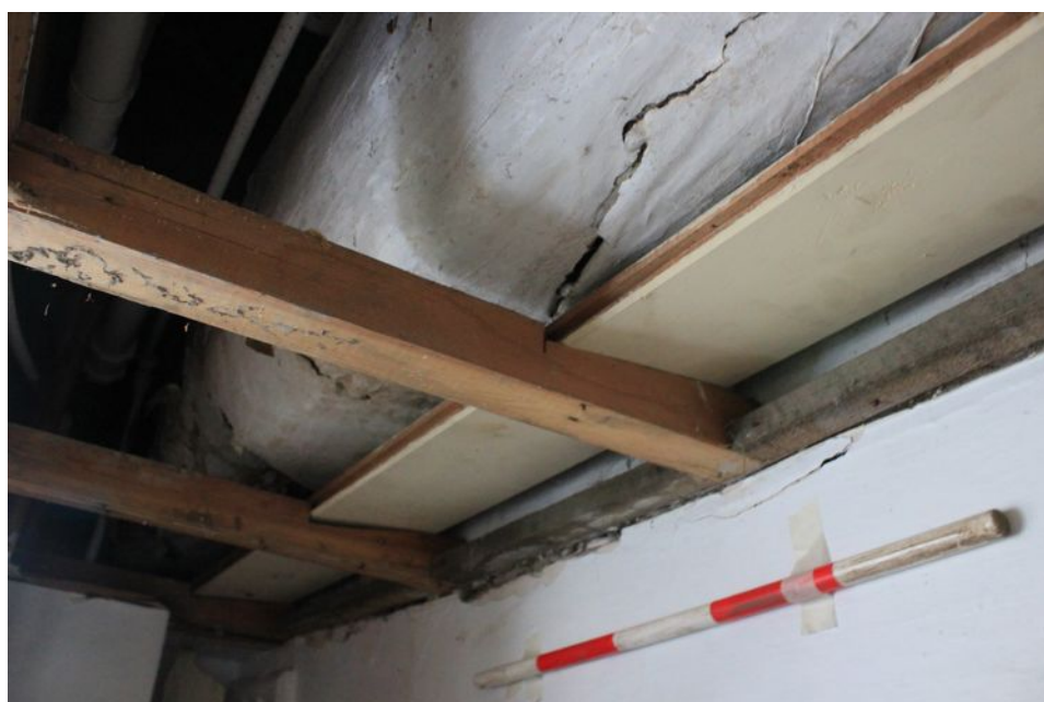
Plate 4: The old timber beam revealed above the plasterboard false ceiling within the cupboard, facing south
