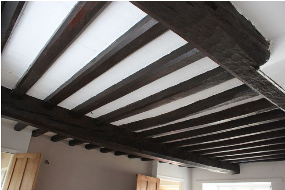
Plate 1: Ceiling structure of Room B, looking south-west
