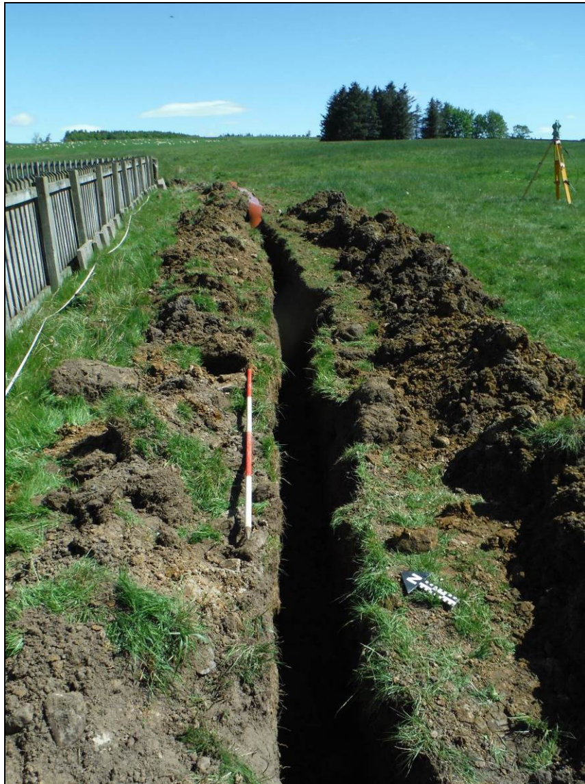
Figure 10. Overview of the trench, facing north-west (scale = 2m).
