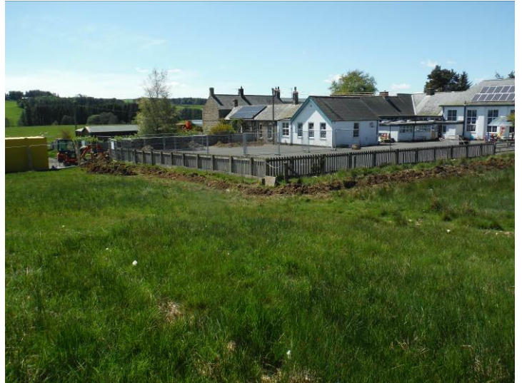
View facing south Otterburn First School.
