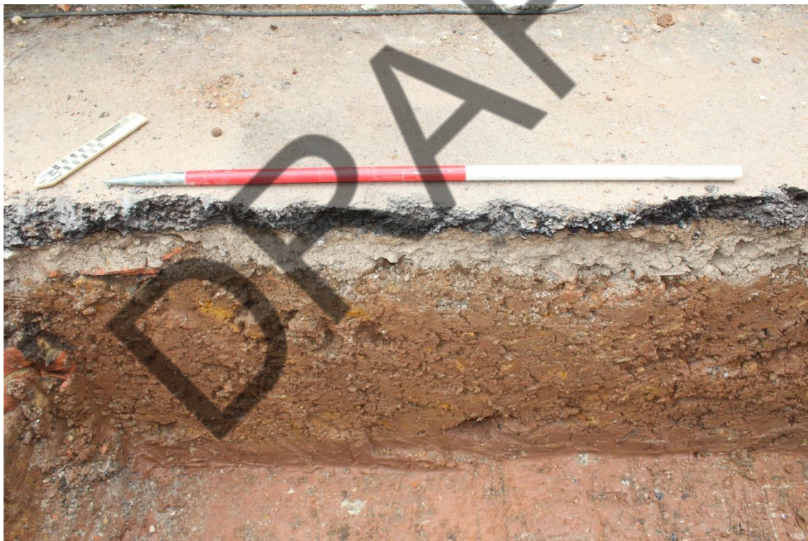
Figure 3: Shot of Representative Section Showing Tarmac (05), Hardcore (02) and Natural Geology (07) and (08)
