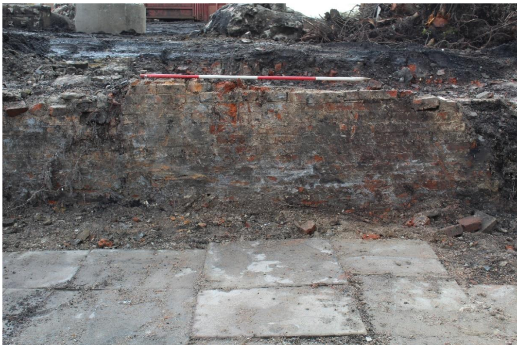
Figure 20. Photograph of 19th century wall {2035}, looking south (scale: 1x2m)
