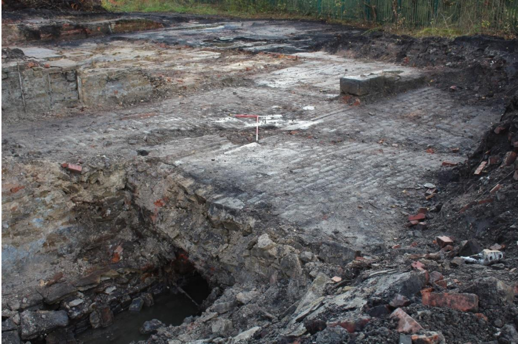
Figure 18. Overview of Area 2, looking south-west with culvert {2064} beneath surface (2055) in foreground and walls {2035}/{2042}/{2043} in background (scale: 1x1m, 1x2m)
