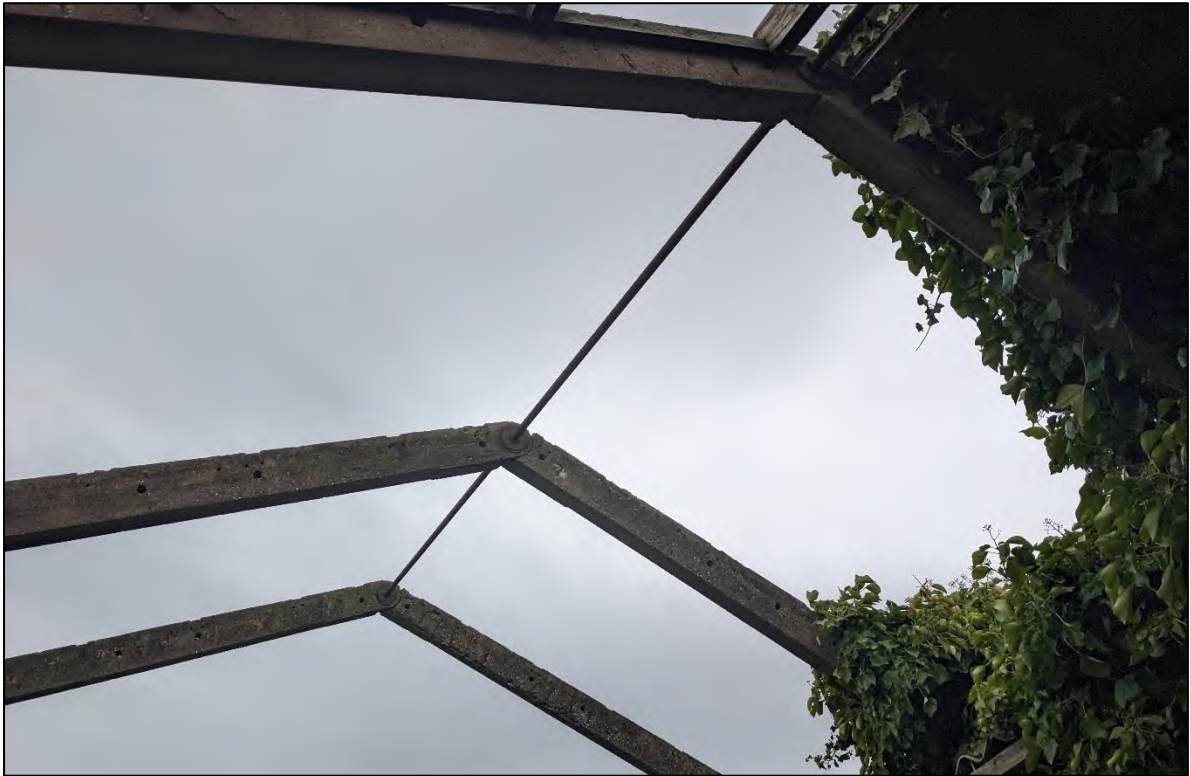
Photograph 11: View of the cast iron ridge beam within Building 1, taken facing north-west (File: HBR_168)
