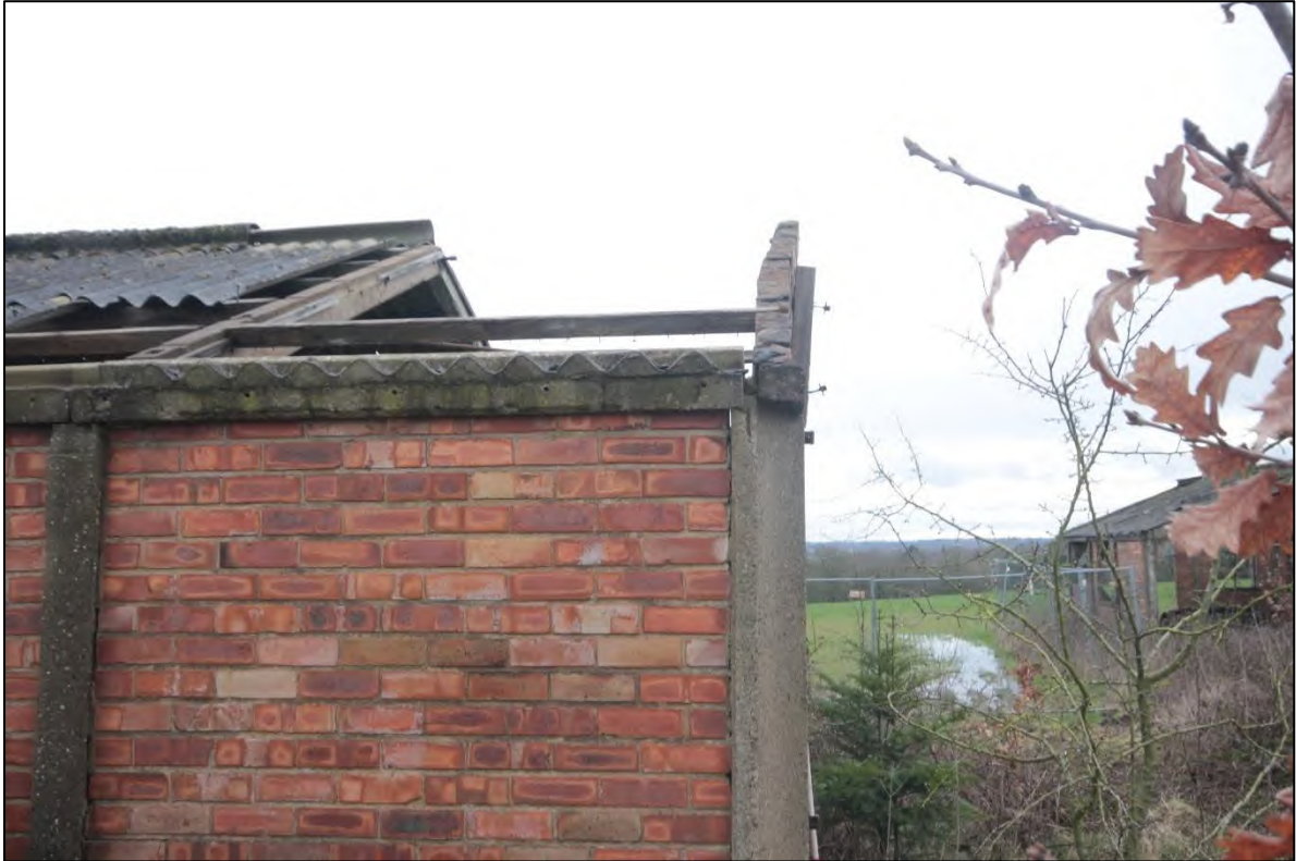
Photograph 45: View of the upper portions of Building 4's elevation leaning westwards, taken facing south (File: HBR_116)
