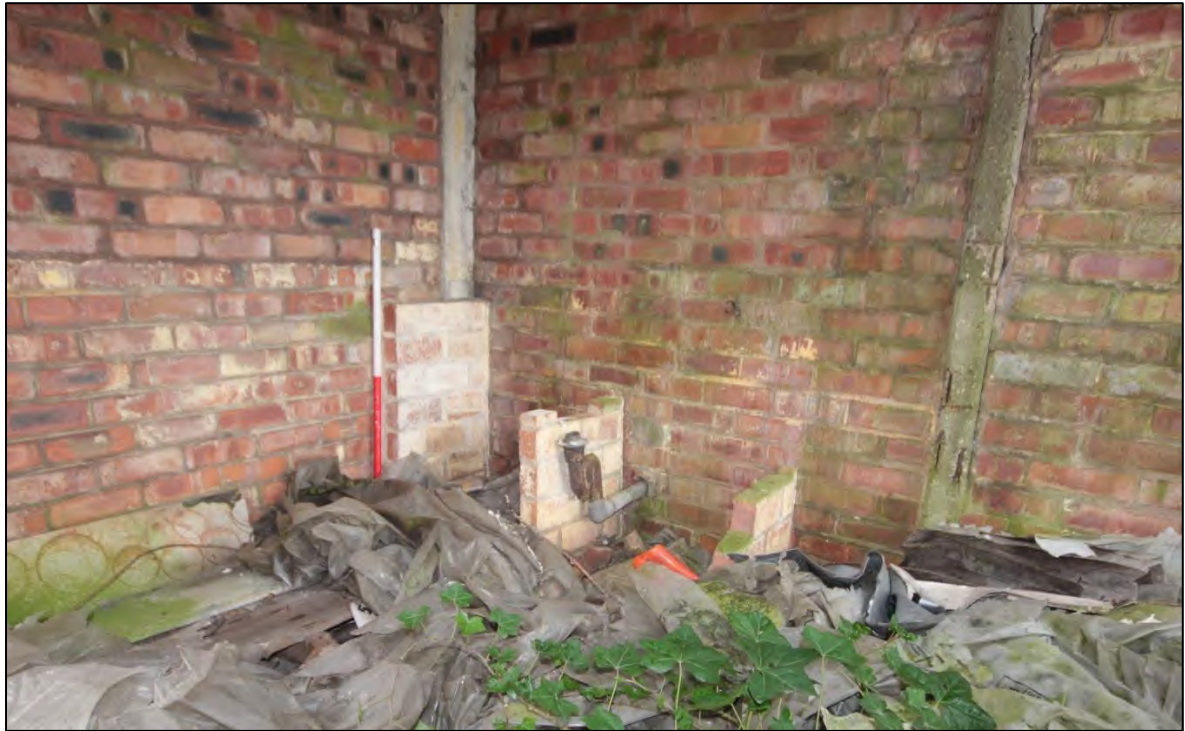
Photograph 26: The brick feature for a sink within the north-eastern corner of Building 1's interior, taken with 1m scale (File: HBR_53)
