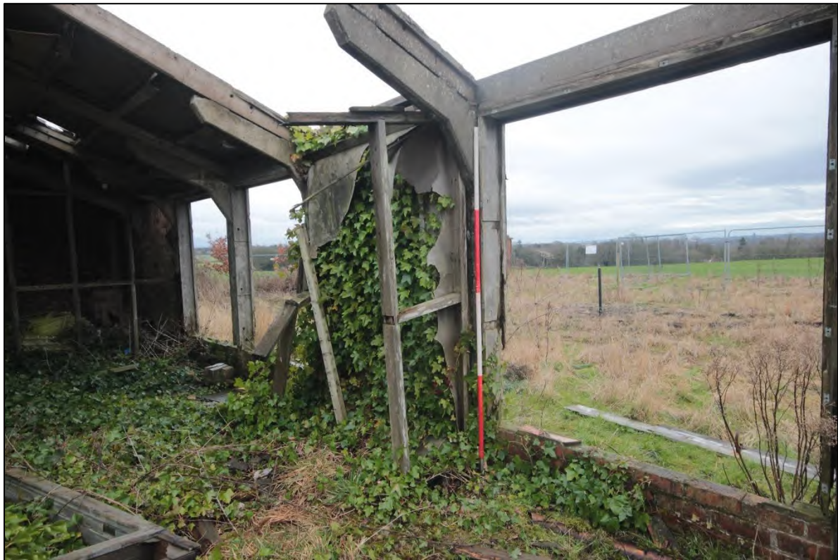
Photograph 24: View of the stud walling within the central extent of Building 1's southern wall, taken facing south-east with 2m scale (File: HBR_49)
