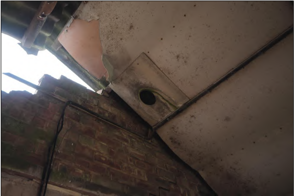
Photograph 22: The circular aperture associated with the flue within the eastern extent of Building 1's roof structure (File: HBR_164)
