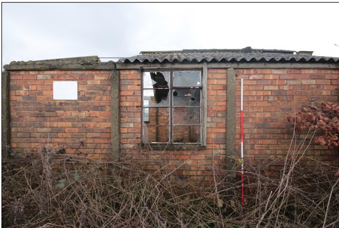
Photograph 13: View of a cast iron window casement associated with Building 2's eastern elevation, taken facing west with 2m scale (File: HBR_71)
