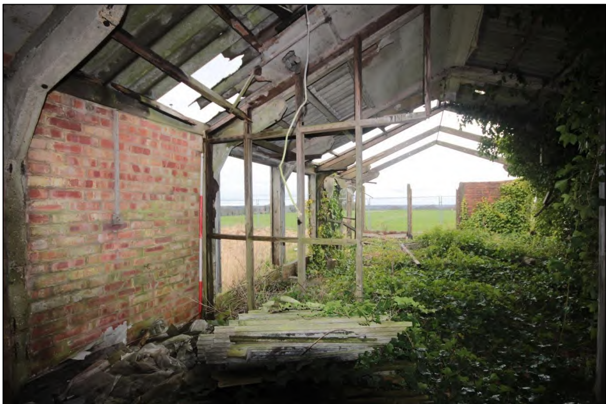
Photograph 25: View of the stud walling within the eastern extent of Building 1's southern wall, taken with 2m scale facing west (File: HBR_54)
