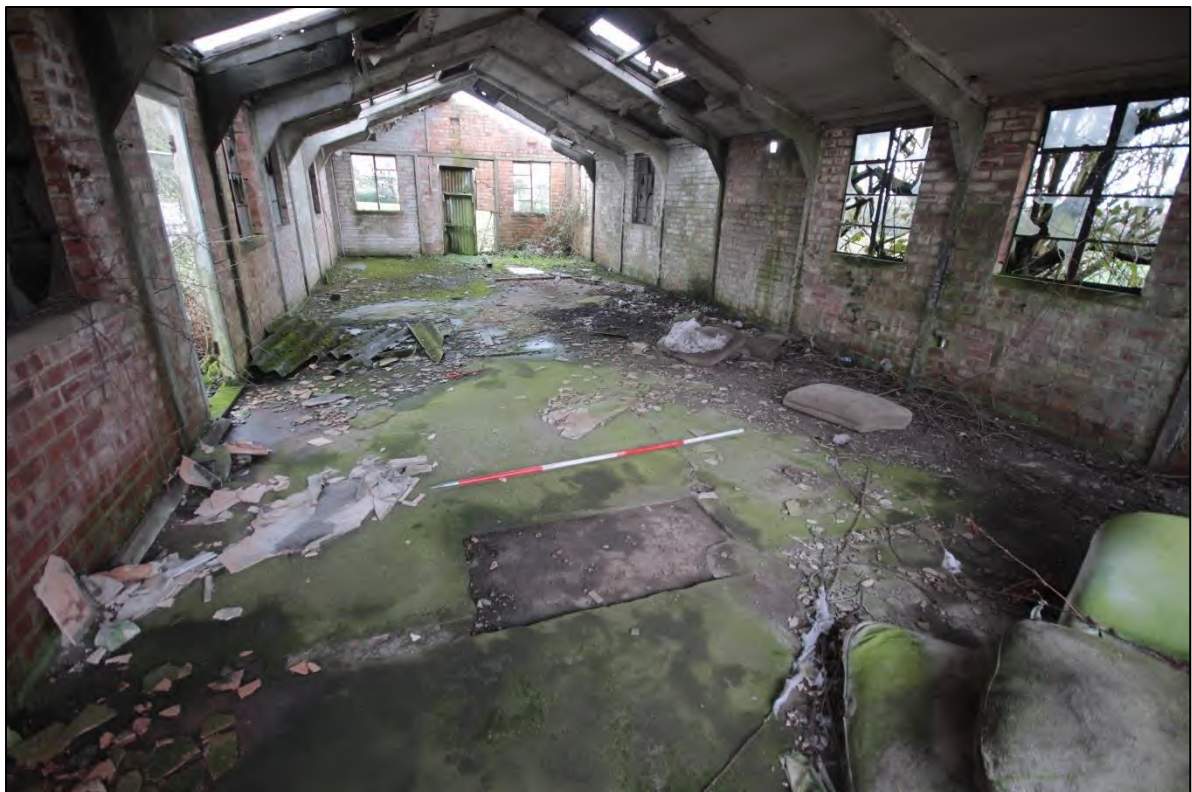
Photograph 61: View of Building 5's concrete flooring, with a straight joint delineating a former partition wall, and rectangular outline likely associated with an earlier heating source. Taken facing south-east with 2m scale (File: HBR_143)
