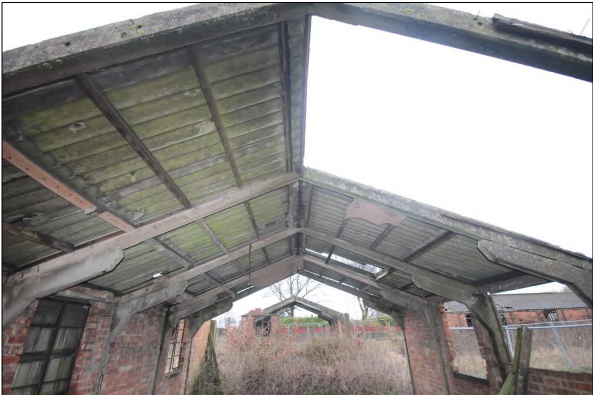
Photograph 10: View of the concrete framed roof structure within Building 3, taken facing north (File: HBR_103)
