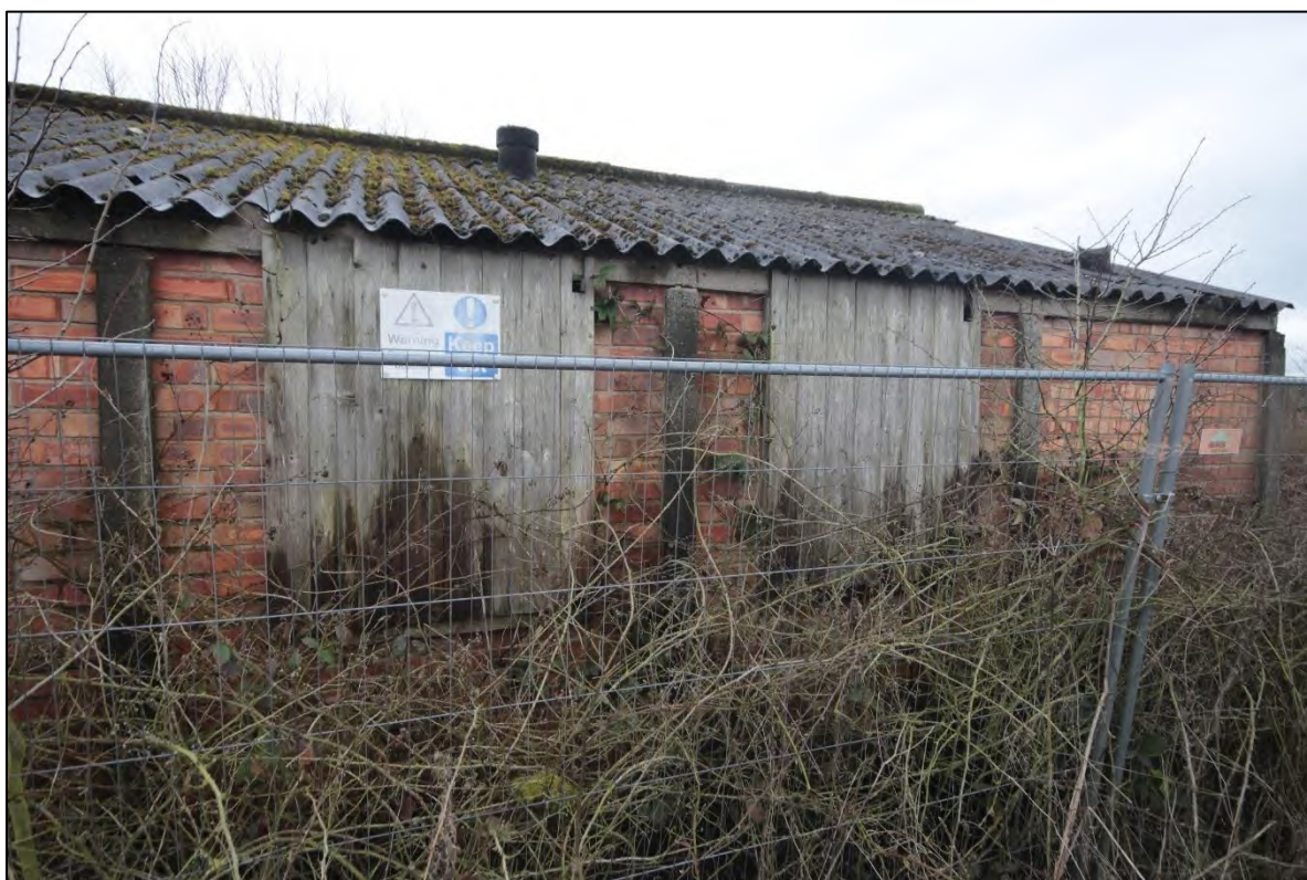
Photograph 14: View of the timber window shutters associated with Building 5's northern elevation, taken facing south-west (File: HBR_139)
