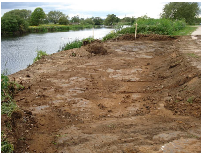
Figure 4: View of the stripped eastern bank showing the subsoil (005).
