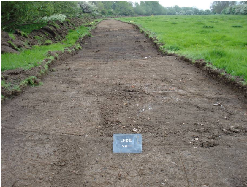
Figure 3: View of the stripped temporary haul route. The dark band shows the location of the debris deposit (003).
