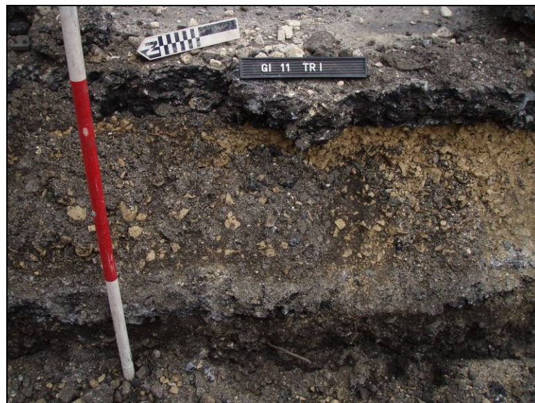
Figure 4: North facing section of Trench 1 showing two levels of hardcore and tarmac.
