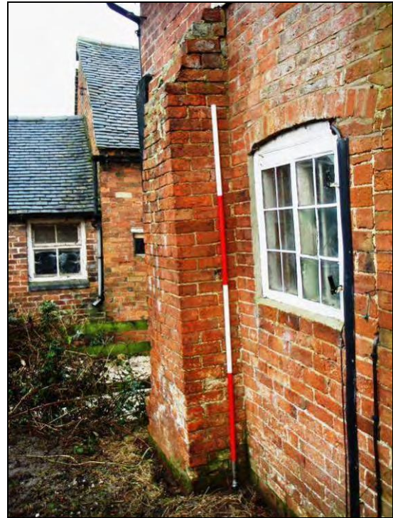
Figure 8: Detail of the chimney and inserted window (scale 2m)
