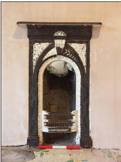
Figure 63: Detail of cast-iron fire grate (scale 300mm)
