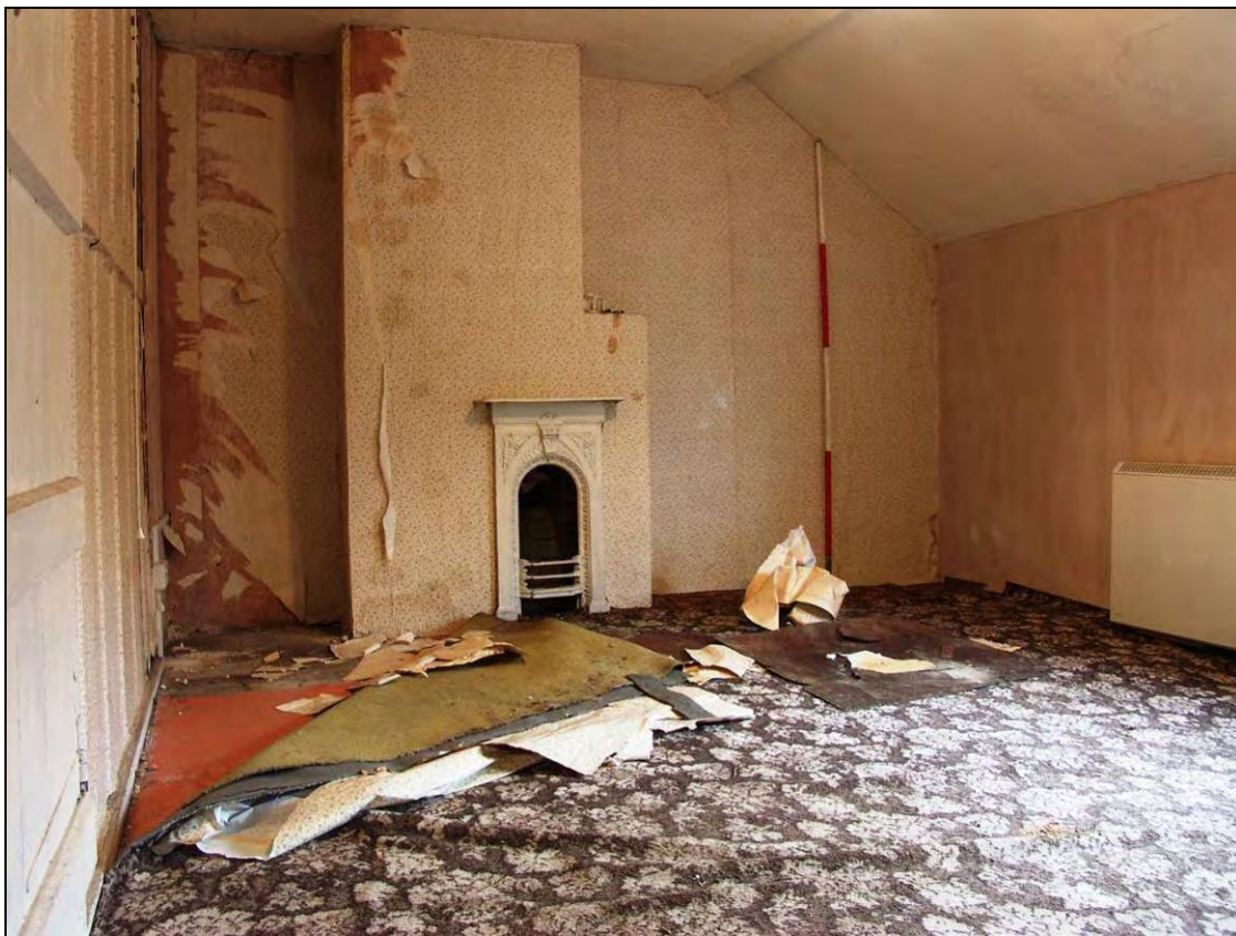
Figure 56: Room F-2 with central cast-iron fire grate, looking south (scale 2m)
