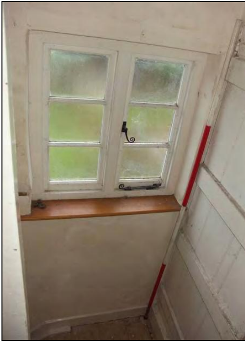
Figure 48: Window on the landing (scale 2m)
