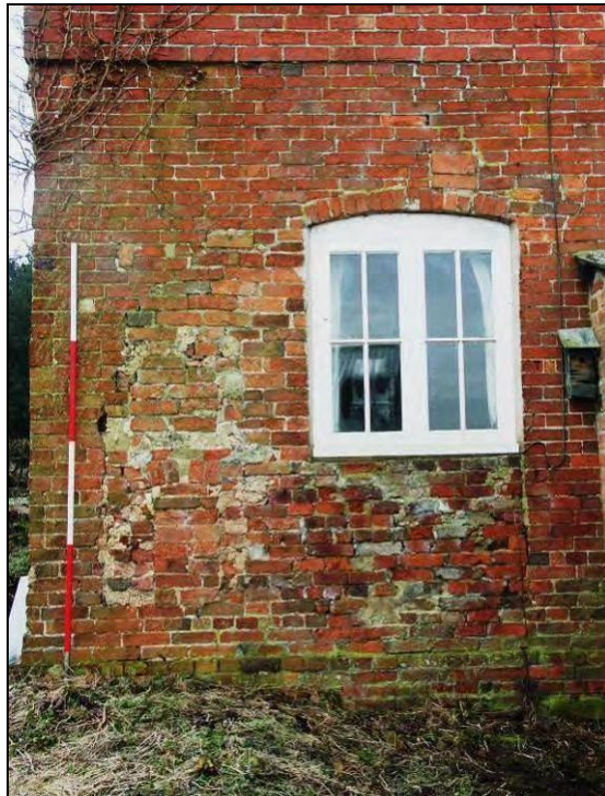
Figure 14: Southern bay with bricked-up oven
