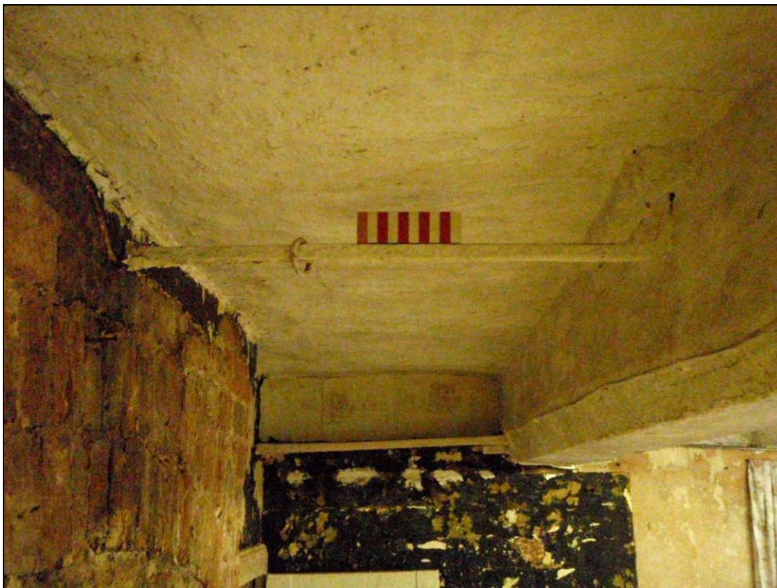
Figure 38: Iron rod with ring over the arched head of a former kitchen range (scale 100mm)
