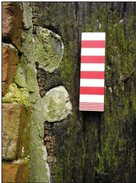
Figure 5: Detail of removed pegs (scale 100mm)
