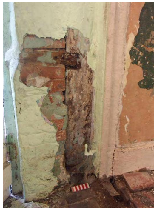
Figure 28: Inclined S-E post in room G-2
