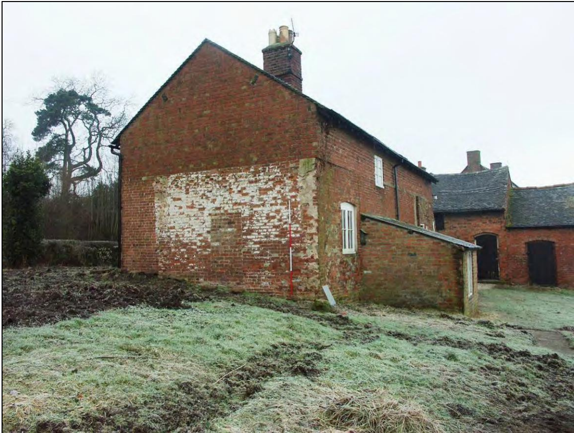
Figure 19: General view of the south elevation (scale 2m)
