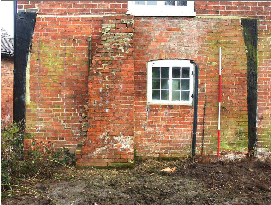
Figure 4: Northern bay with the remains of a timber-framed building (scale 2m)
