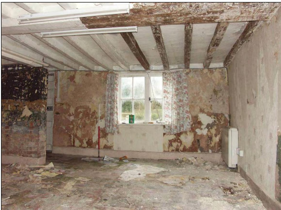
Figure 35: Room G-3, looking west (scale 1m)
