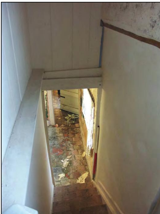
Figure 46: Staircase with timber wall plate (scale 1m)
