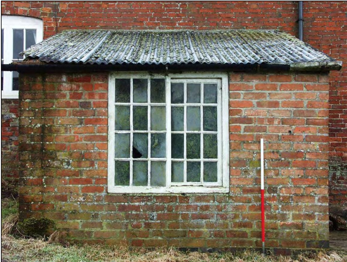
Figure 16: Lean-to extension with salvaged horizontal sliding sash window (scale 1m)
