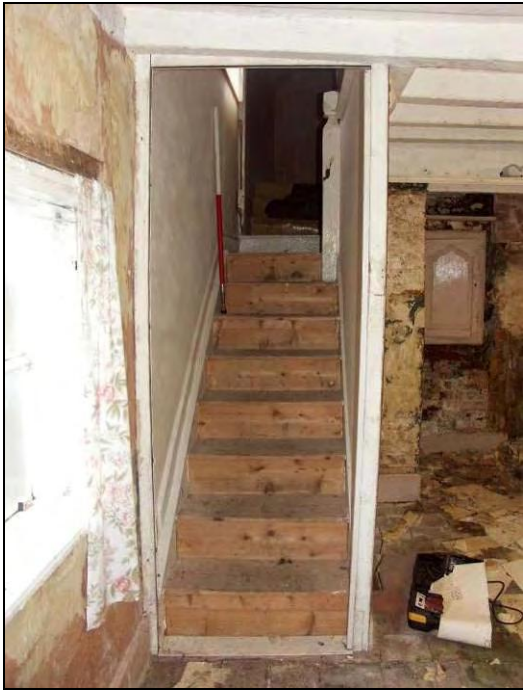
Figure 41: Staircase to the upper floor (scale 1m)
