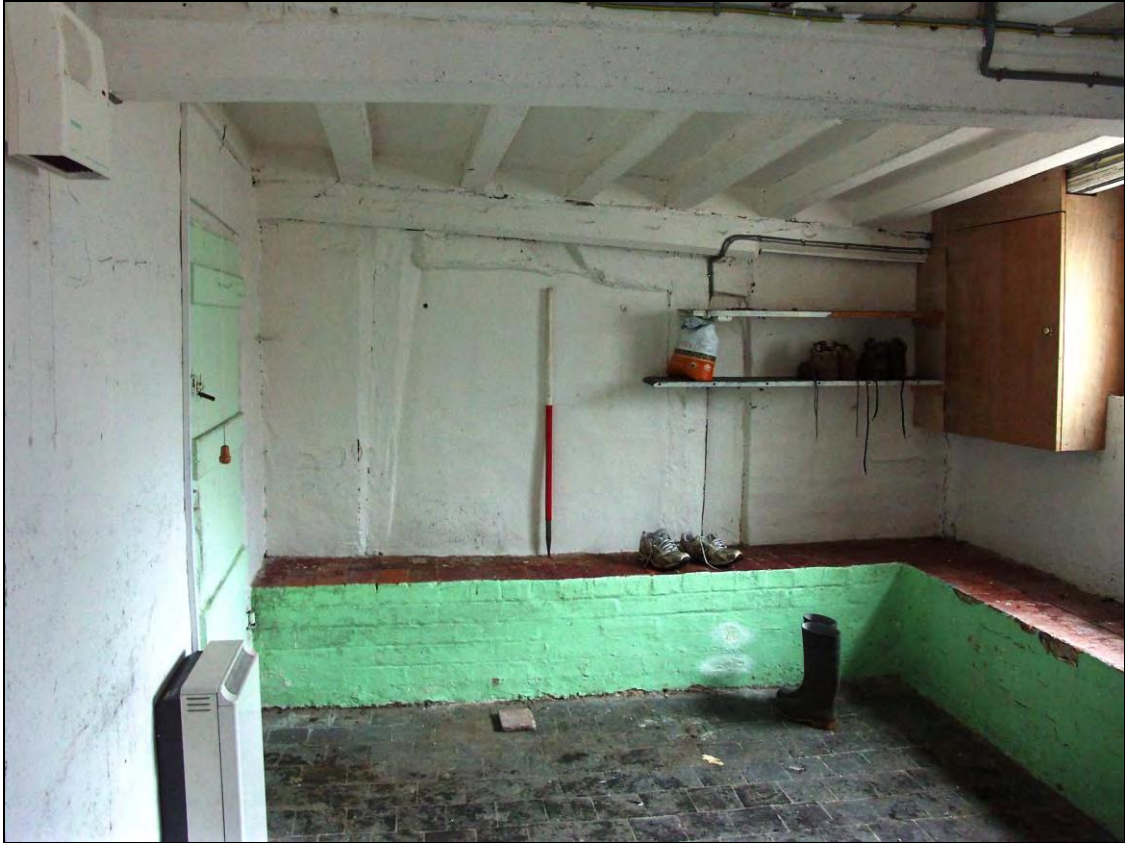
Figure 29: Surviving timber frame on the south wall of room G-2 (scale 1m)
