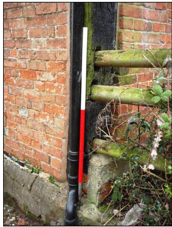
Figure 6: Slots in northern post for the present fence
