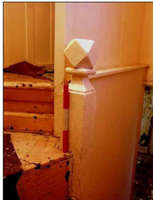
Figure 47: Detail of newel post (scale 300mm)
