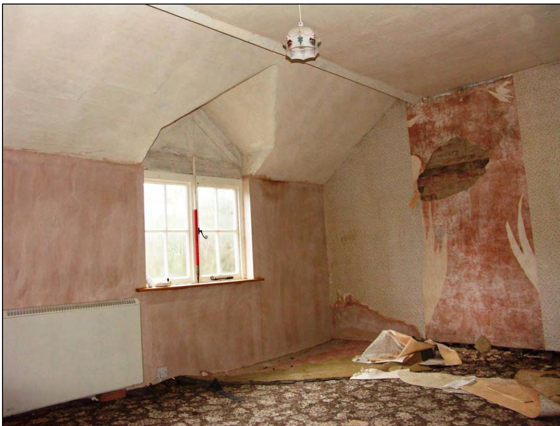
Figure 57: Western wall with repaired plaster work (scale 1m)
