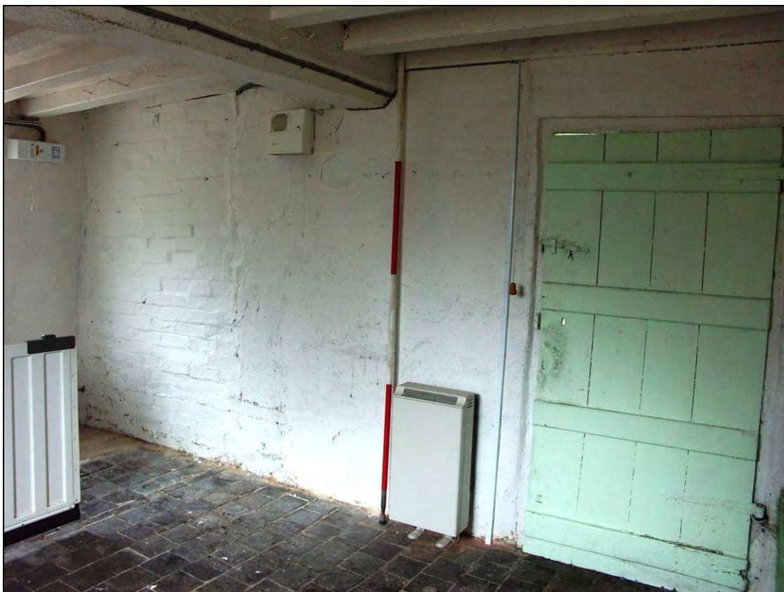
Figure 31: Doorway of room G-2 (scale 2m)
