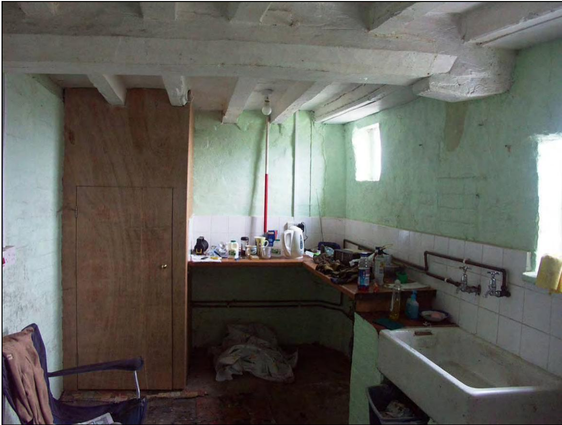
Figure 24: Southern wall of room G-1 (scale 1m)
