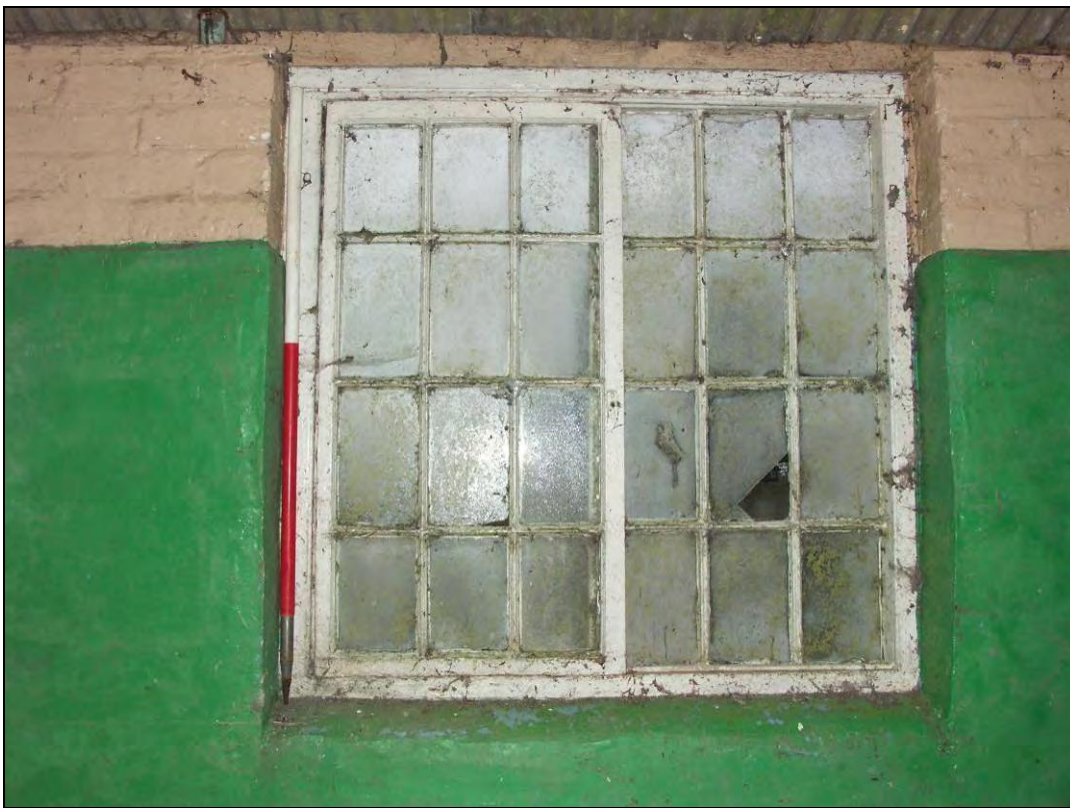
Figure 45: Detail of horizontal sliding sash window in room G-5, looking east (scale 1m)
