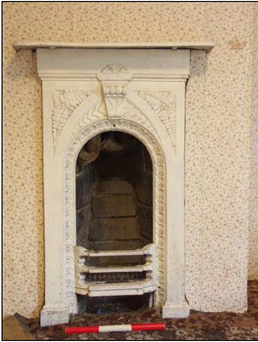
Figure 58: Detail of cast-iron fire grate (scale 300mm)
