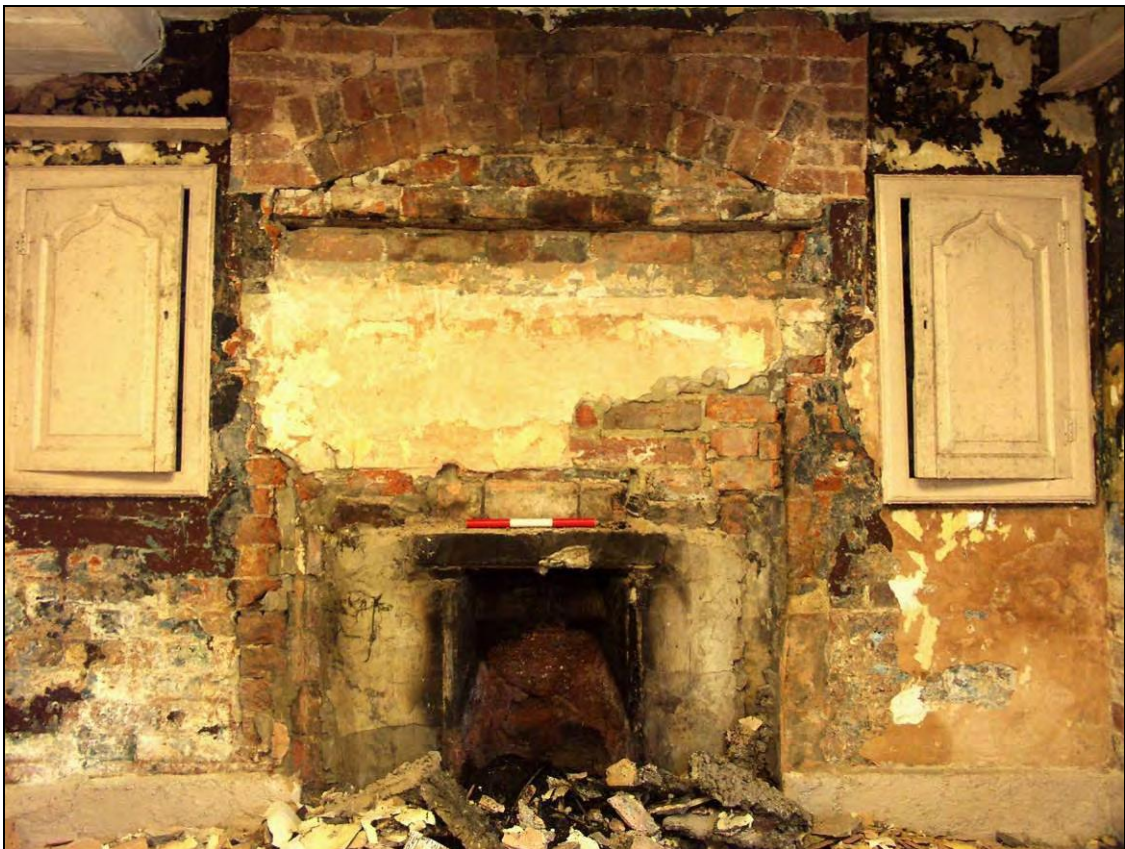
Figure 37: Detail of the fire place inserted in a larger blocked-up opening of a kitchen range (scale 300mm)
