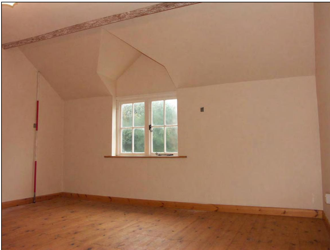
Figure 53: General view of room F-1 with new plaster board walls and floor boards (scale 2m)
