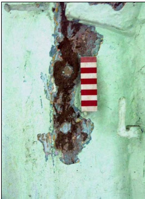
Figure 27: Surviving brace pegs on the S-E post
