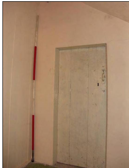
Figure 51: Doorway to room F-1 (scale 2m)
