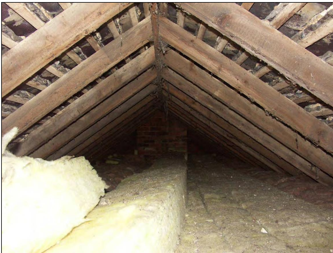
Figure 54: Inside the roof structure, looking south
