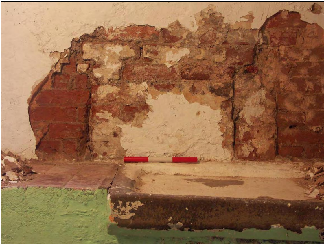
Figure 33: Former fire place next to salting trough, looking west (scale 300mm)
