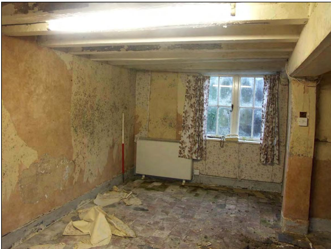
Figure 43: Room G-4, looking west (scale 1m)
