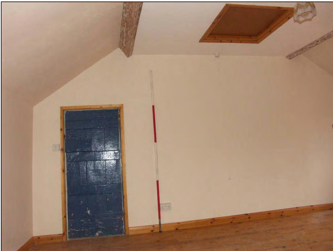
Figure 52: Room F-1 with ceiling hatch, looking south (scale 2m)
