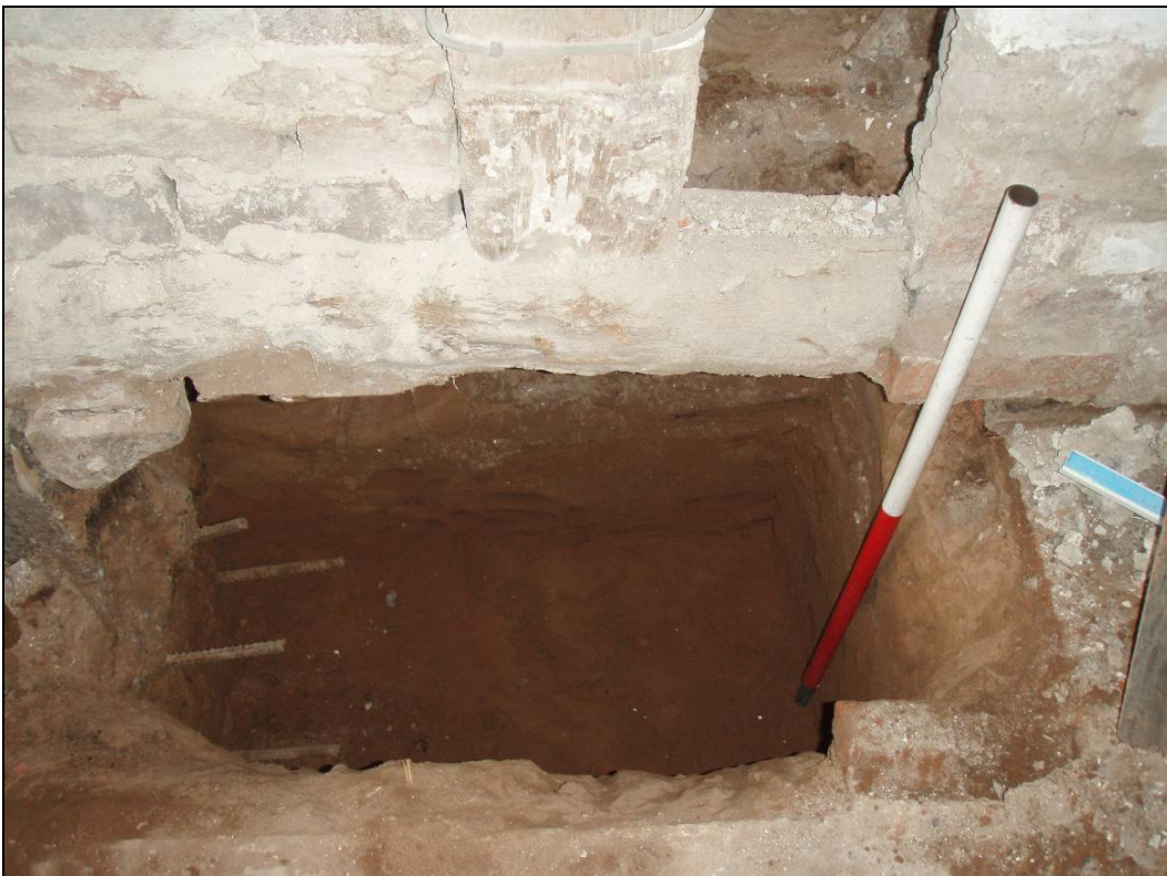
Figure 6: Underpinning trench beneath the timber-framed partition, looking south (scale 1m)
