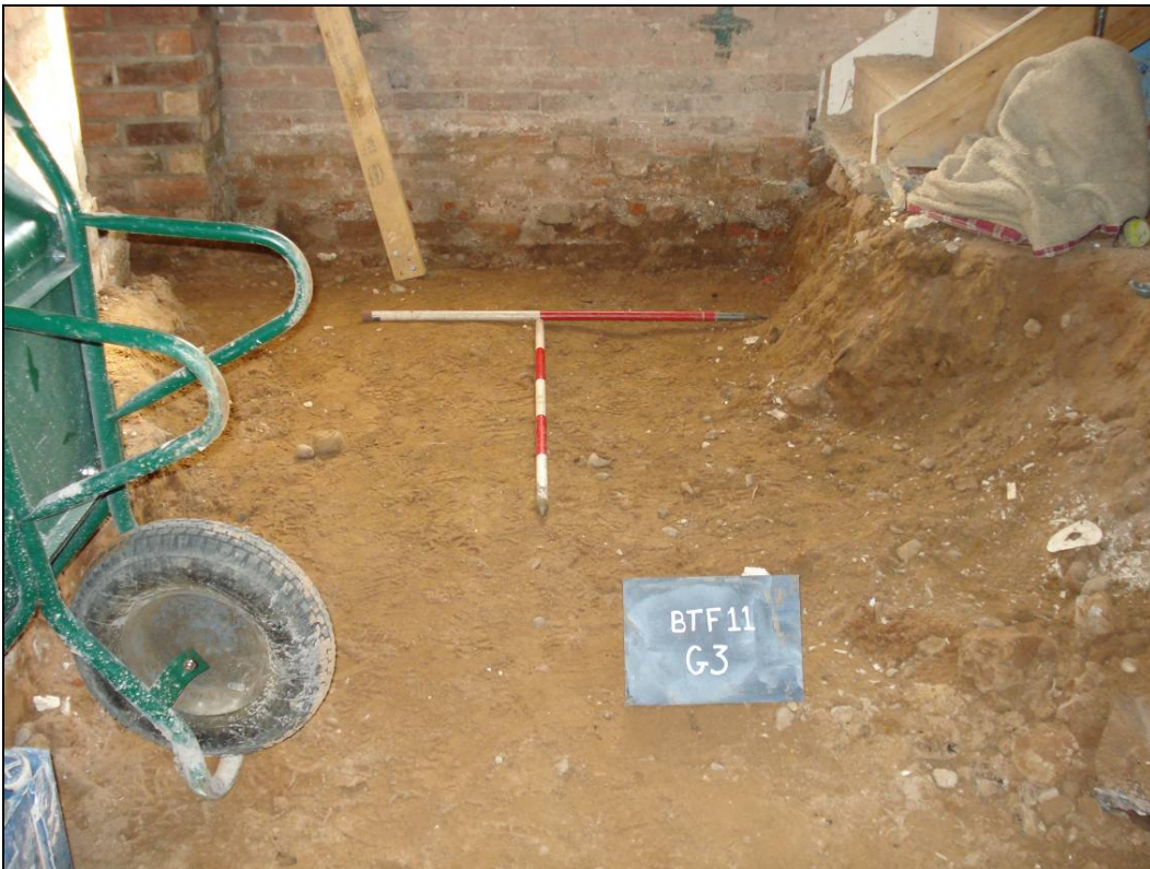
Figure 8: Subsoil layer exposed following general floor level reduction in the central room G-3
