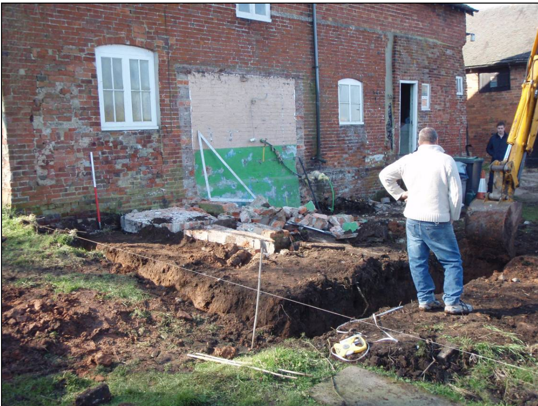
Figure 4: Foundation trench of the new extension, looking north-west
