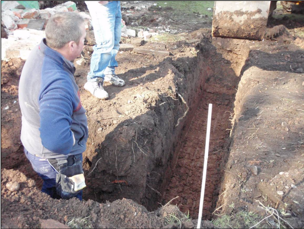
Figure 3: Excavation of the foundation trench for the new extension
