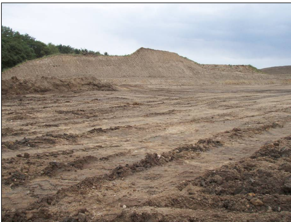
Figure 4. Removal of soil bund
