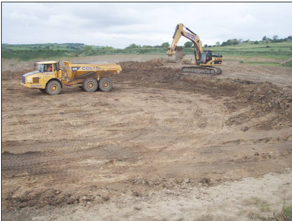
Figure 3. Soil removal
