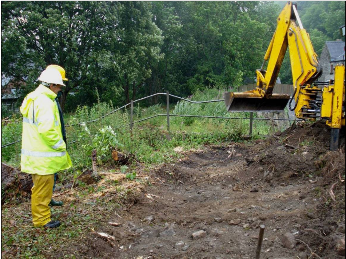
Figure 3: Trench 1 during excavation, looking east
