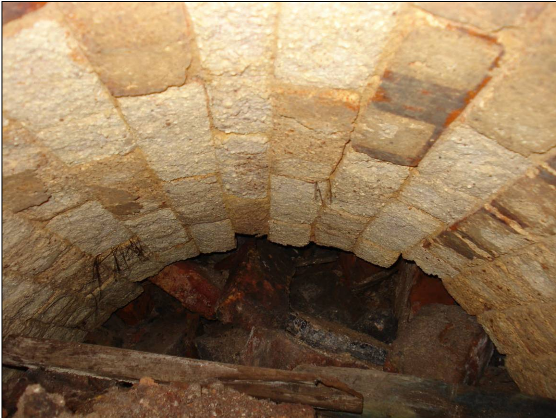
Figure 7: Vaulted flue opening, looking east
