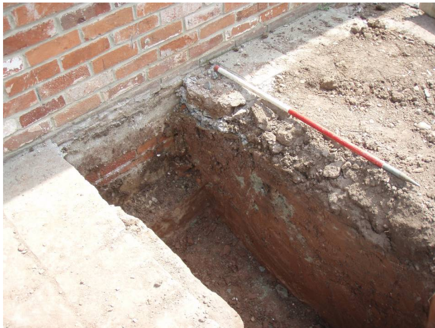
Figure 7. Section of the North Eastern-most trench showing the footings of the previous extension and the typical stratigraphy of the site (scale = 1m).
