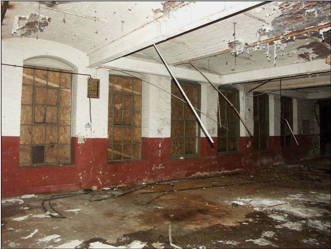
Figure 34: Ground floor of Building D with jack-arched ceiling
