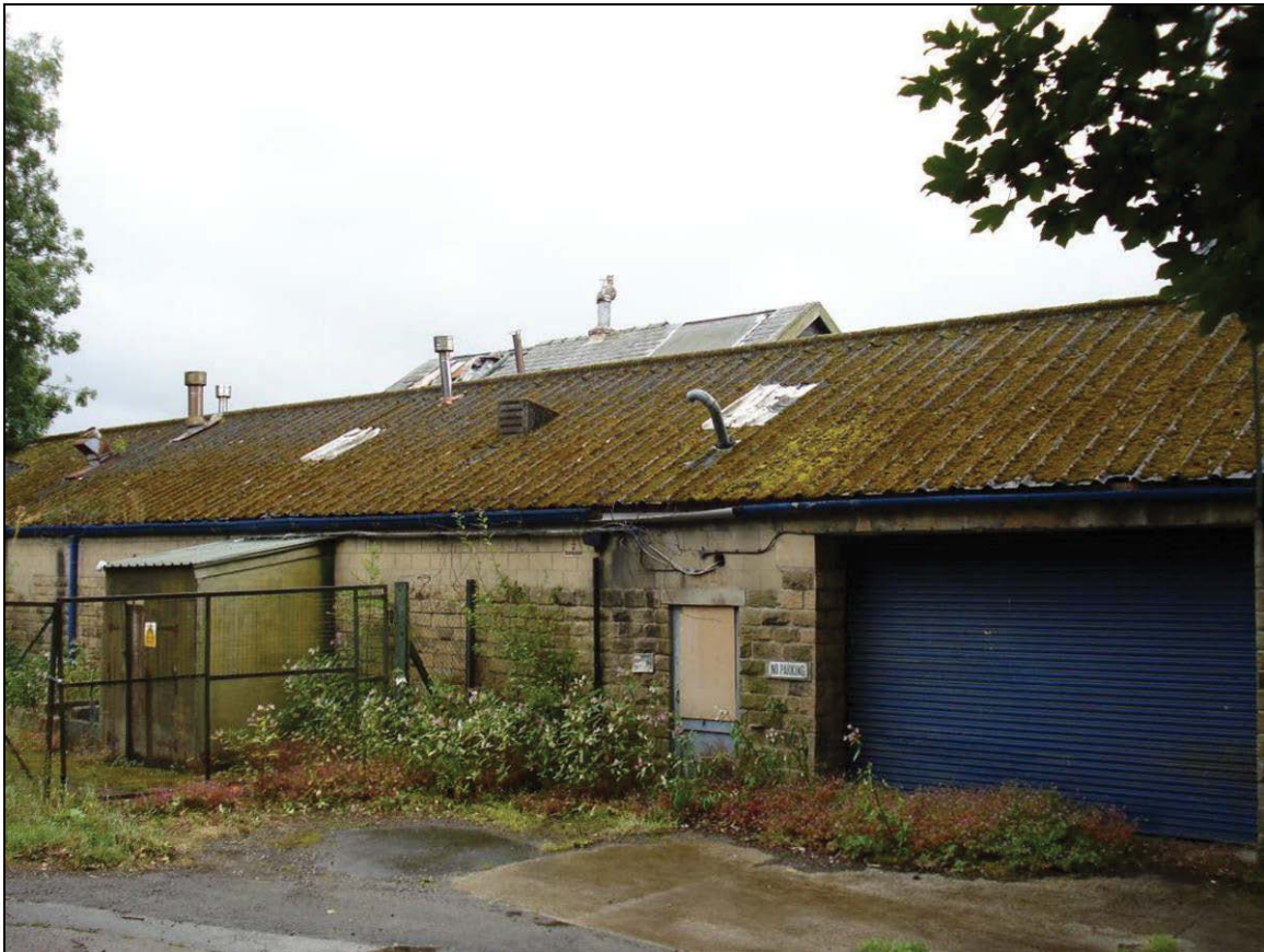
Figure 50: Eastern elevation of Building I
