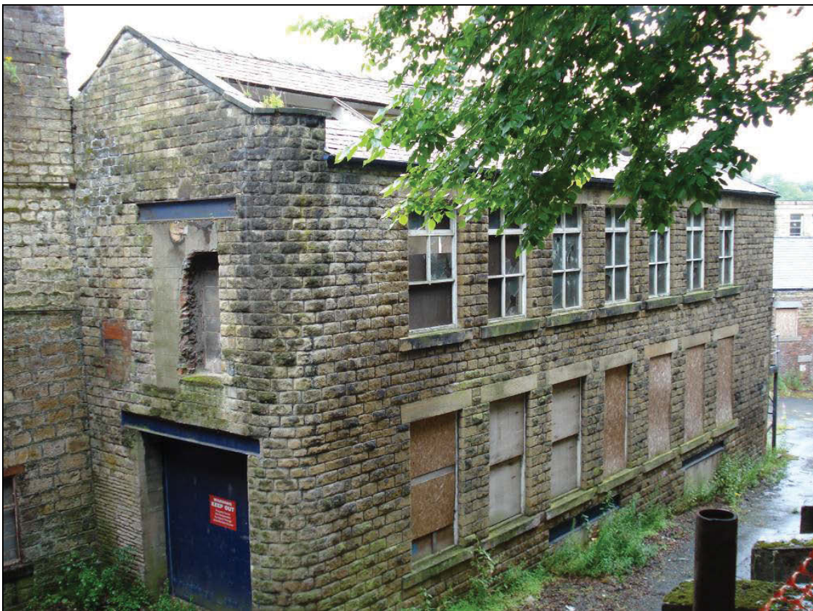
Figure 31: General view of the side eastern elevation of Building D
