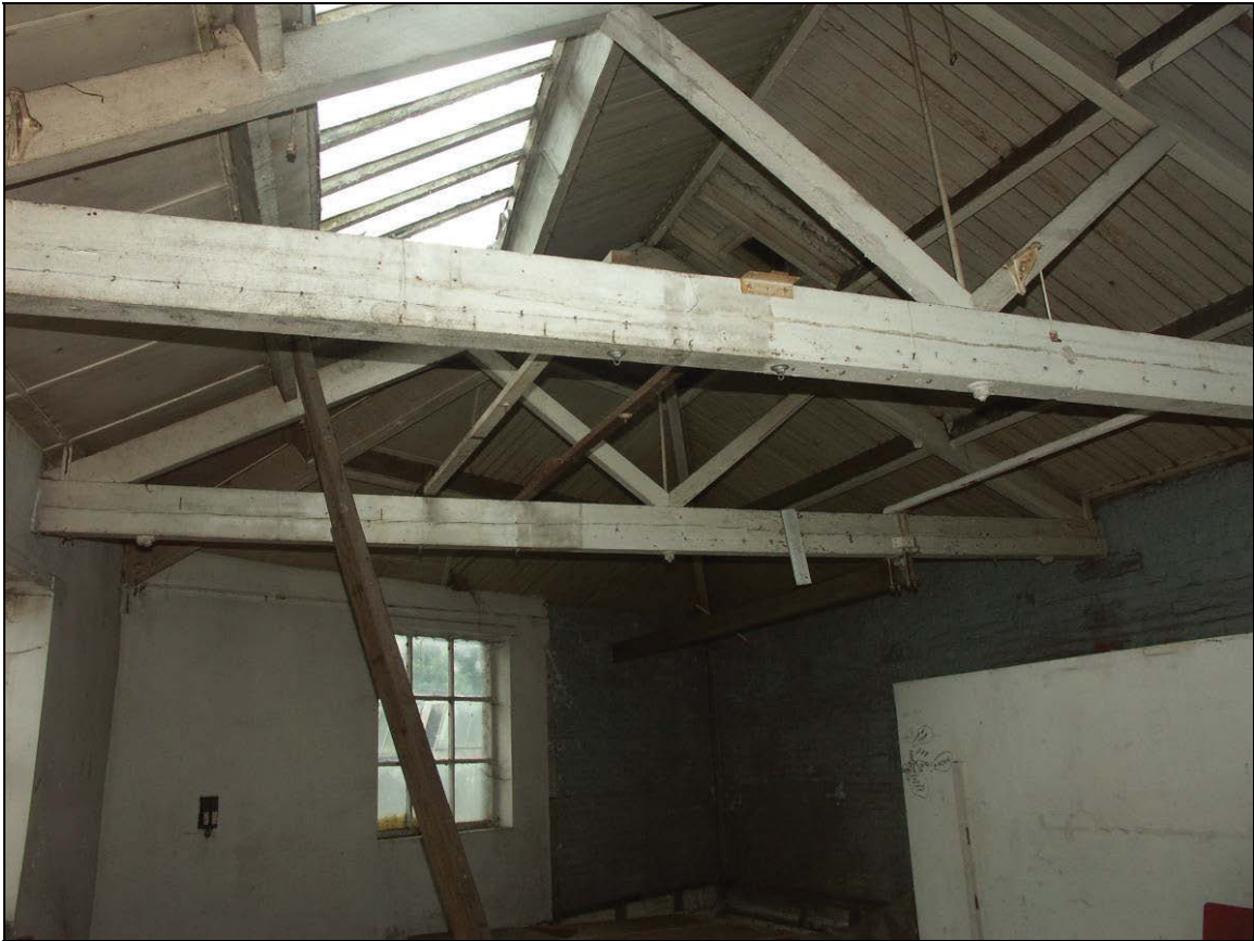
Figure 64: Roof structure of Building Q
