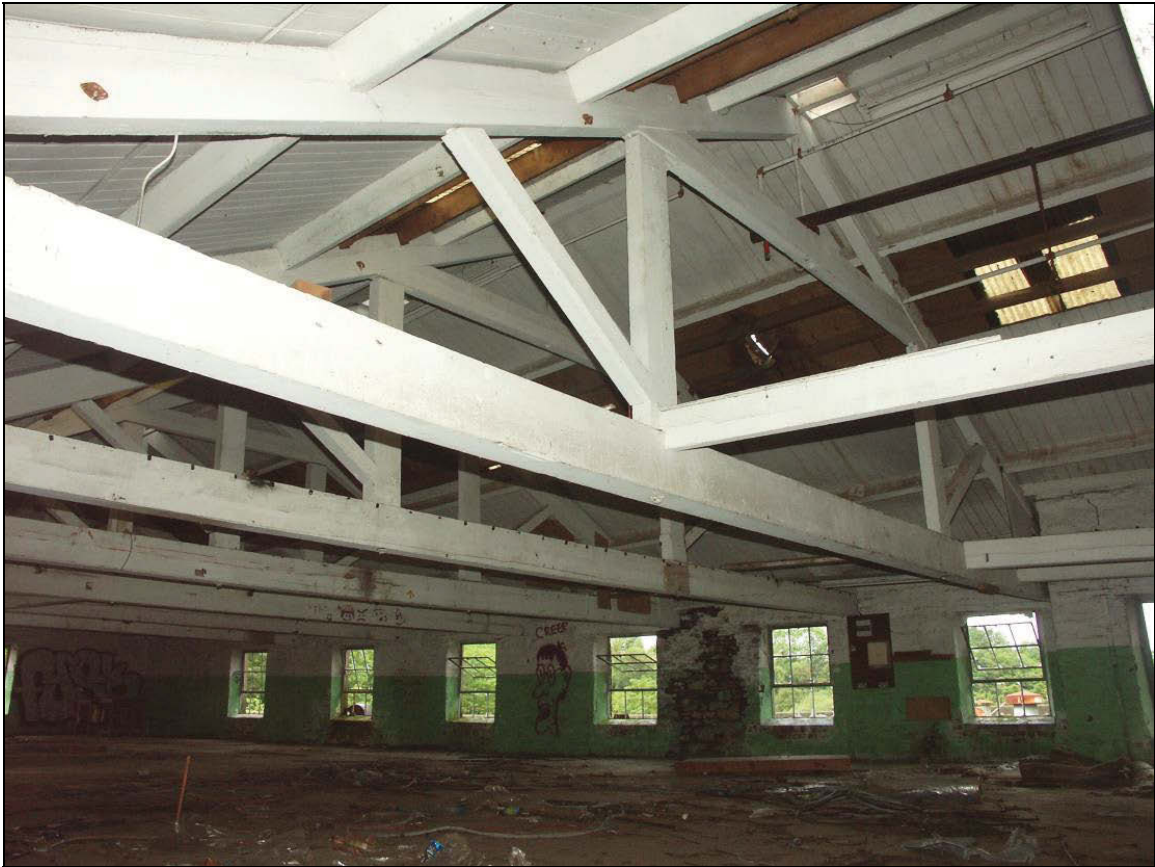
Figure 45: Roof structure of Building G
