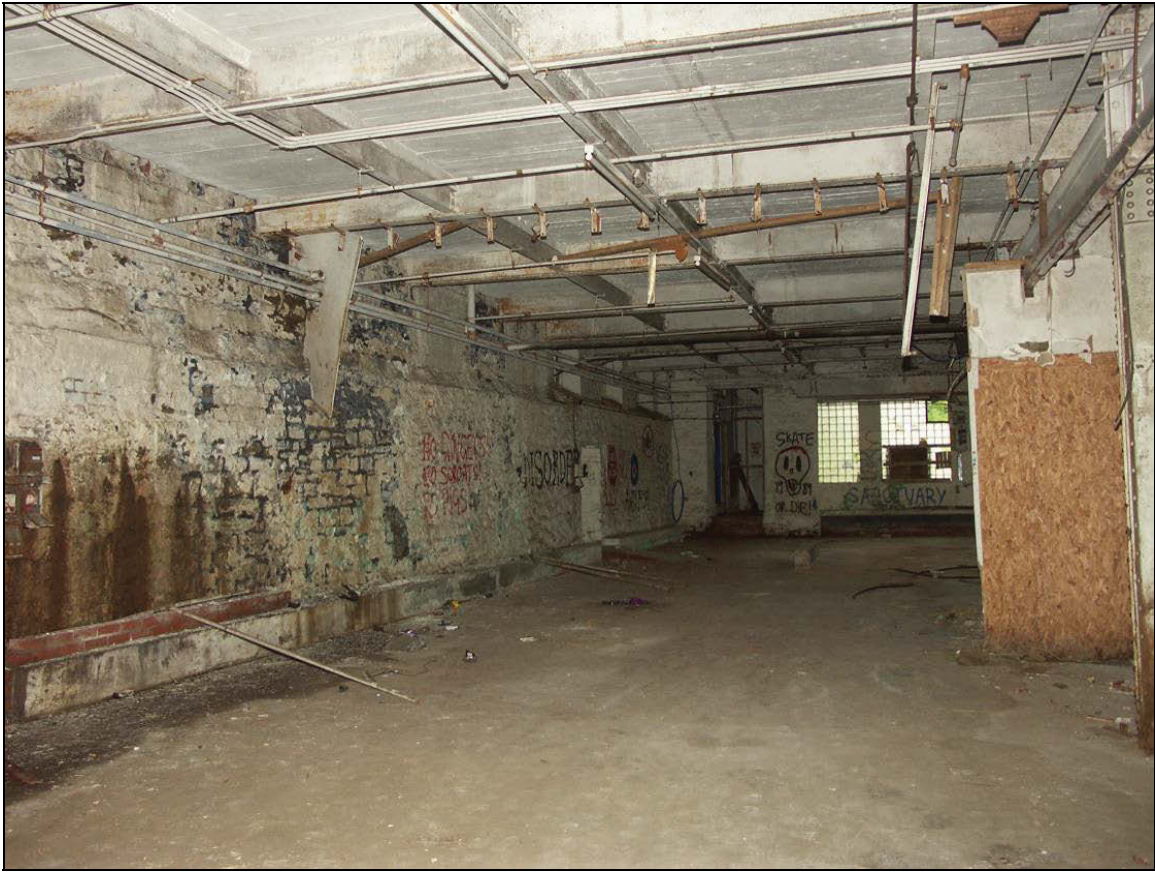
Figure 48: General view of the interior of Building H
