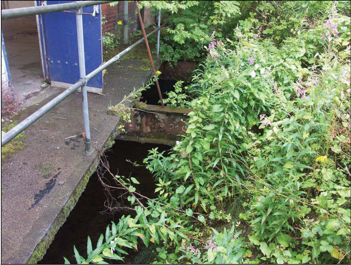
Figure 18: Viewpoint 9 –Sluice to the south of Building S
