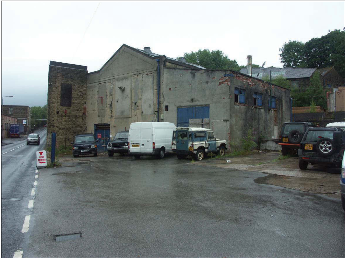
Figure 56: Front elevation of Building L
