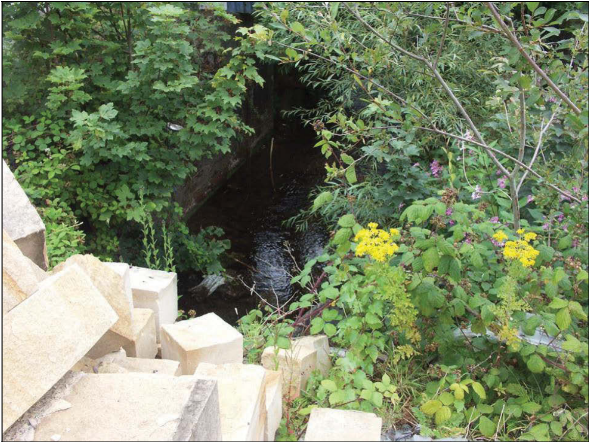
Figure 16: Viewpoint 7 – Sluice within the stone yard
