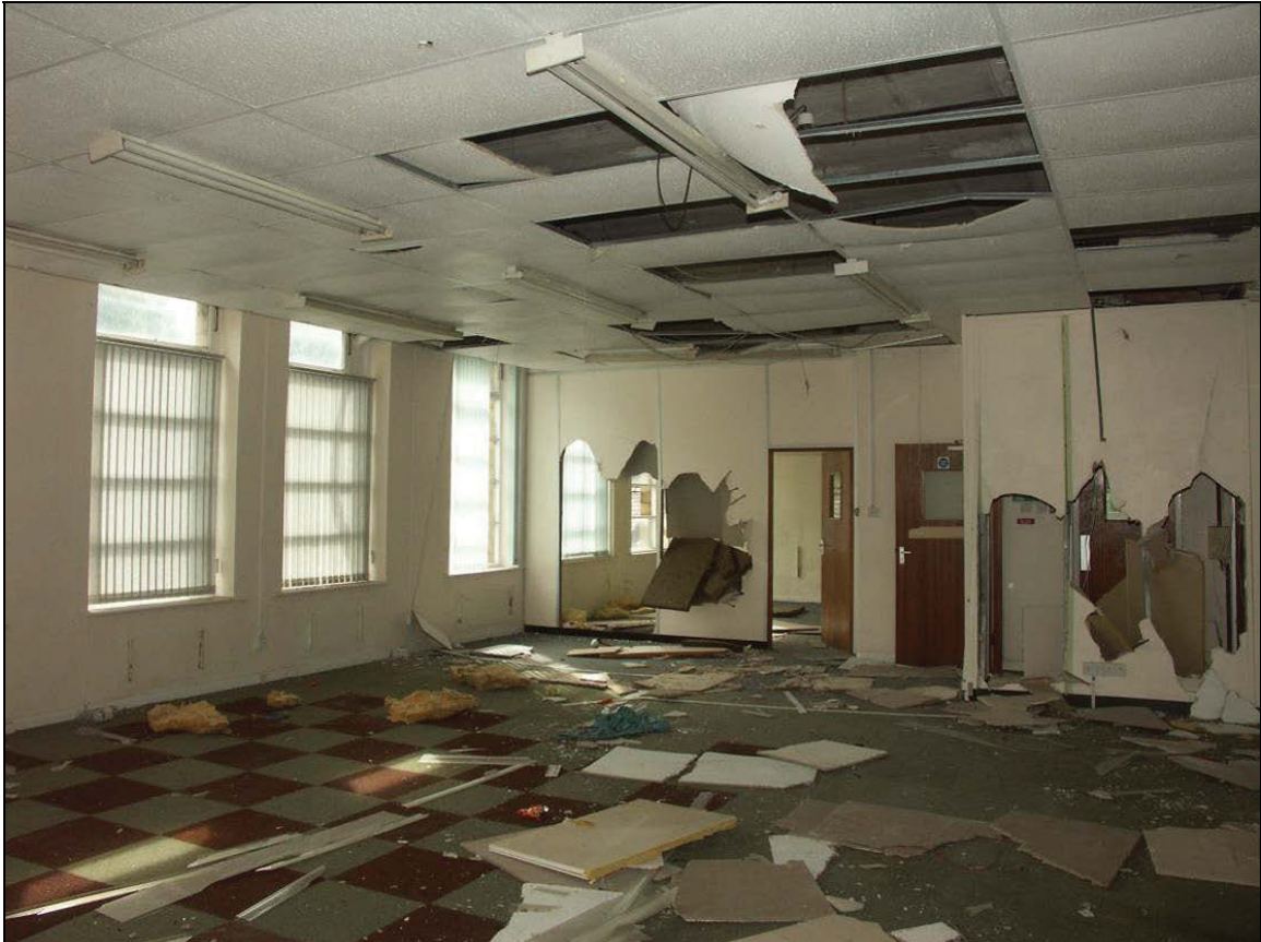
Figure 80: Second floor of Building U
