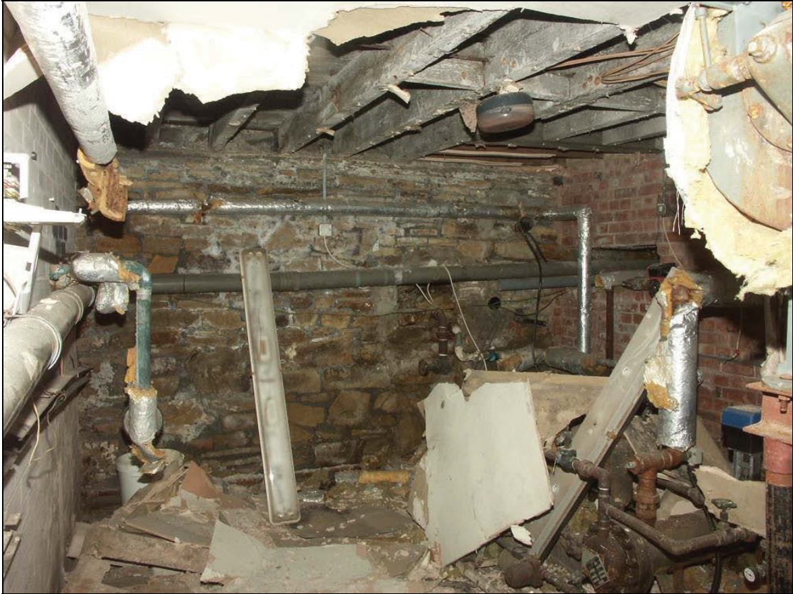
Figure 75: Eastern wall of basement
