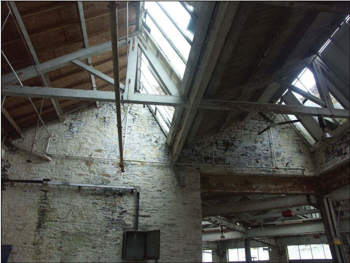
Figure 40: North-light roof structure of Building F
