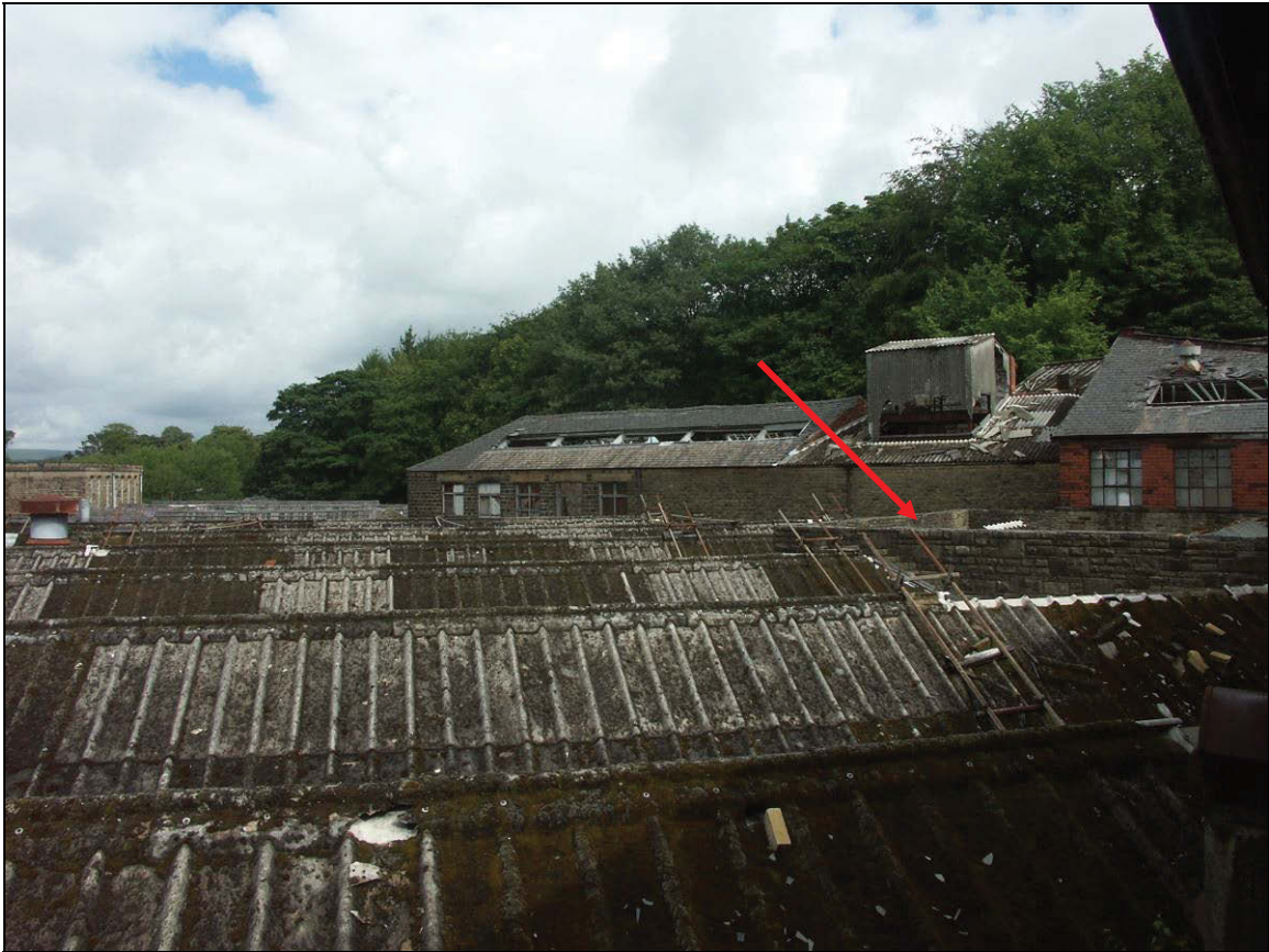
Figure 38: View of the parapet of Building F
