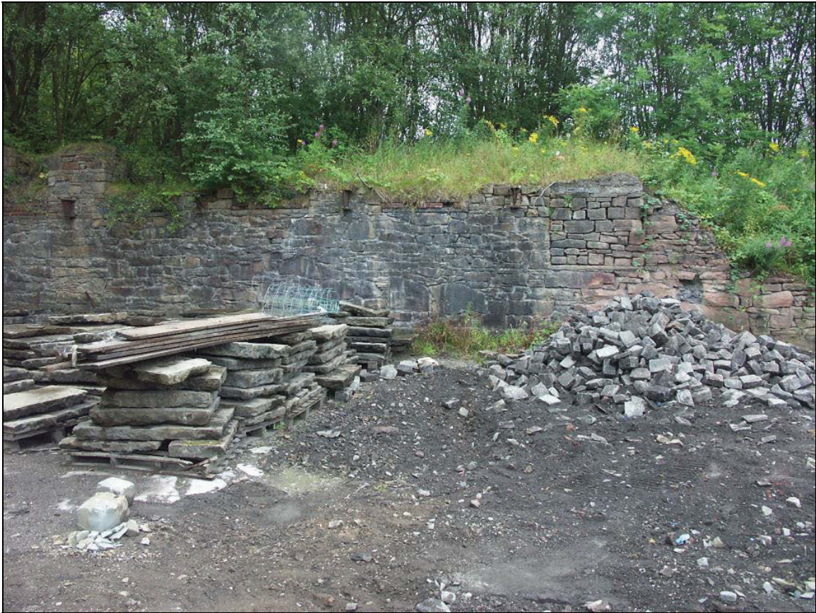
Figure 10: Viewpoint 1 –Remains of a former building acting currently as a retaining wall
