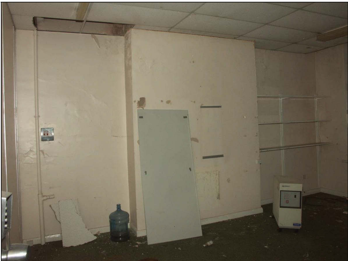
Figure 78: Chimney breast within the western side of the ground floor
