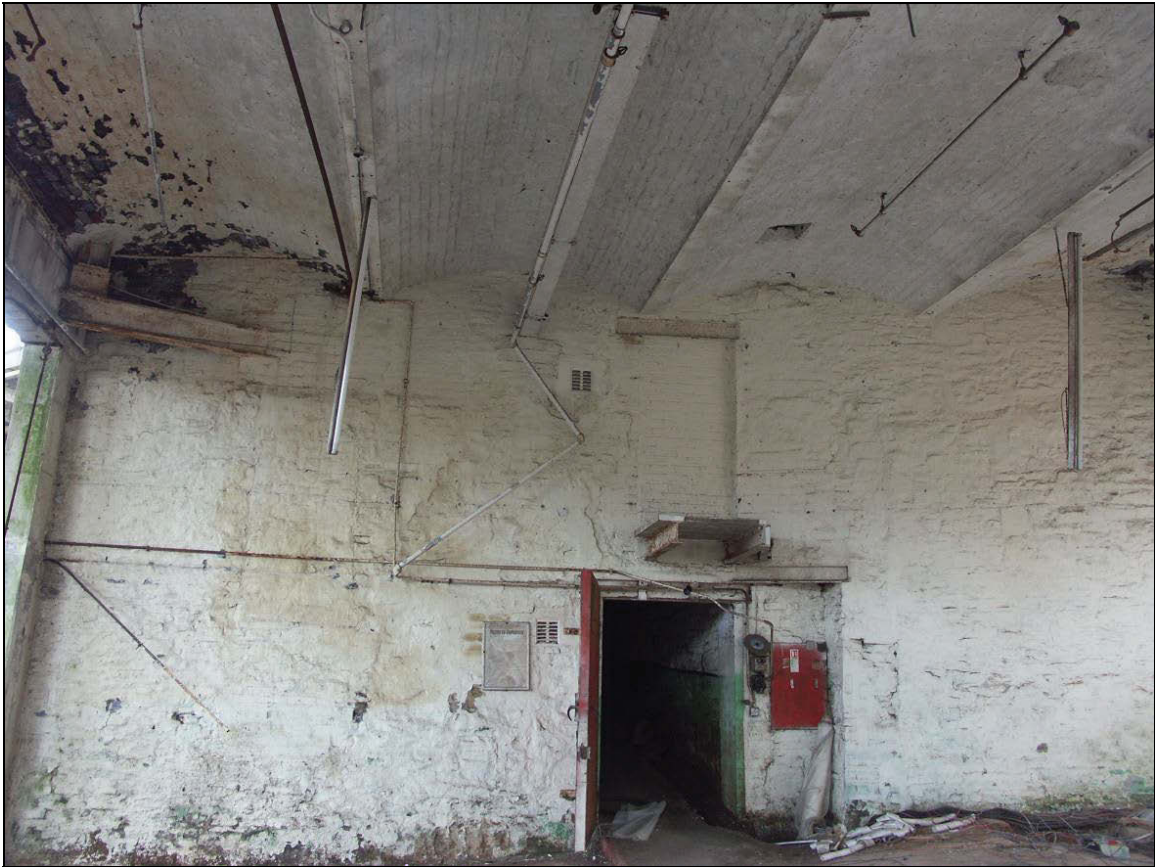
Figure 43: Jack-arched ceiling in the basement of Building G
