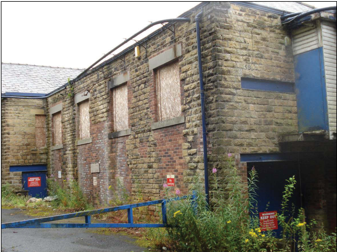
Figure 26: Rear elevation of Building B
