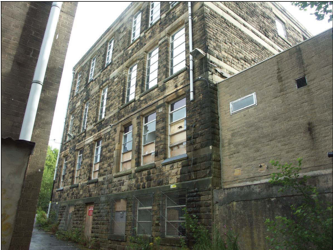
Figure 74: Rear elevation of Building U showing the basement floor
