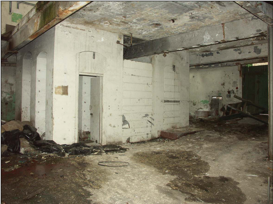
Figure 57: Internal view of Building L
