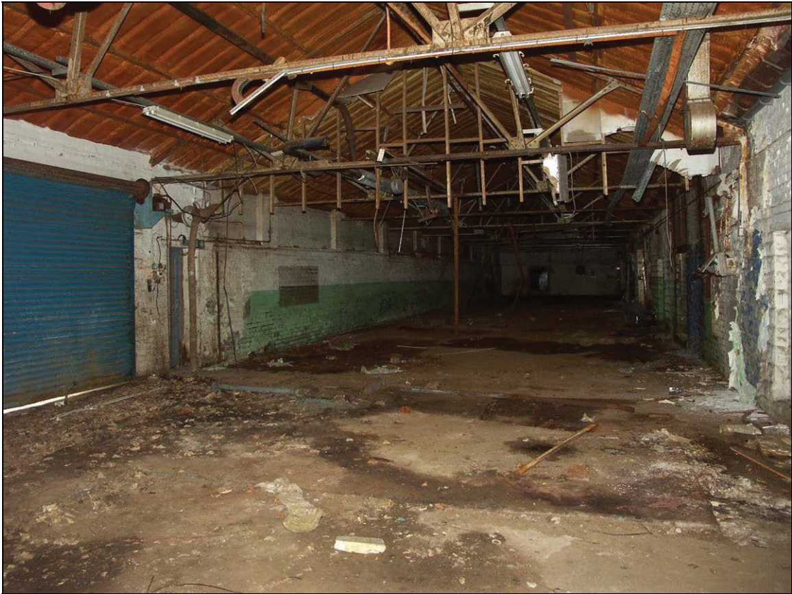
Figure 51: Roof structure of Building I
