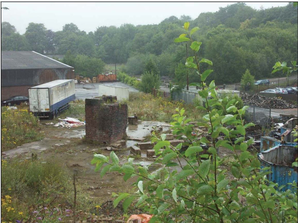
Figure 15: Viewpoint 6 –Brick base of a possible former tank
