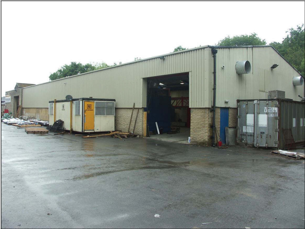
Figure 60: General view of Building O
