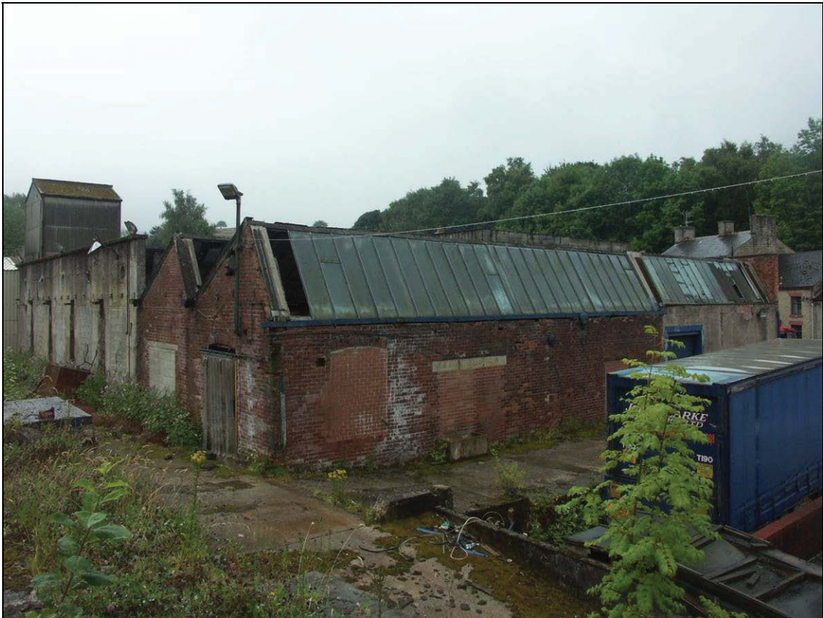
Figure 58: General view of Building M
