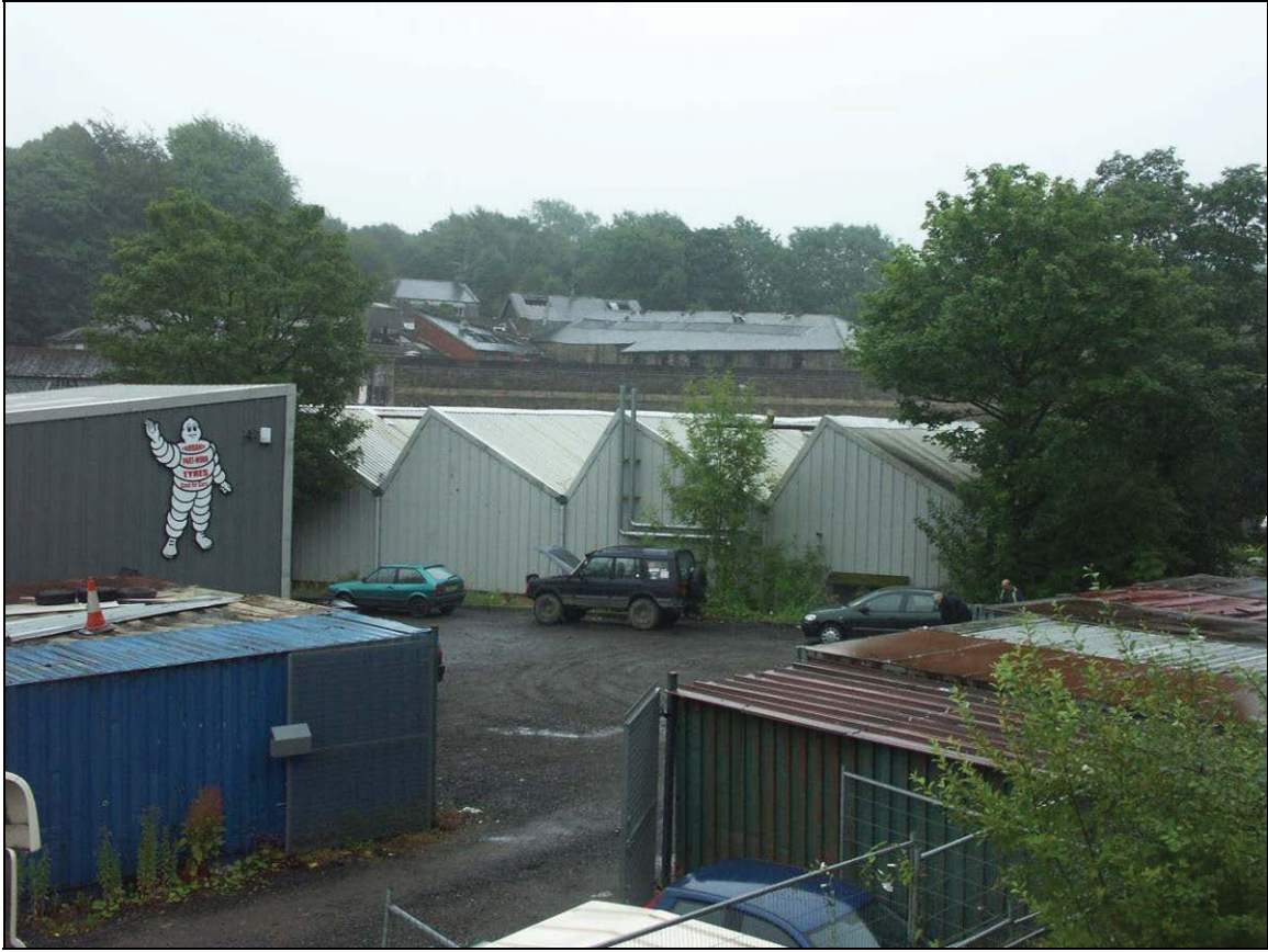
Figure 68: Rear view of Building S
