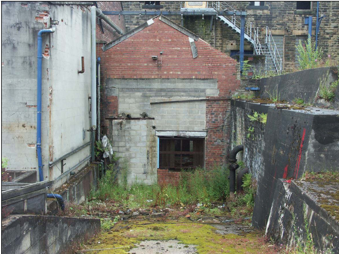
Figure 54: Southern gable end of Building K
