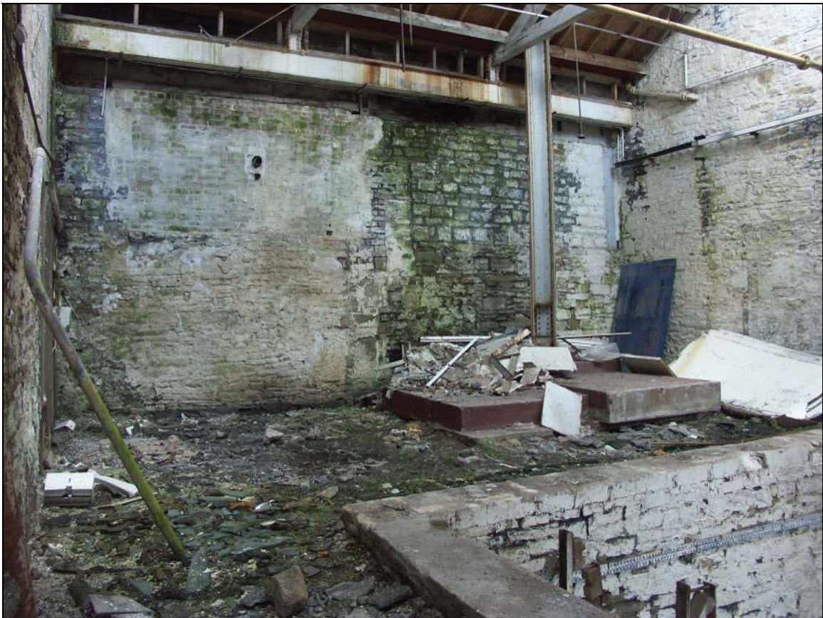
Figure 39: Internal view of Building F
