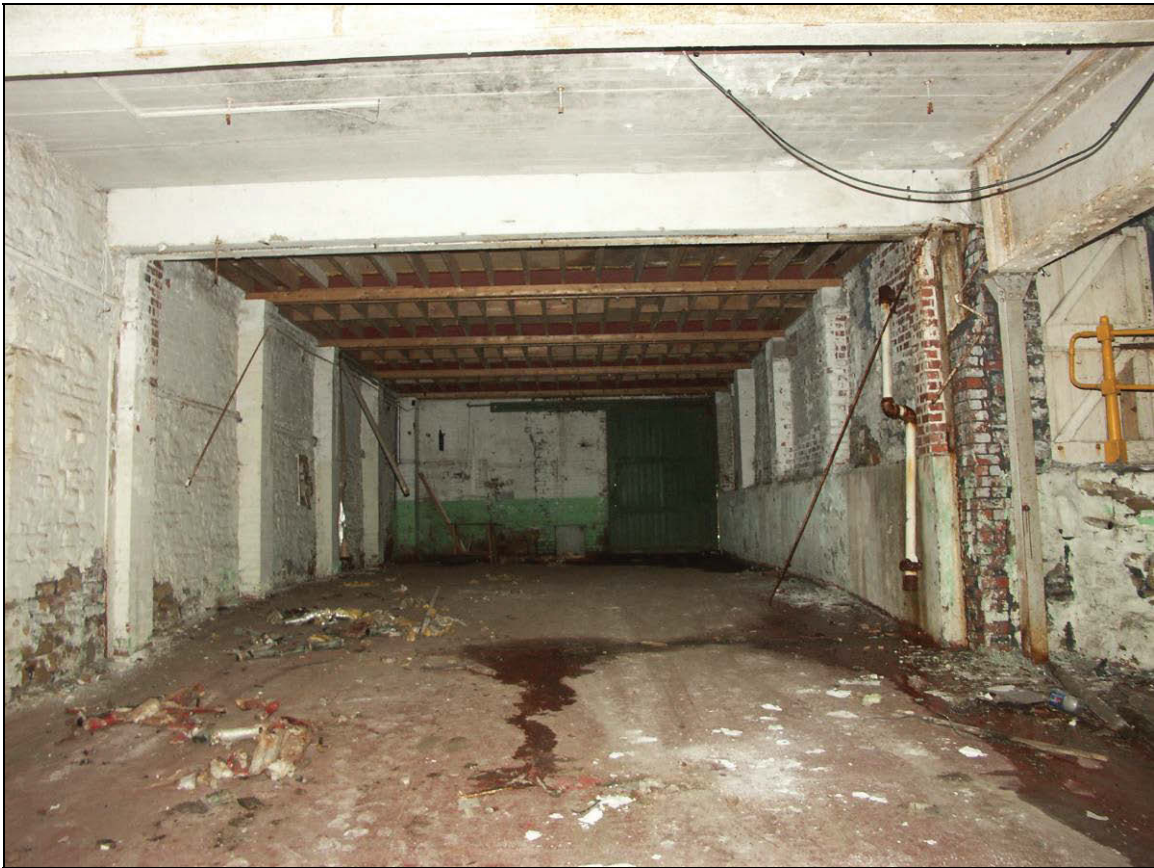
Figure 27: Internal view of Building B
