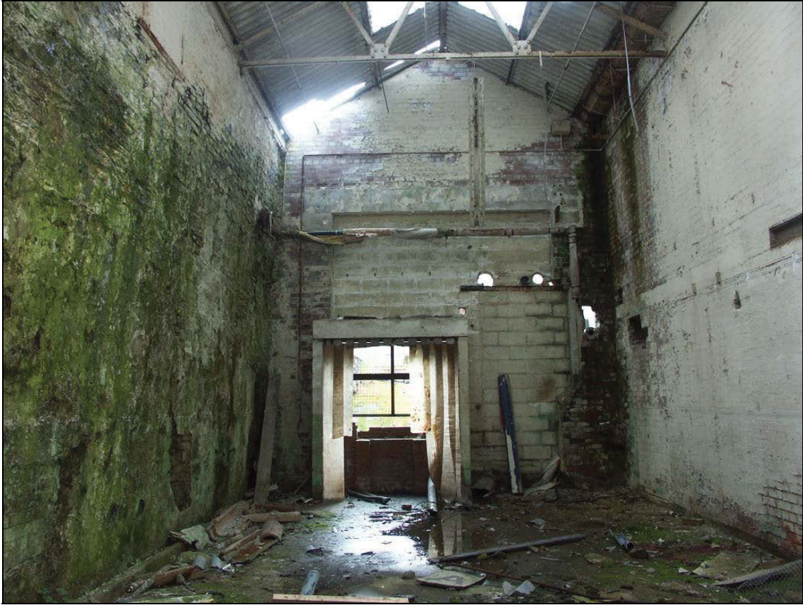
Figure 55: Internal view of Building K
