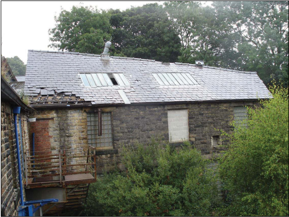
Figure 52: Western elevation of Building J
