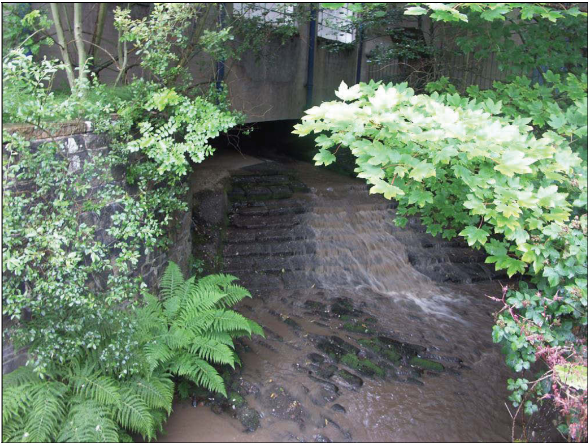
Figure 19: Viewpoint 10 –Weir adjacent to Building M
