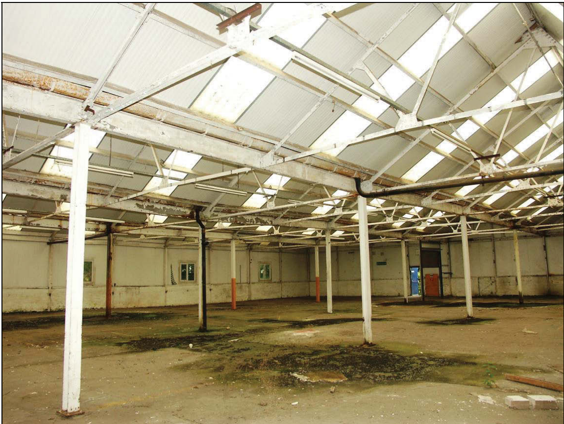
Figure 69: Internal view of Building S
