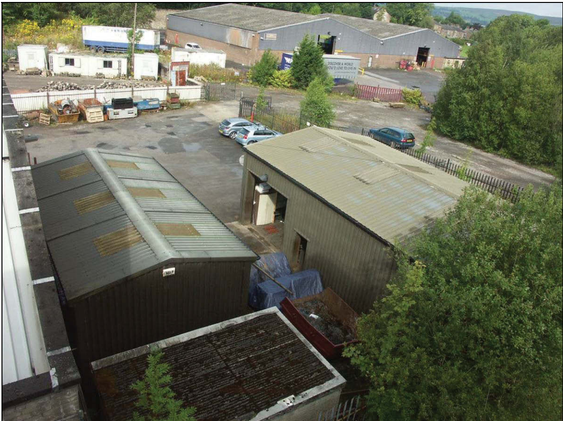
Figure 83: Steel sheds adjacent to Building W
