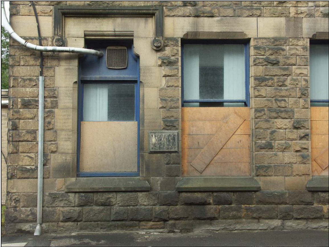
Figure 73: Detail of window openings within the front elevation of Building U
