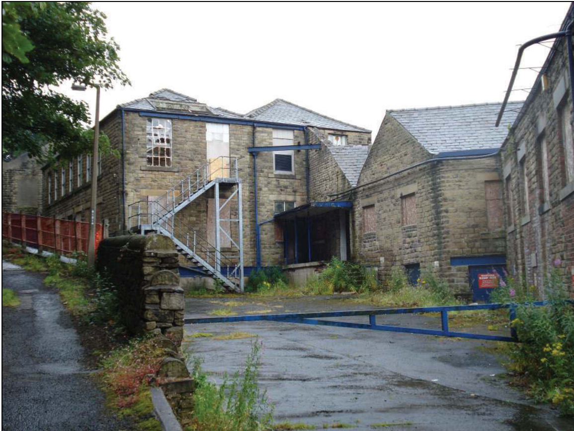
Figure 30: Northern elevation of Building D with double hipped roof
