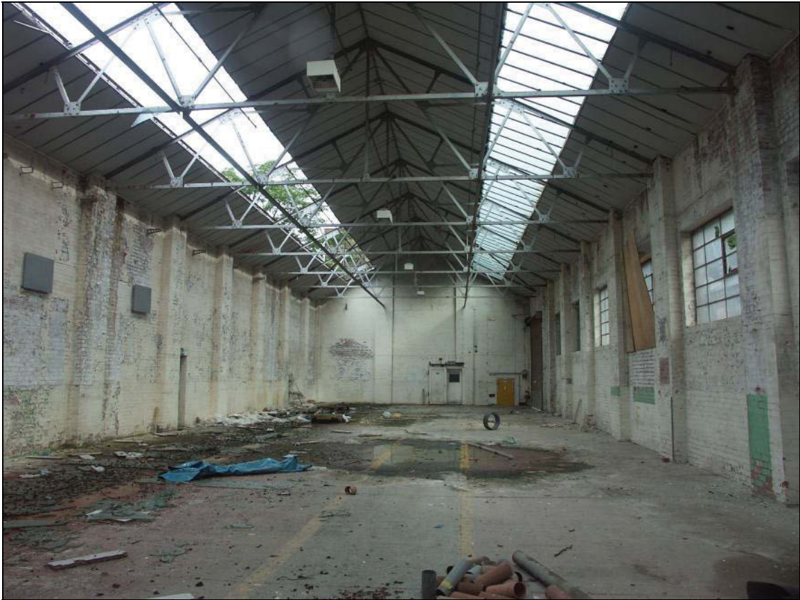
Figure 71: Internal view of Building T
