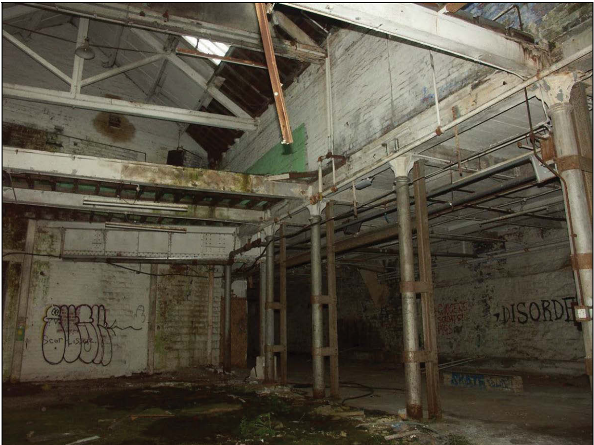
Figure 53: Surviving cast-iron columns supporting timber king-post trusses in Building J
