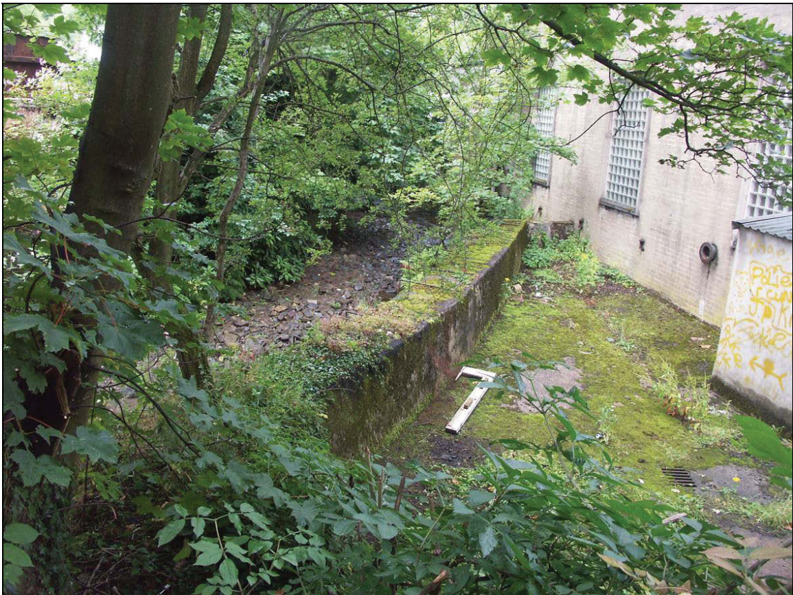
Figure 17: Viewpoint 8 – Sluice to the south of Building W
