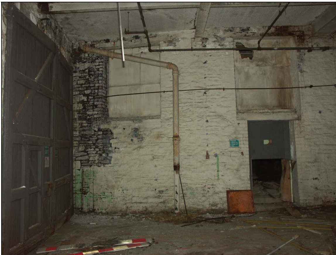
Figure 47: Internal north-eastern corner of Building H
