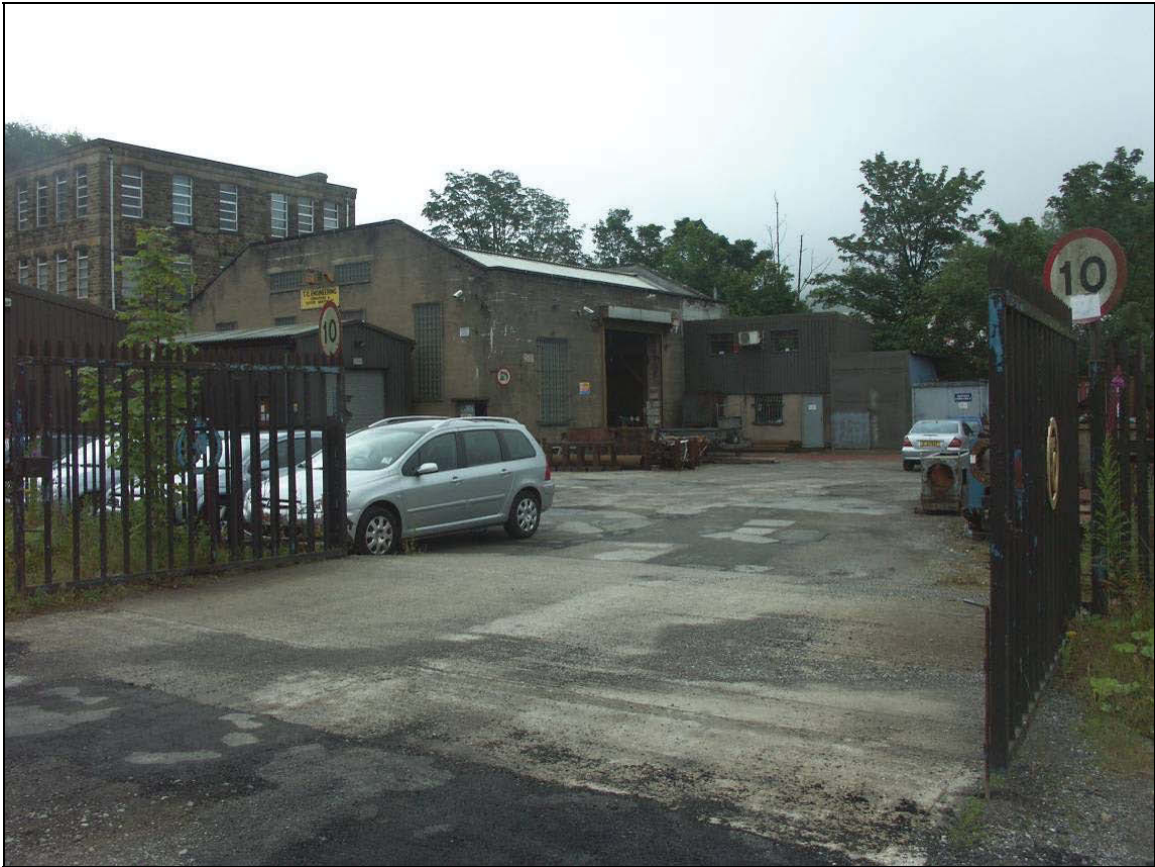
Figure 82: Northern and western elevations of Building W
