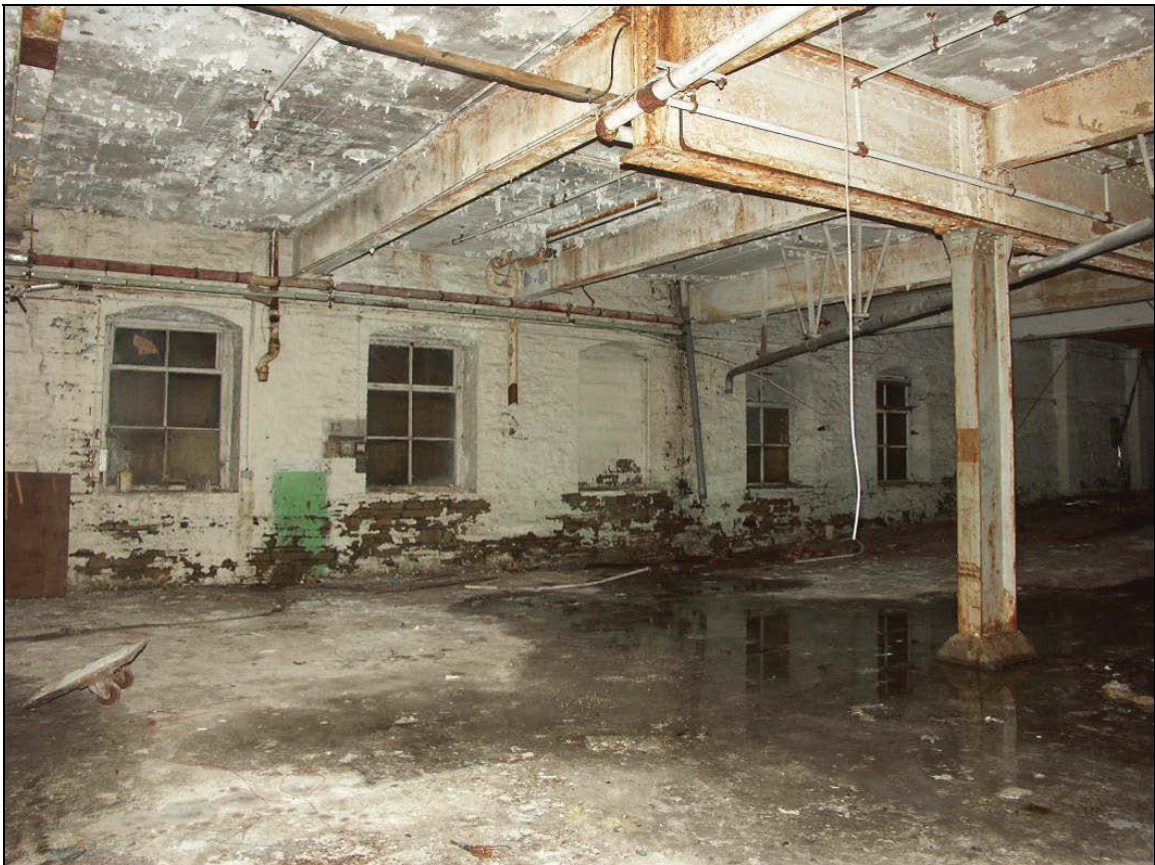
Figure 29: Internal view of Building C
