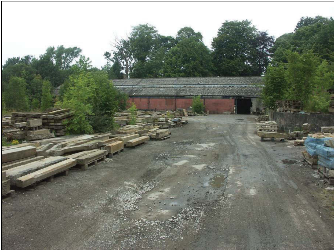
Figure 84: Southern elevation of Building X
