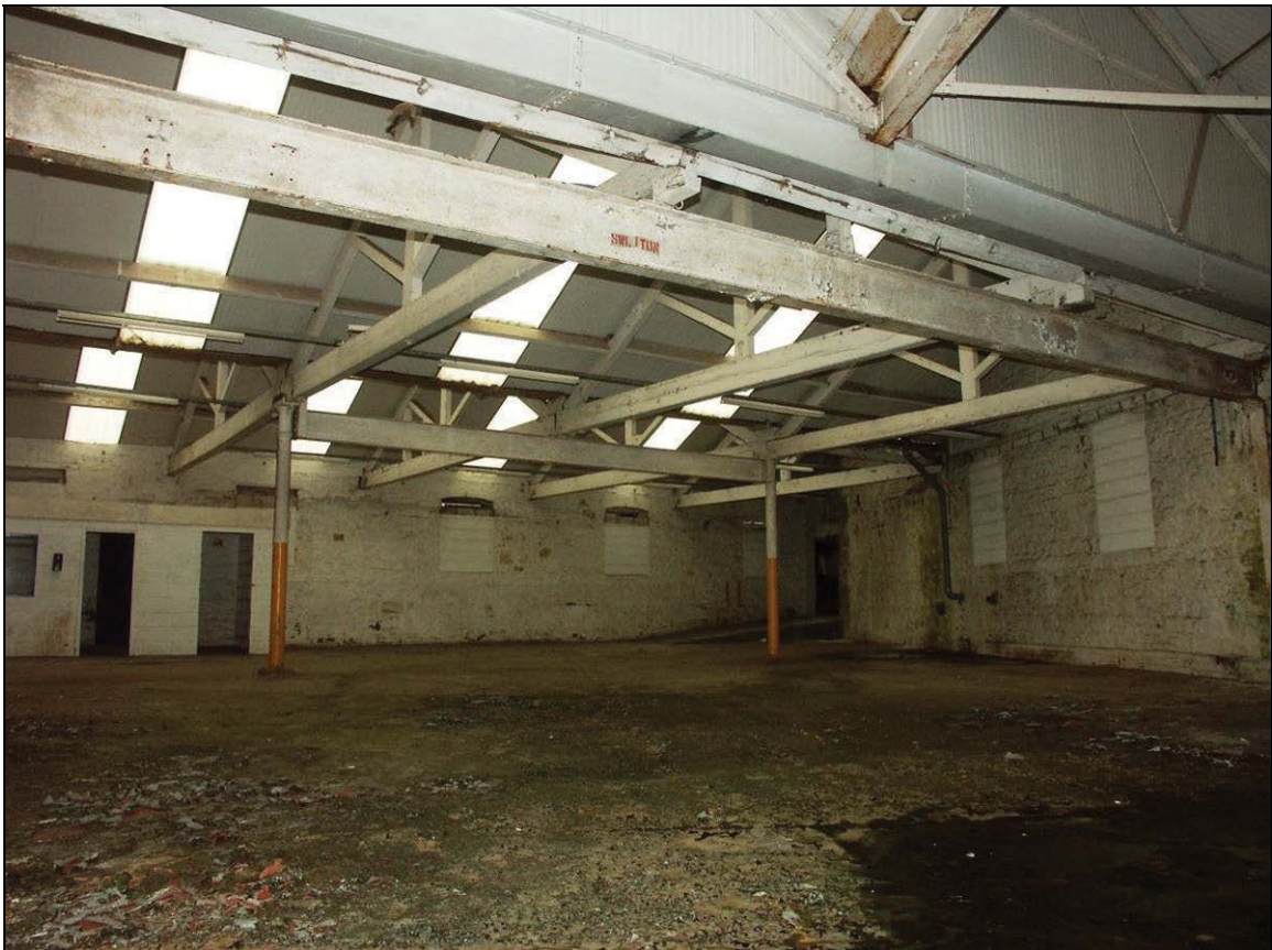
Figure 66: Building R with cast-iron columns supporting double king-post trusses
