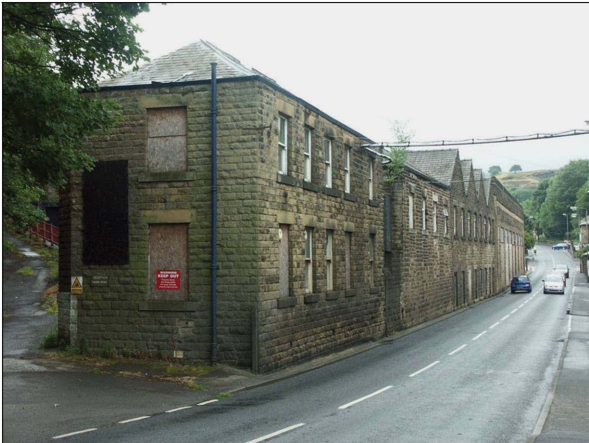
Figure 23: Charlestown Road with Building A in the foreground
