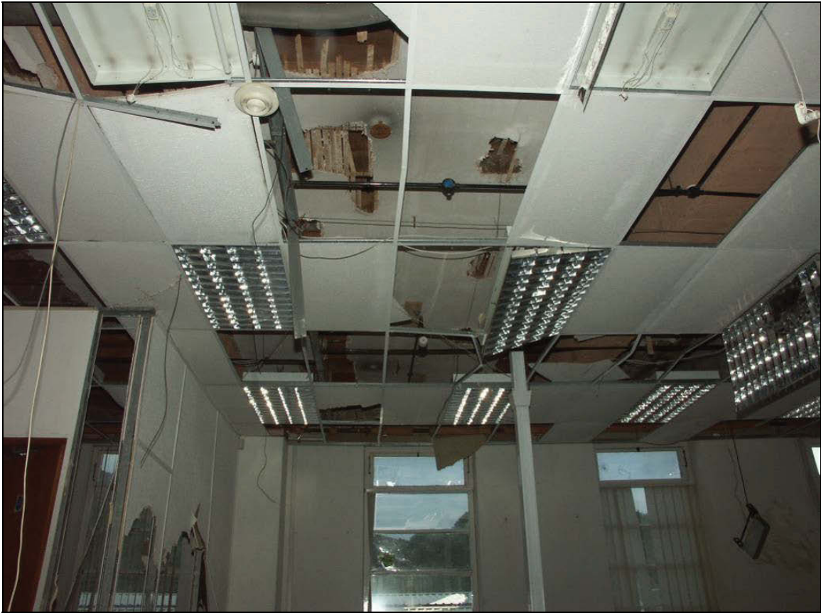
Figure 79: First floor of Building U
