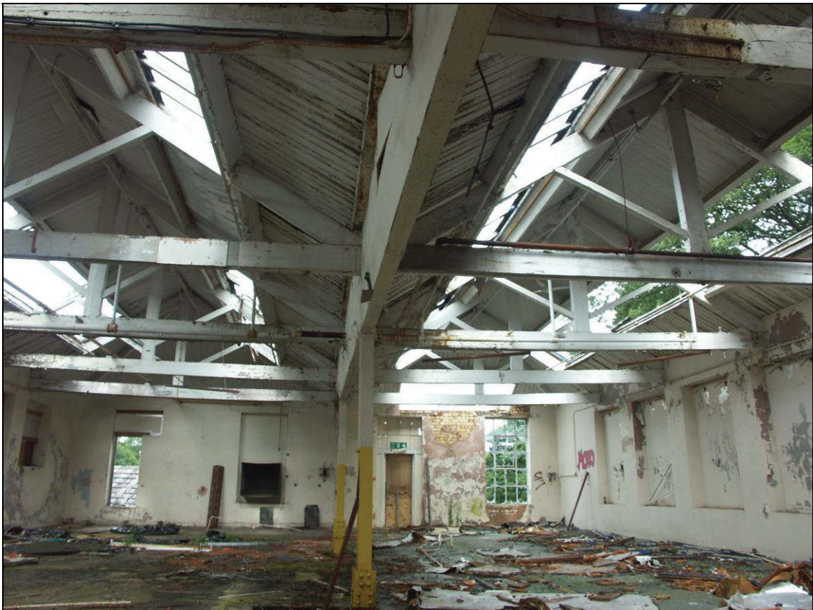
Figure 35: Roof structure of Building D
