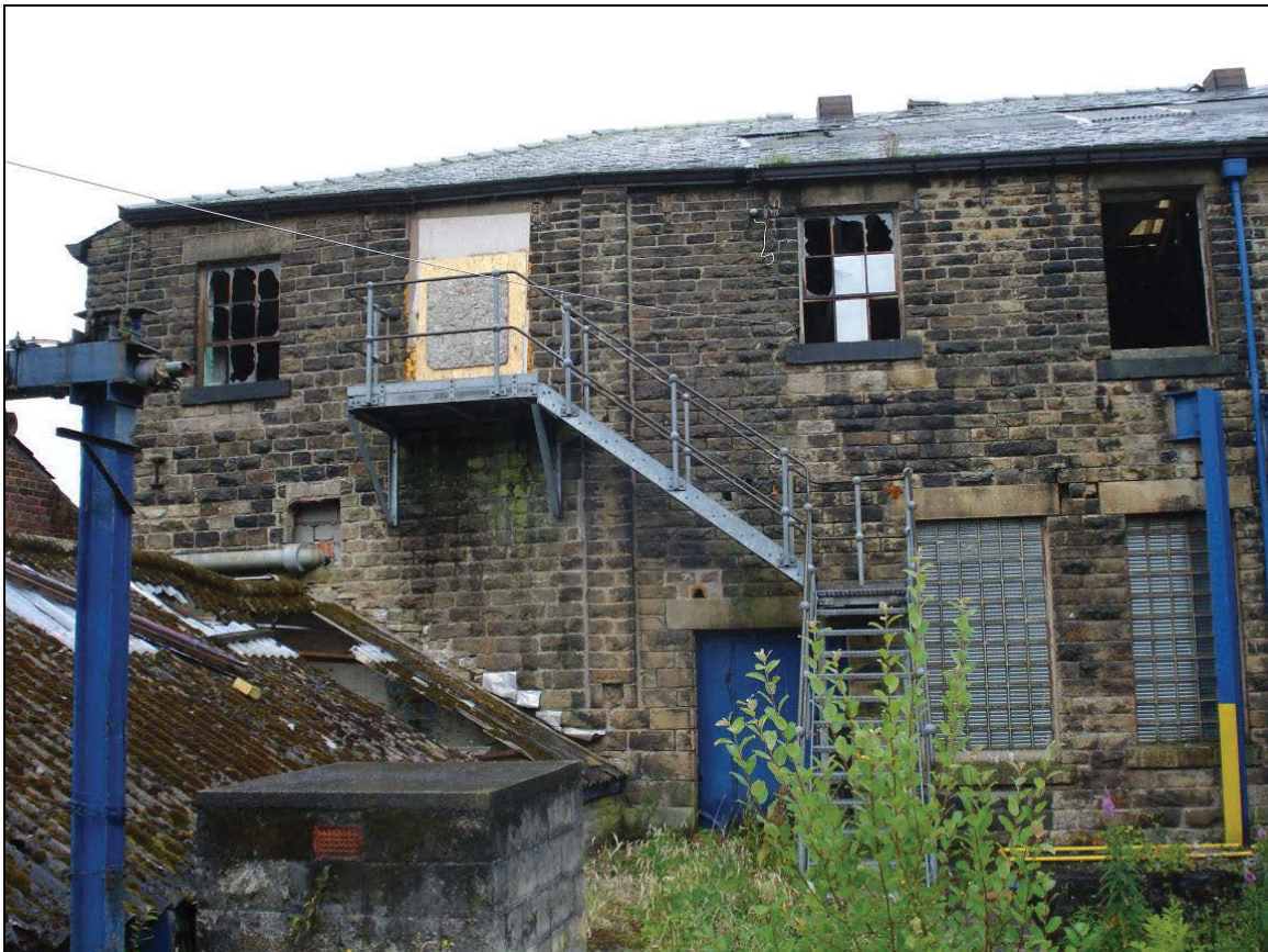
Figure 42: South-western end of Building G
