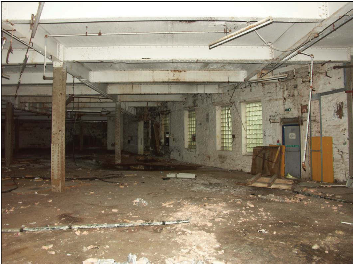
Figure 44: Internal view of the ground floor of Building G
