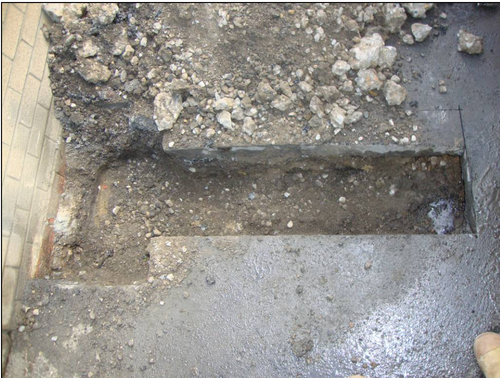
Figure 4. Excavation for eastern gantry.
