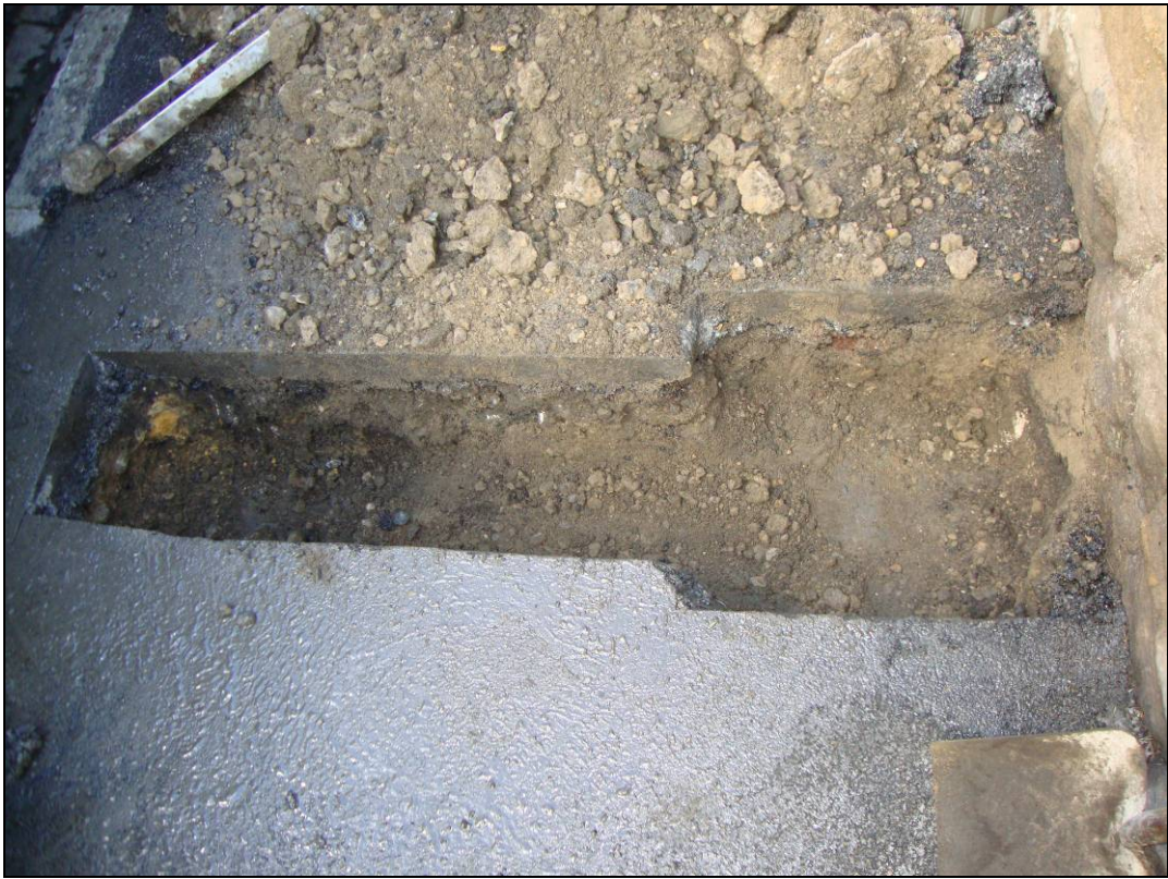
Figure 5. Excavation for western gantry.
