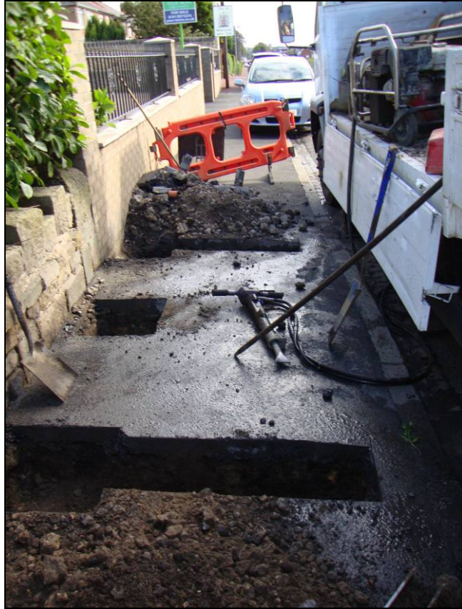
Figure 3. Extent and arrangement of excavations.
