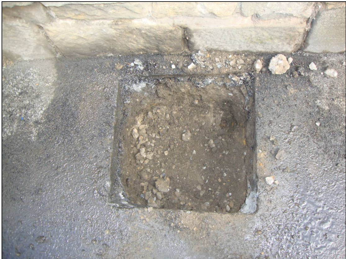
Figure 6. Excavation for intermediate post.
