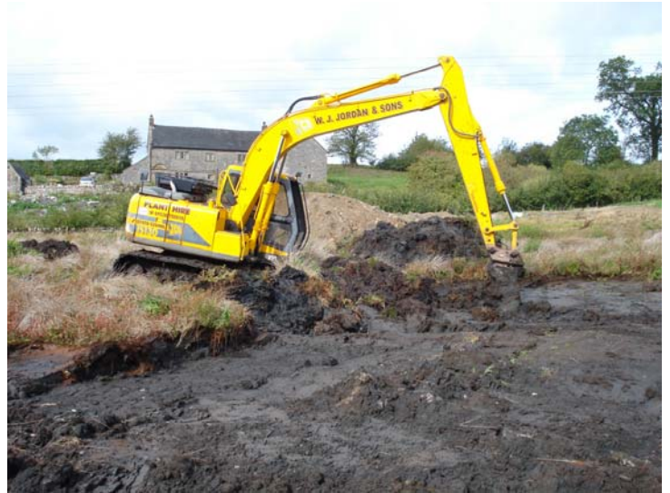
Working shot of the topsoil strip
