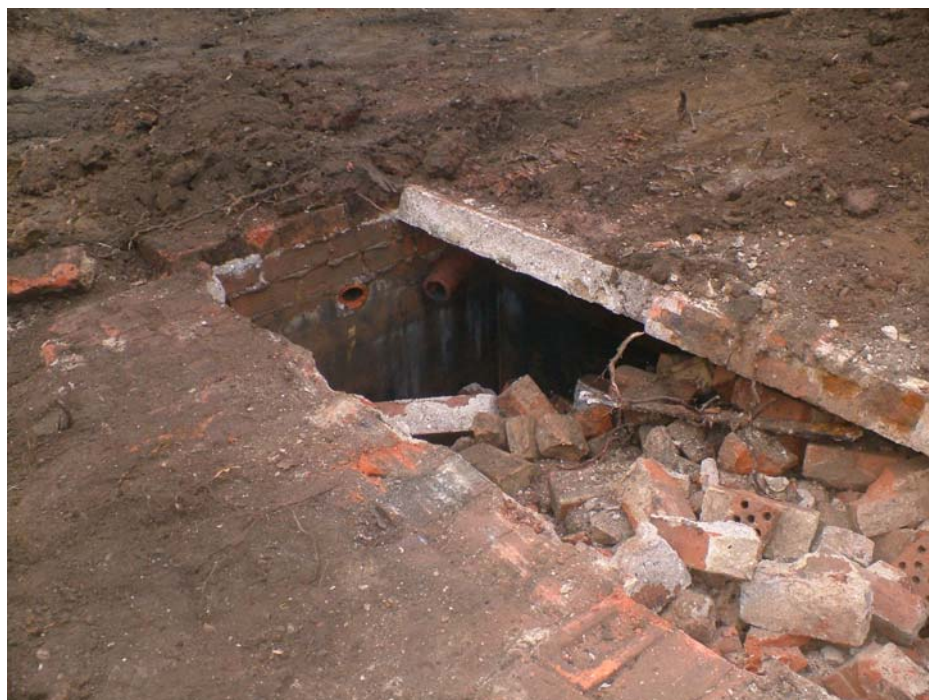
Figure 4: Storage tank after demolition. Note the concrete lining and pipes.
