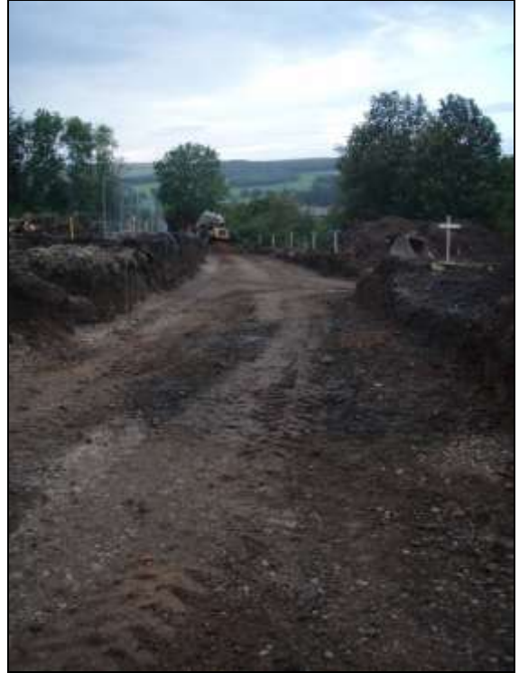
Looking south across the site at Nursery Gardens
