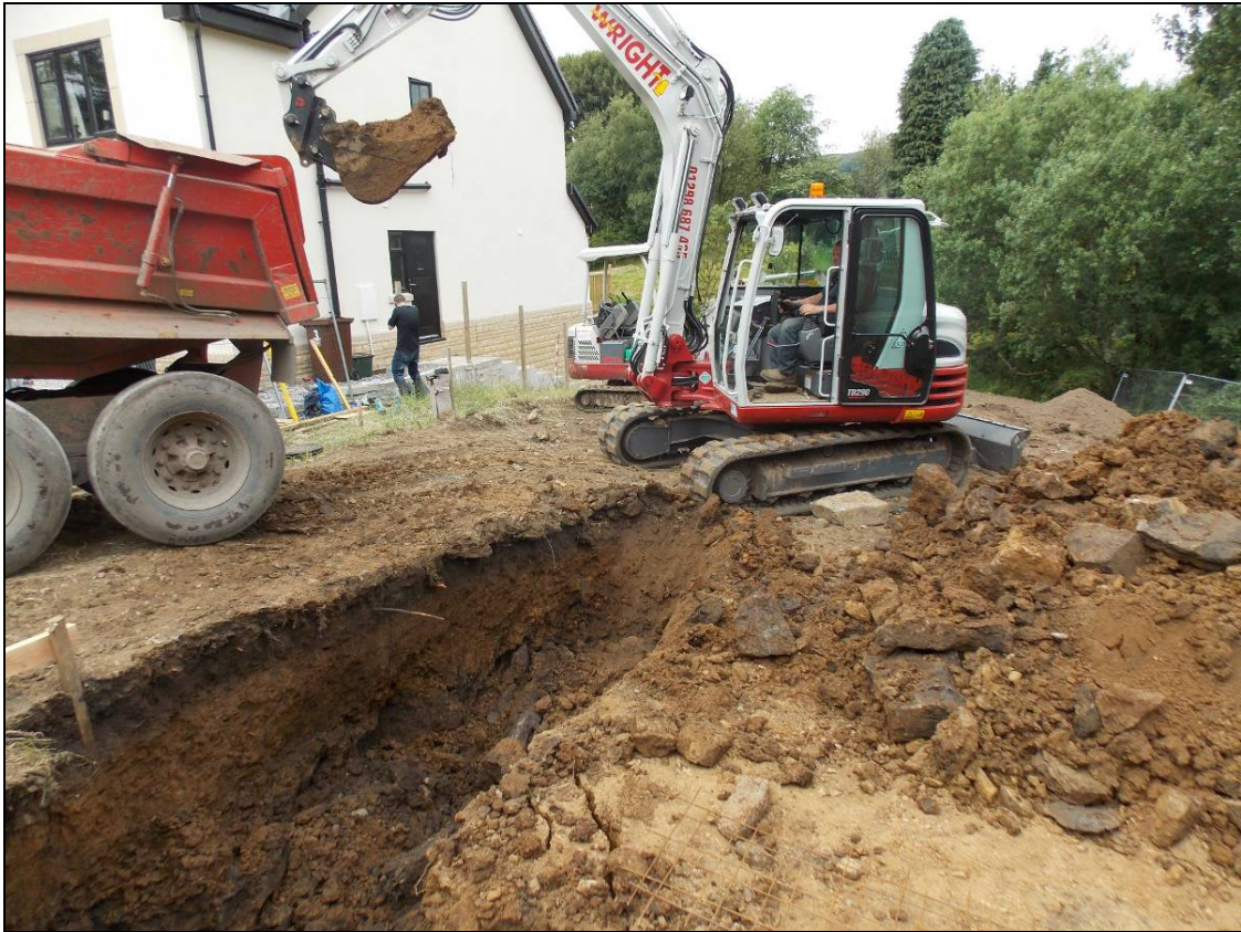
Figure 9: Westernmost trench of Plot 2, looking west.
