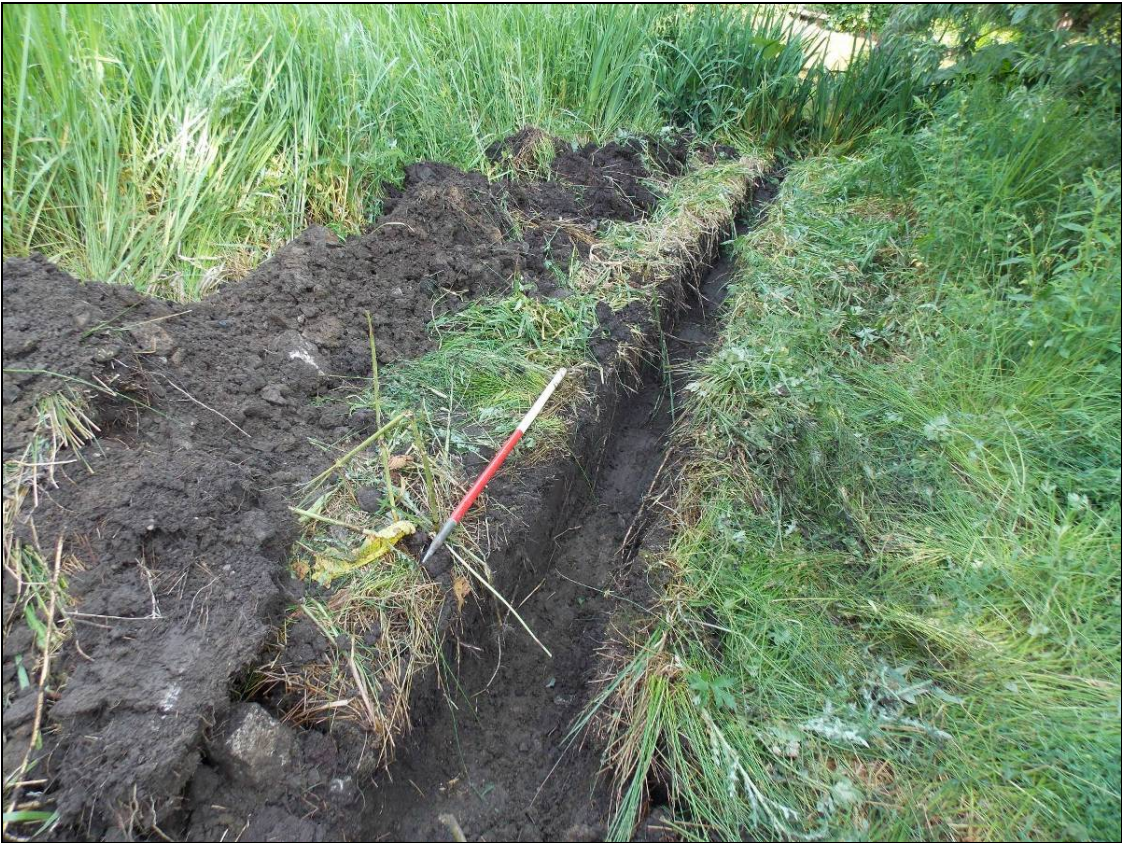
Figure 23: Drainage trench, looking north (scale 1m).
