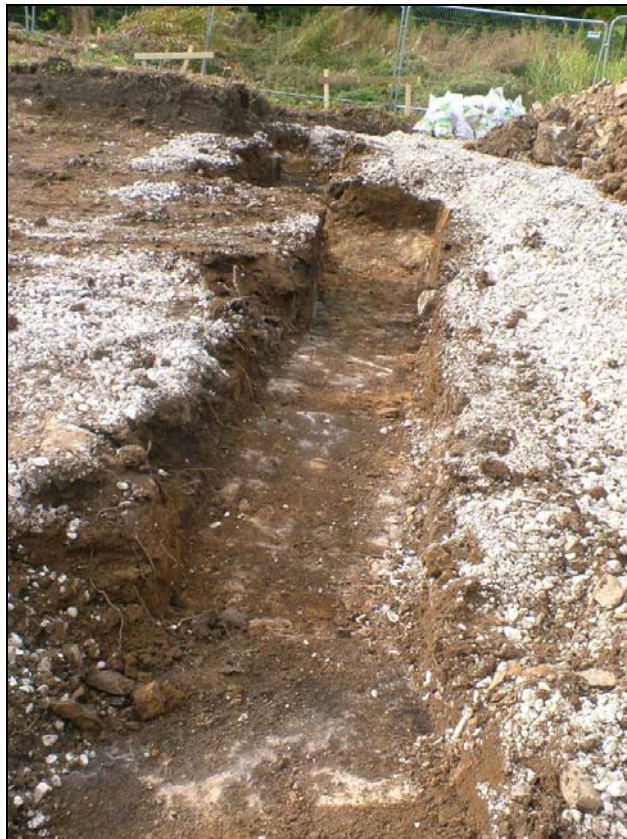
Figure 15: Foundation trench within Plot 3, looking north.
