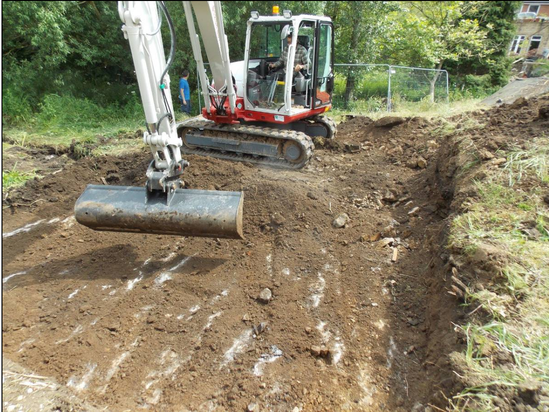
Figure 20: General view of Plot 6 during excavation of the overburden, looking east.
