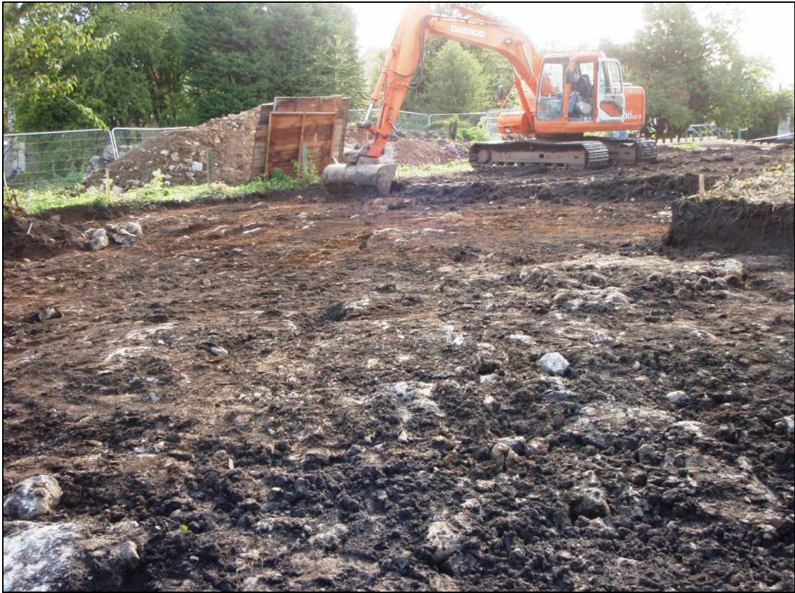
Figure 12: General view of Plot 3 during excavation of the overburden, looking south-east.
