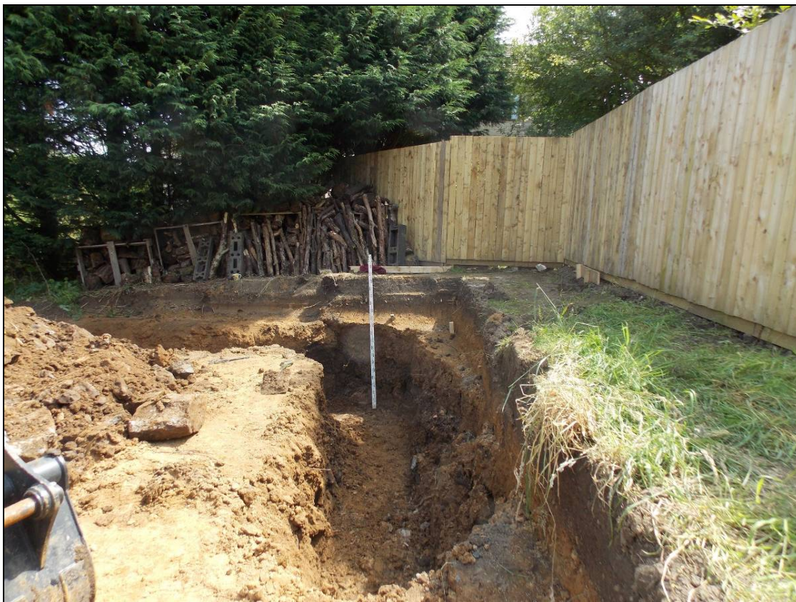
Figure 11: Southernmost trench of Plot 2, looking east (scale 2m).
