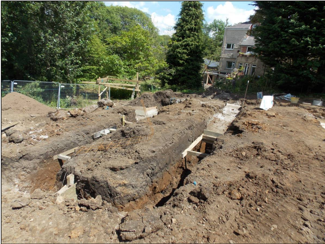
Figure 7: General view of foundation trenches of Plot 2, looking east.
