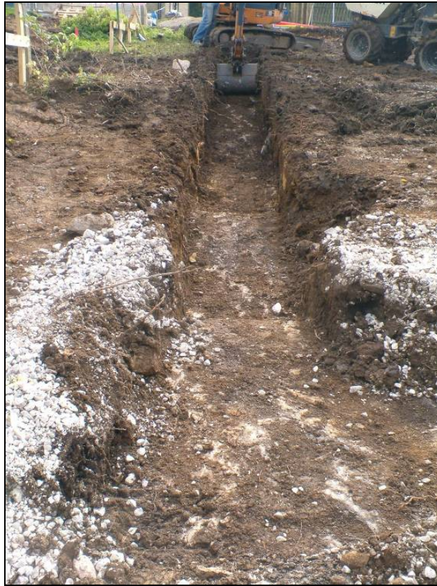
Figure 14: Excavation of foundation trench within Plot 3, looking south.
