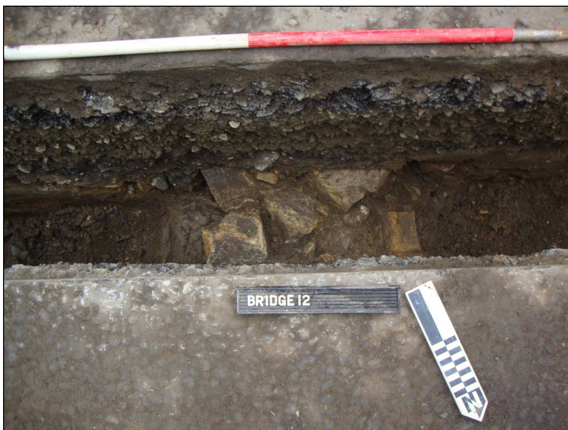
Figure 9. The small section of sandstone wall foundation. Scale = 1m.
