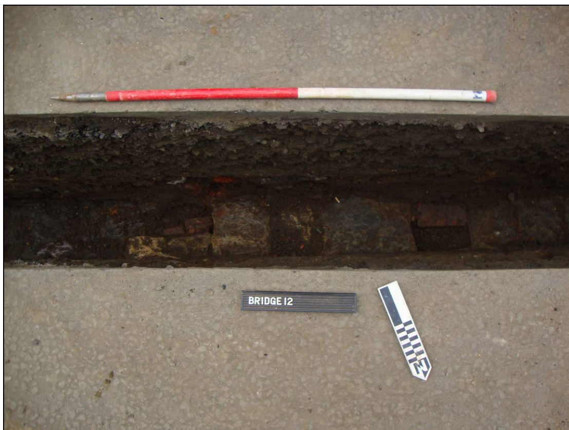
Figure 8. Photograph showing the repair to the drain using bricks. Scale = 1m.
