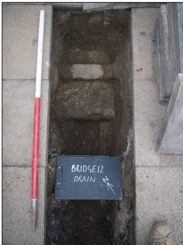
Figure 10. Small offshoot of drain. Scale = 1m.
