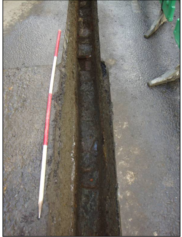
A section of stone and brick lined drain running along the base of the trench on Bridge Street
