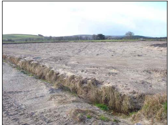
View across the stripped area at Phase D, Cloddach Quarry
