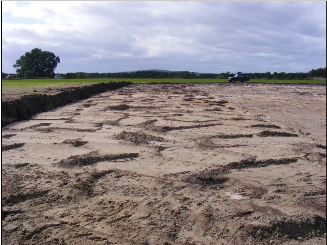
Figure 5: Strip in progress, looking west across the site.
