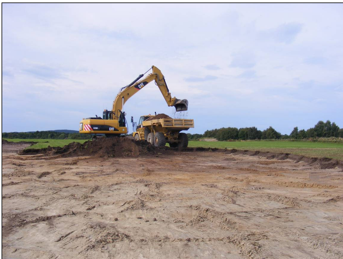
Figure 3: View of strip in progress, looking northwest across the site.
