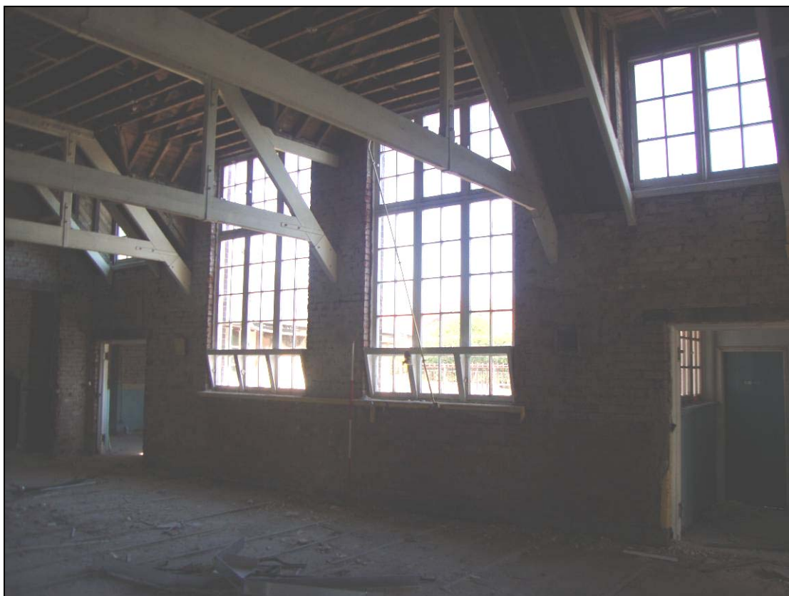
Figure 42: North elevation of Room 4, looking north west. Scale = 2m
