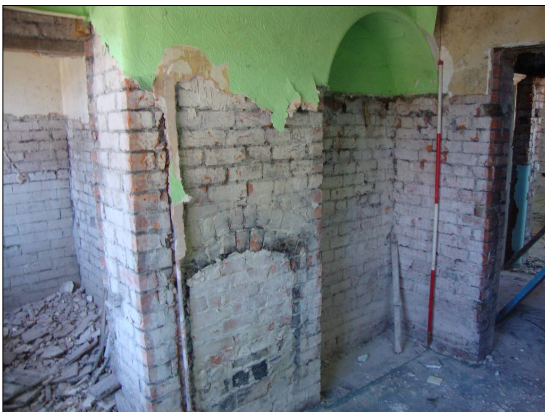
Figure 34: East elevation of Room 2, looking south. Scale = 2m
