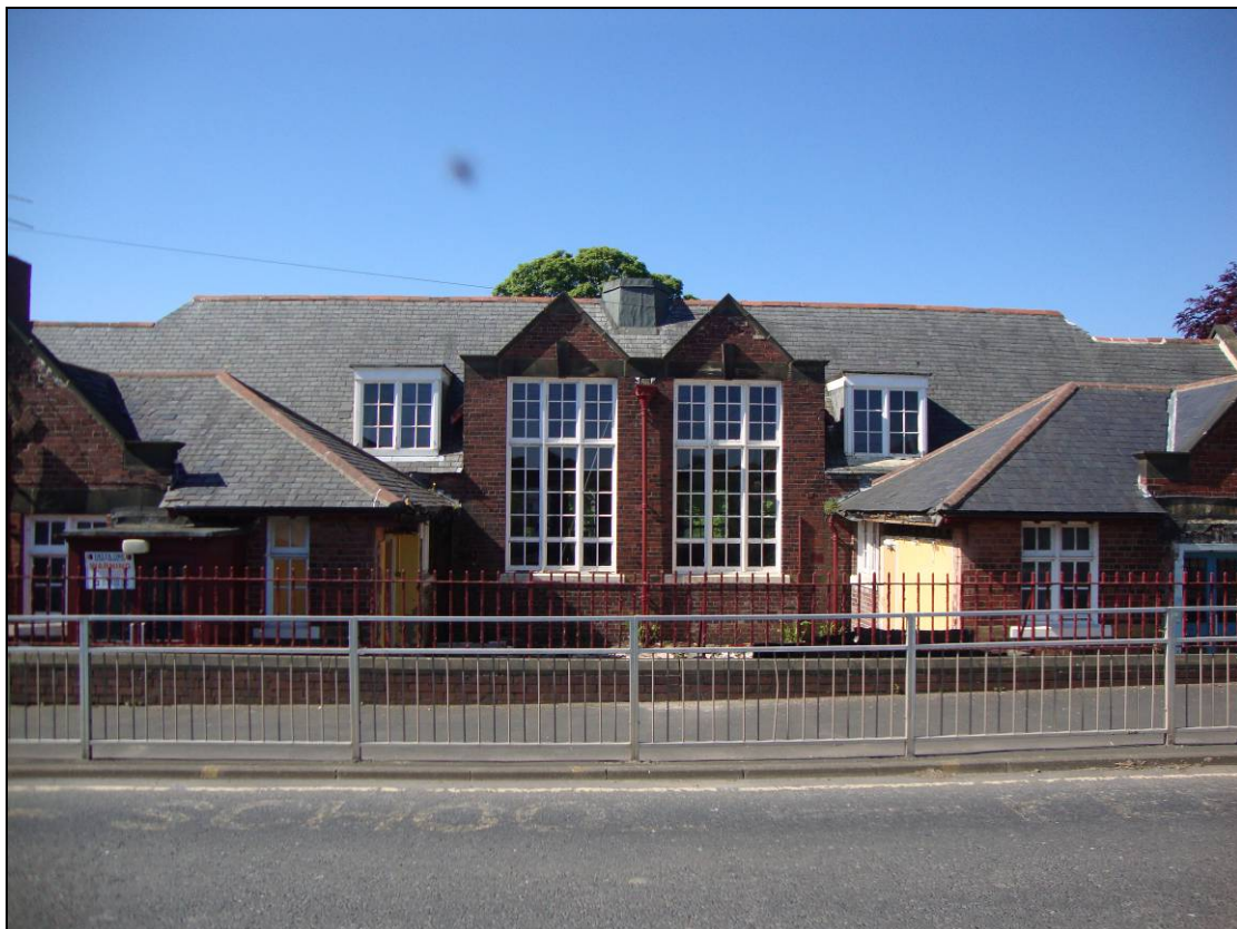
Figure 23: Central section of the north facing elevation, looking south.
