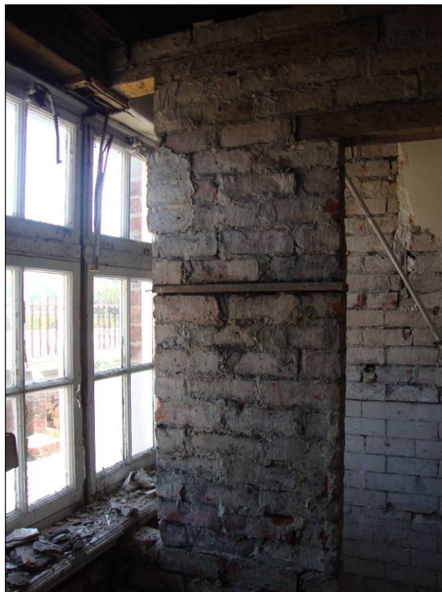
Figure 35: North elevation of Room 2, looking east and showing the detail of the later inserted partition wall.
