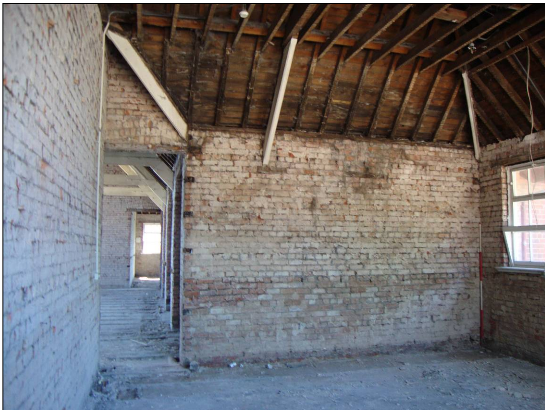
Figure 47: East elevation of Room 6, looking east. Scale = 2m
