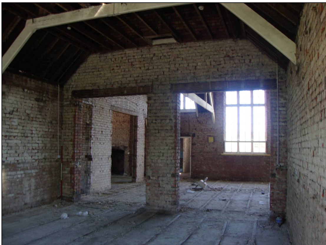
Figure 52: North elevation of Room 7, looking north. Scale = 2m
