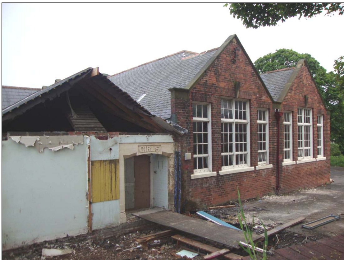
Figure 27: West facing elevation, looking south east.
