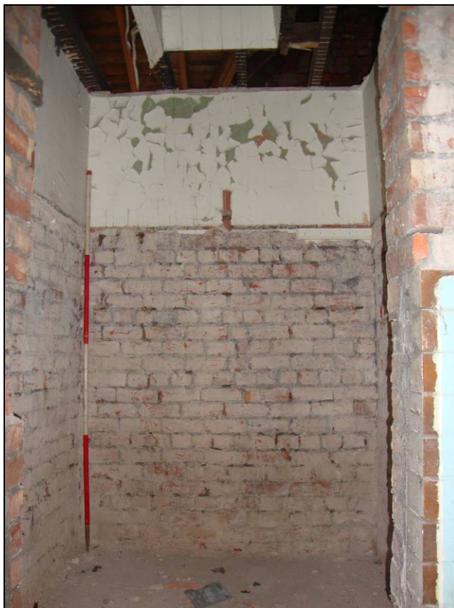
Figure 37: Room 3, looking north. Scale = 2m
