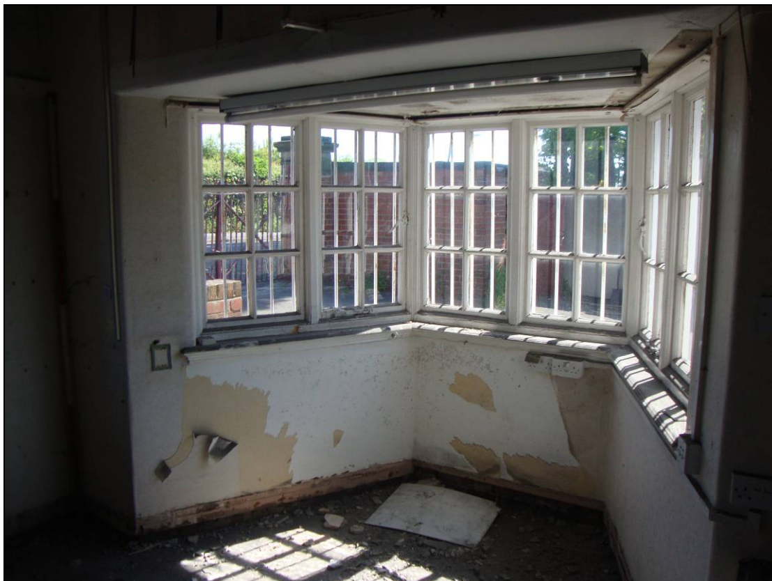
Figure 74: East elevation of Room 13, showing detail of bay window, looking east. Scale = 2m
