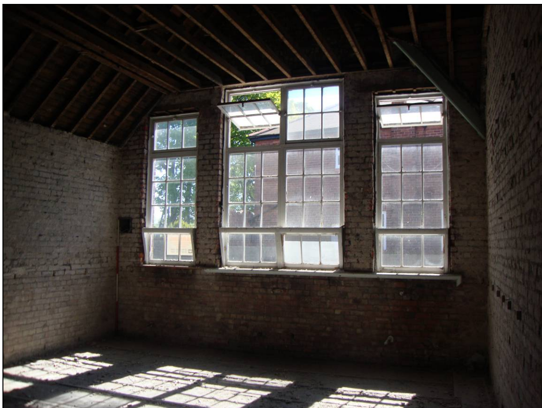
Figure 63: East elevation of Room 10, looking east. Scale = 2m
