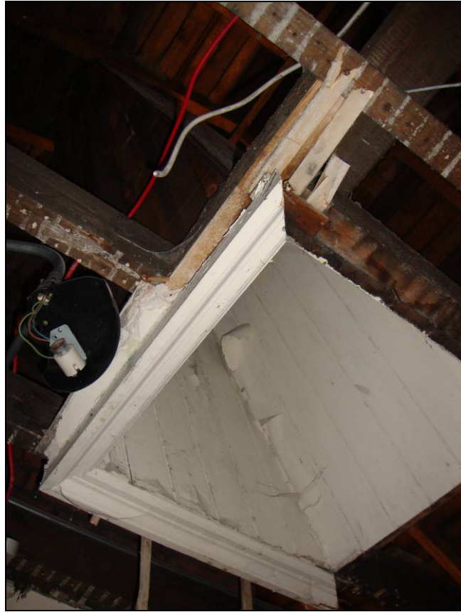
Figure 38: Room 3, ventilation shaft in ceiling.
