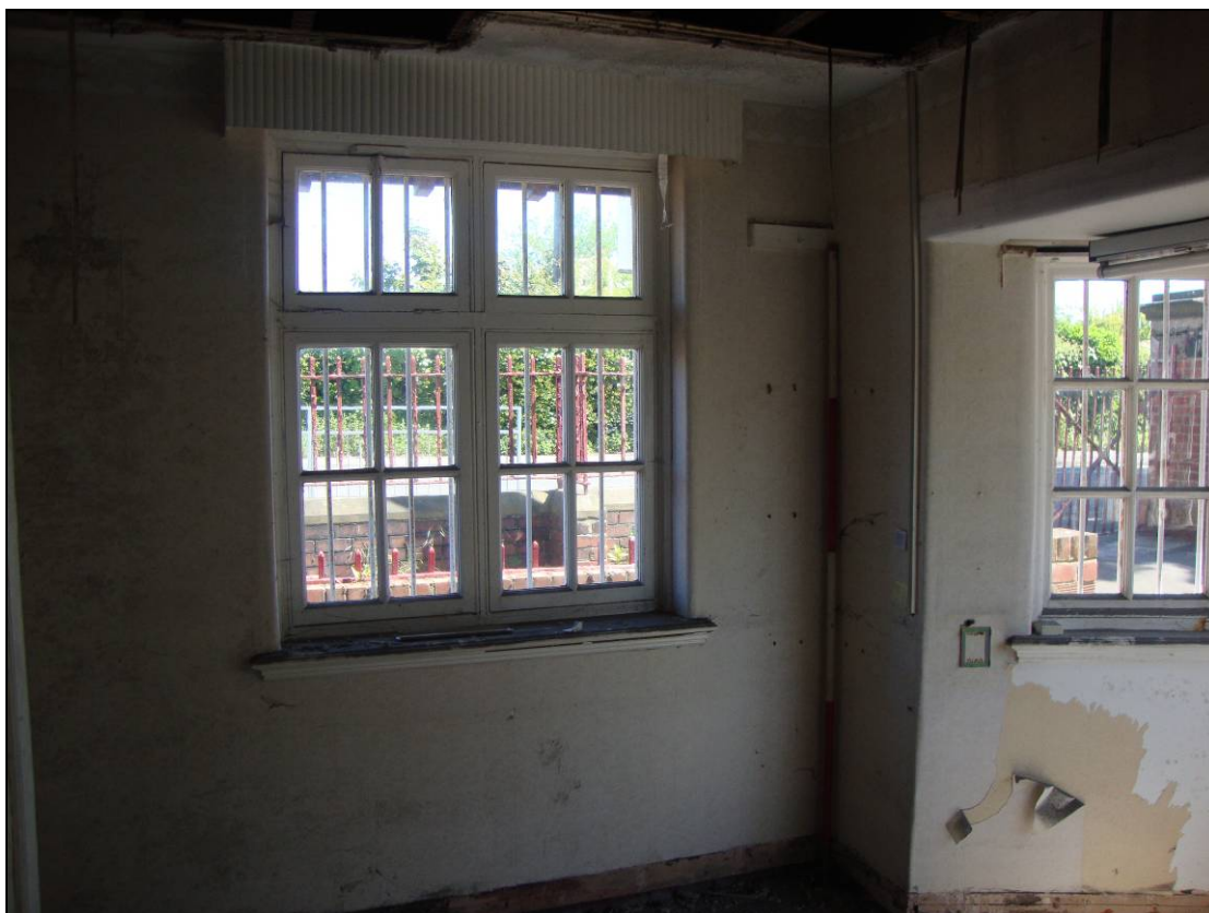
Figure 75: North elevation of Room 13 with window, looking north. Scale = 2m
