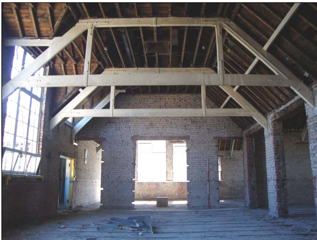
Figure 39: East elevation of Room 4, looking east. Scale = 2m
