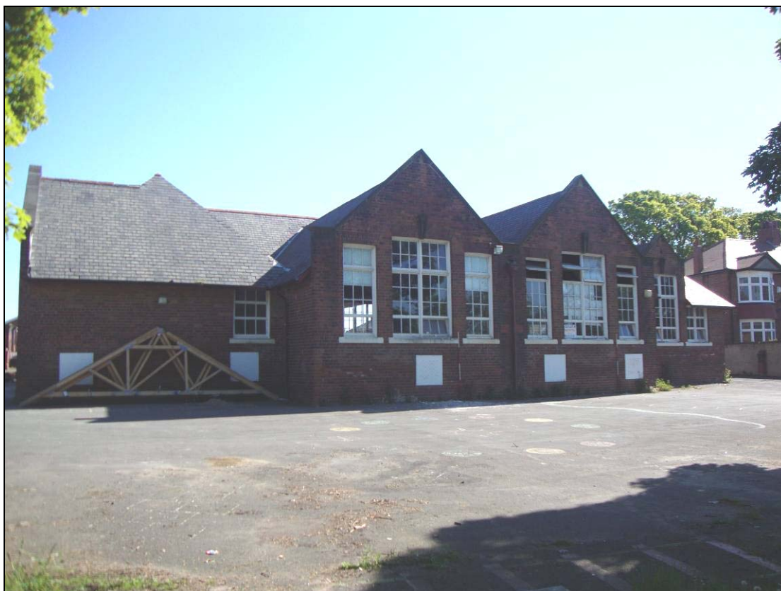
Figure 16: South facing elevation, looking north east. Scale = 2m
