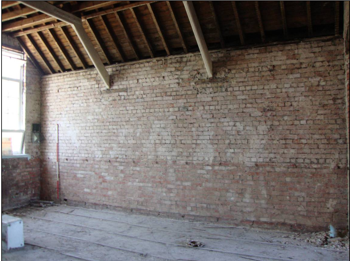
Figure 57: West elevation of Room 8, looking west. Scale = 2m
