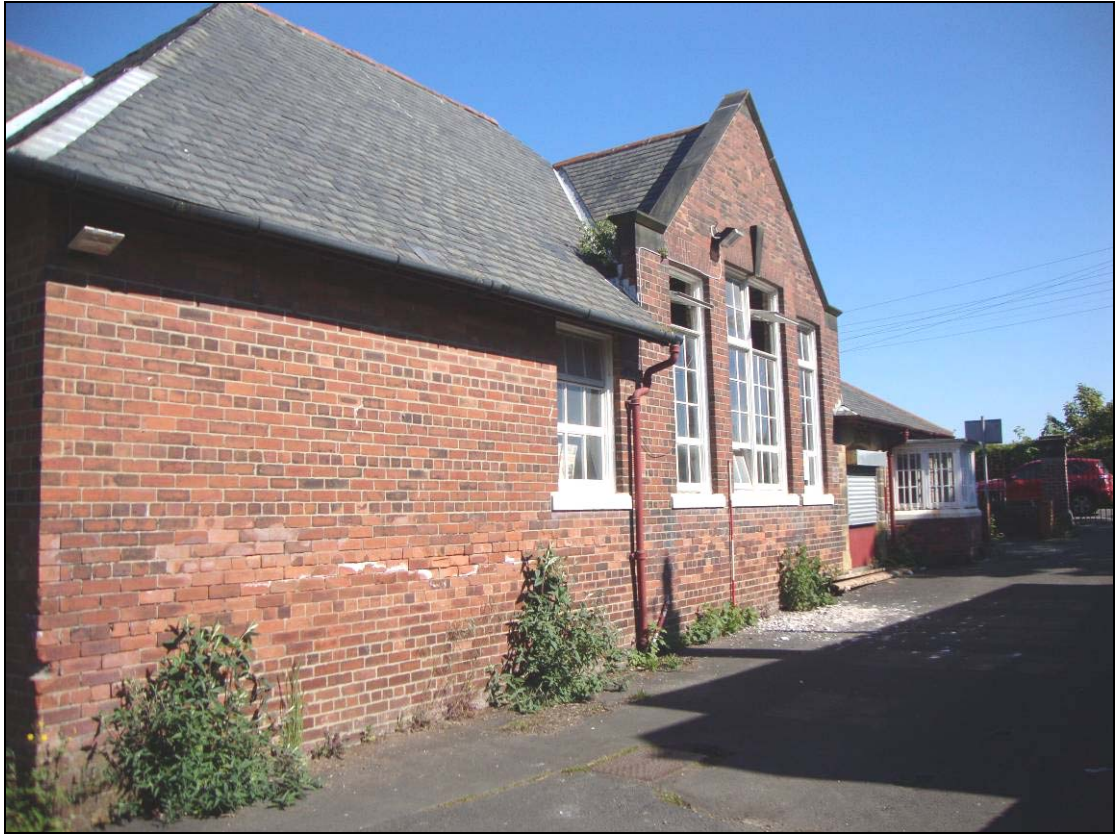
Figure 17: East facing elevation, looking north west. Scale = 2m
