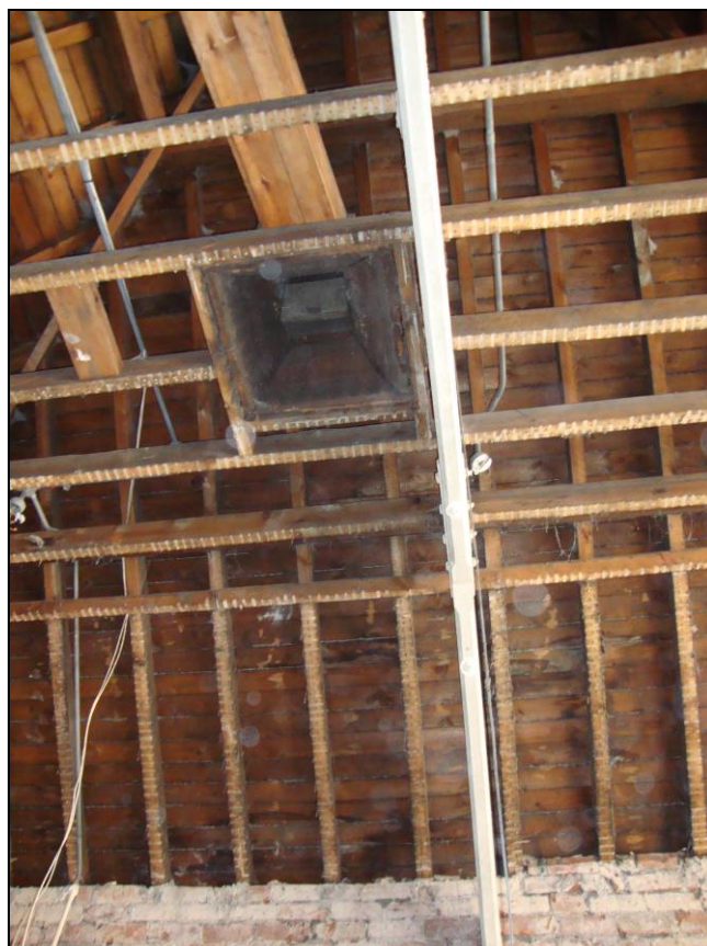
Figure 48: Roof detail of Room 6 with ventilation shaft.
