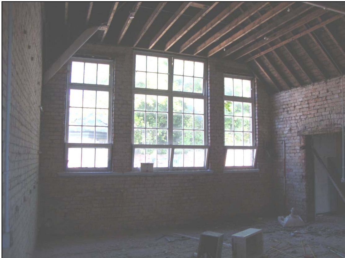
Figure 46: West elevation of Room 5, looking west. Scale = 2m
