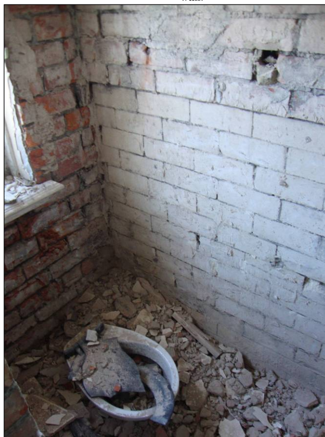
Figure 36: East elevation of Room 2, showing detail of toilet.
