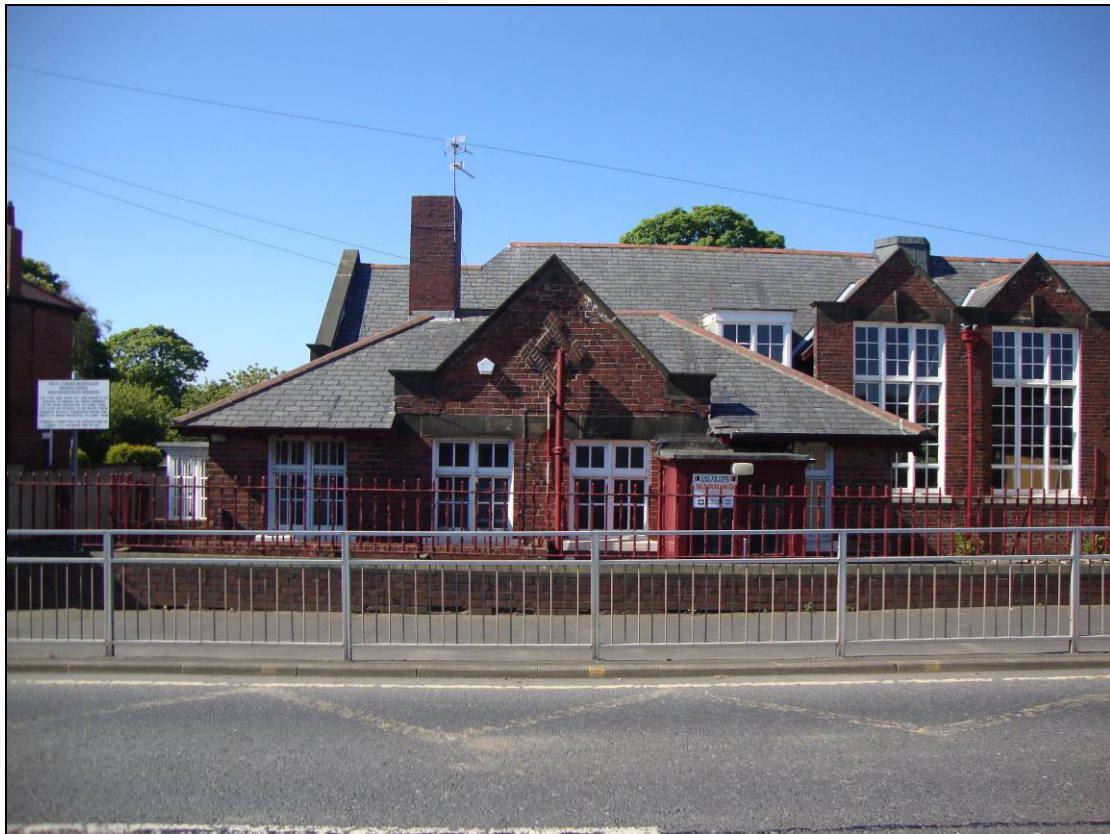
Figure 22: Eastern extent of north facing elevation, looking south. Scale = 2m
