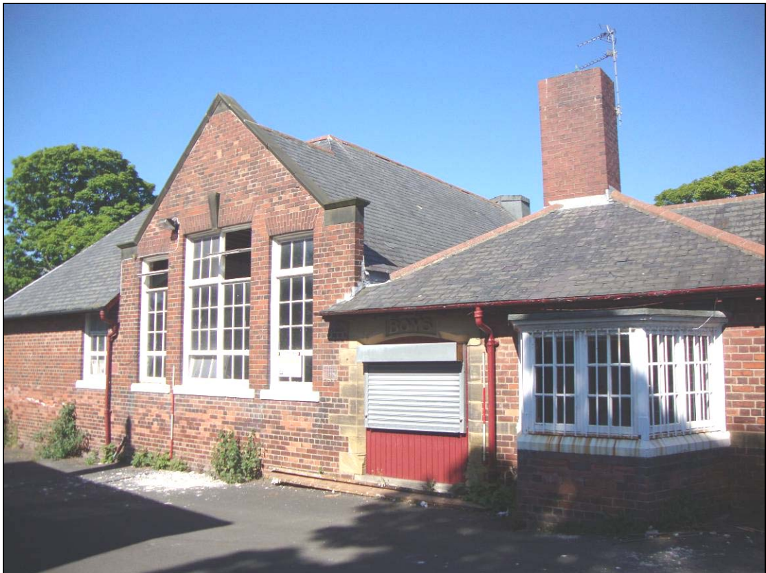
Figure 18: East facing elevation, looking south west. Scale = 2m
