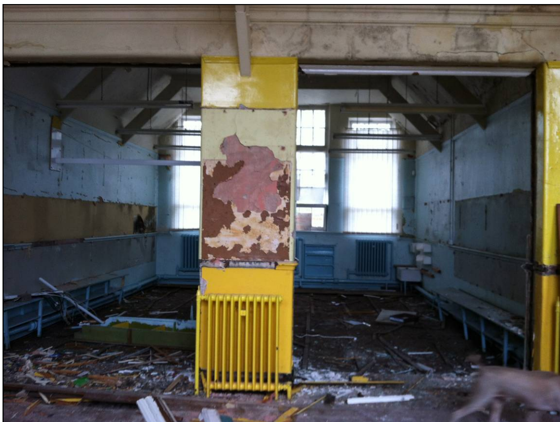
Figure 8: A view into one of the classrooms (Room 8) from the main hall. Note the cast iron radiators below the windows and the benches along the eastern and western walls.
