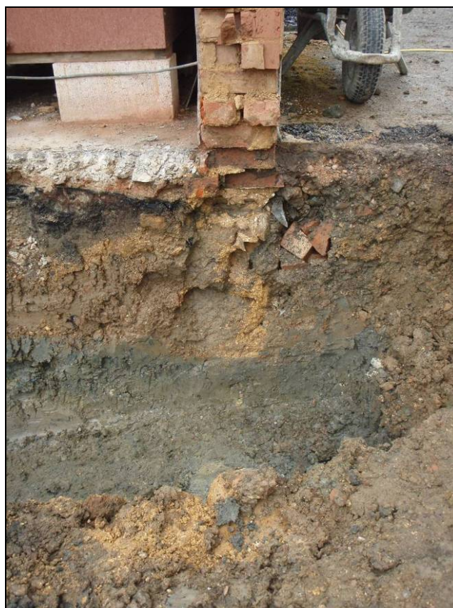
Figure 6: Foundation trench showing the footings of the outbuilding
