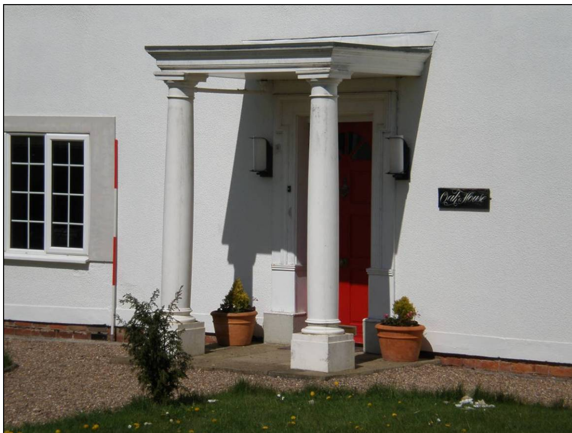
Plate 3: Detail of the porch (scale 2m)
