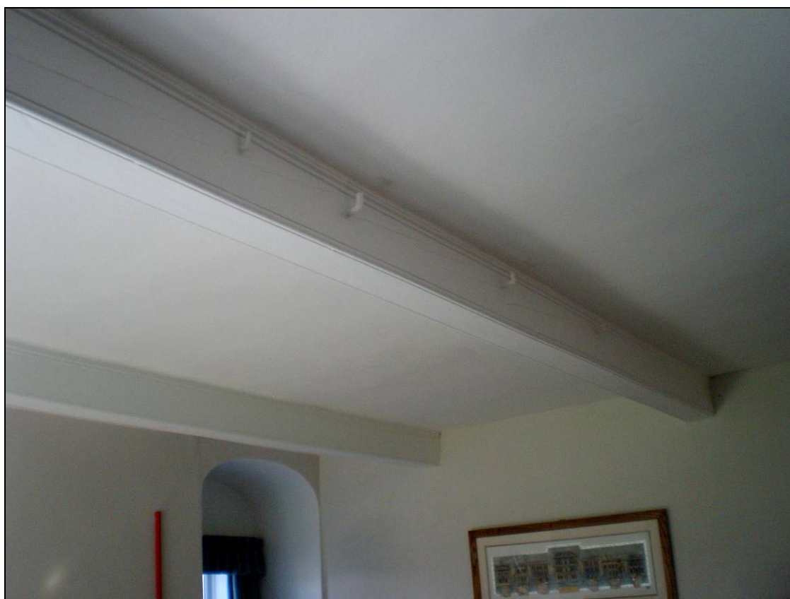
Plate 19: Detail of ceiling beam with iron hooks in room G-3, looking north-west
