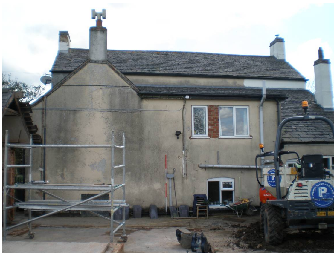
Plate 7: Eastern side of the north elevation (scale 2m)
