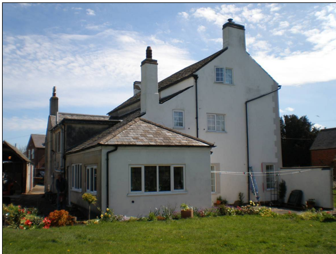
Plate 12: General view of the west elevation (scale 2m)
