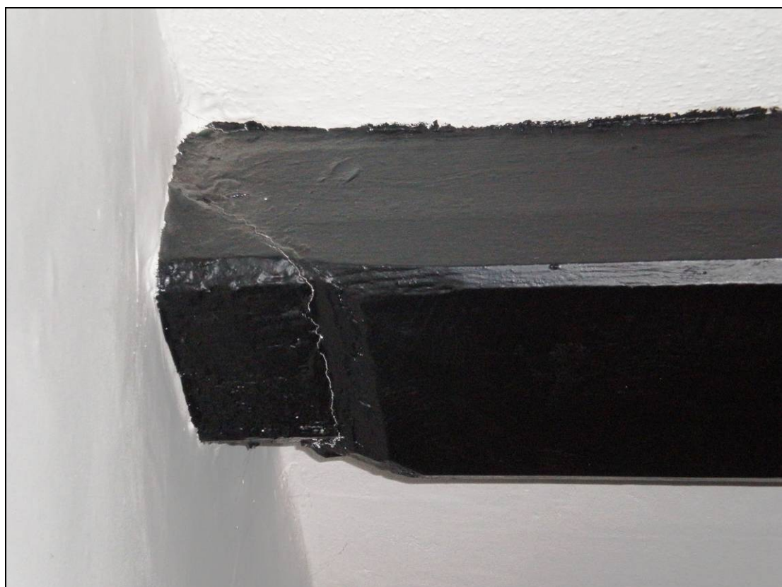
Plate 42: Scarf joint along the side purlins in room S-3
