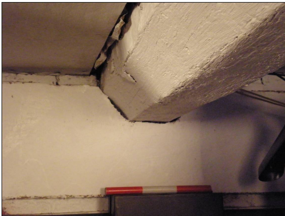
Plate 23: Detail of ceiling beam in room G-5, looking west (scale 300mm)
