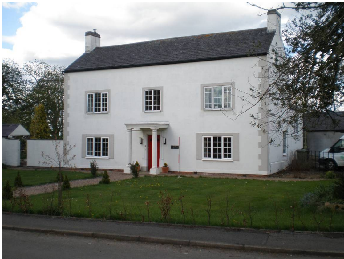
Plate 1: General view of the front south elevation (scale 2m)
