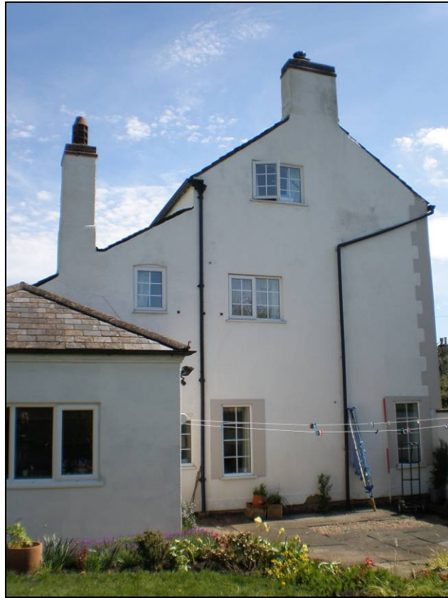
Plate 13: Detail of the gable side (scale 2m)
