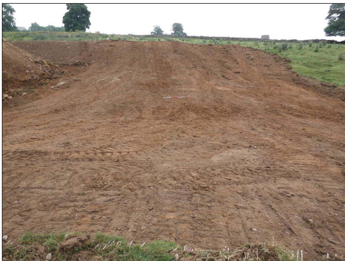
Figure 7. Phase 2b completed strip area
