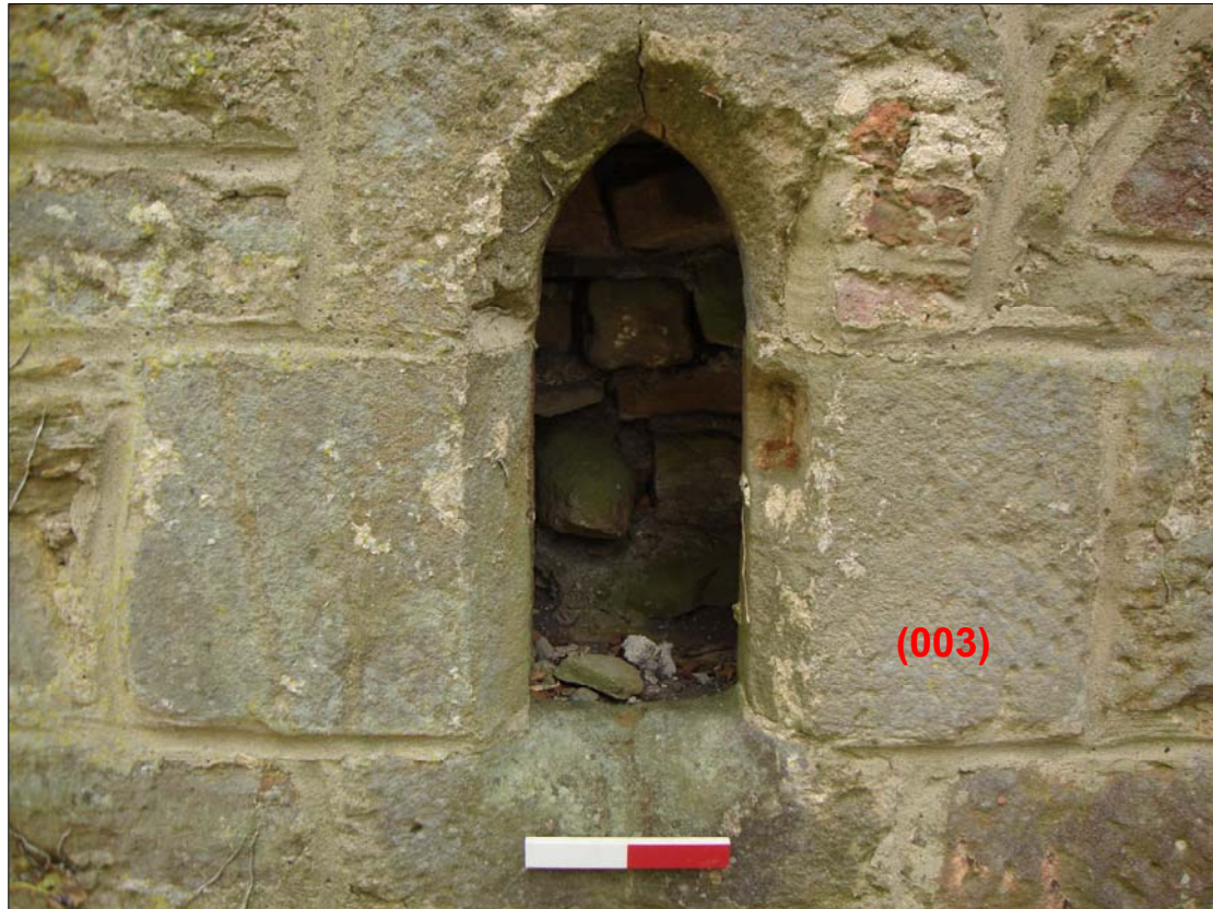
Figure 5. Original 15 th century window (003) blocked by the insertion of the brick skin wall and fireplace (001), looking south (scale = 0.2m)
