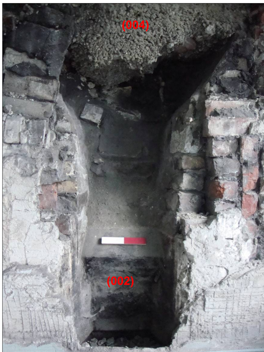
Figure 4. Profile of the brick infill and inserted small fireplace (002), looking north (scale = 0.2m)
