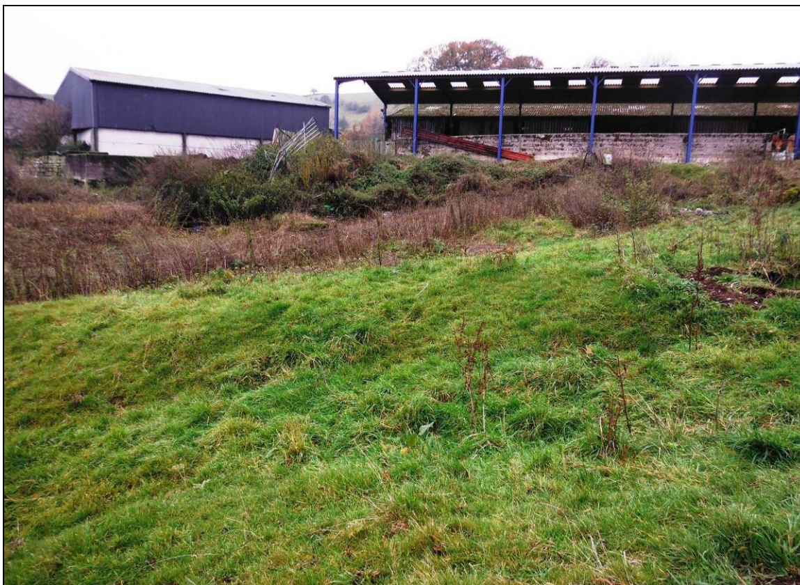
Figure 13: The large disturbed area within the western side, looking south-west
