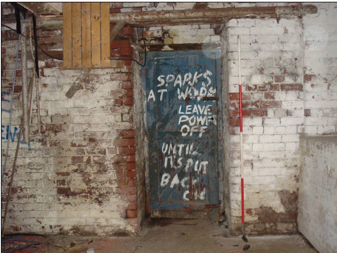
Figure 53: Doorway to the electrical switchboard room, looking south (scale 2m)
