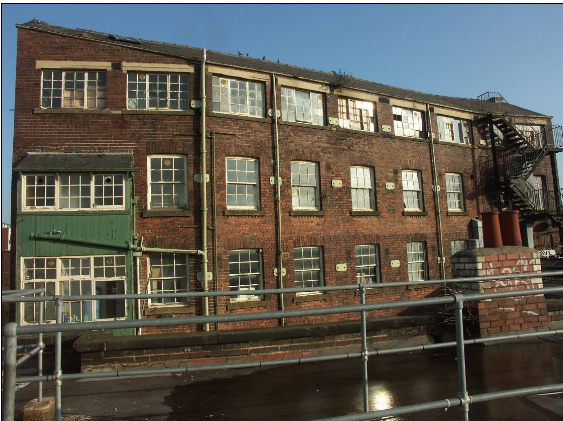
Figure 41: South elevation of Building 2, looking north
