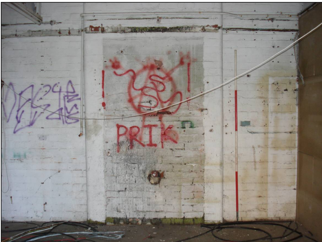
Figure 29: Blocked-up fire place within the northernmost room of the eastern wing, looking east (scale 2m)
