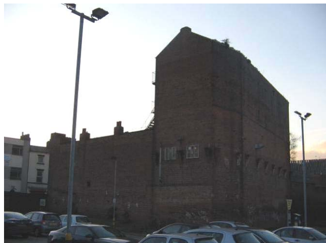
The extant buildings on the site looking south-east
