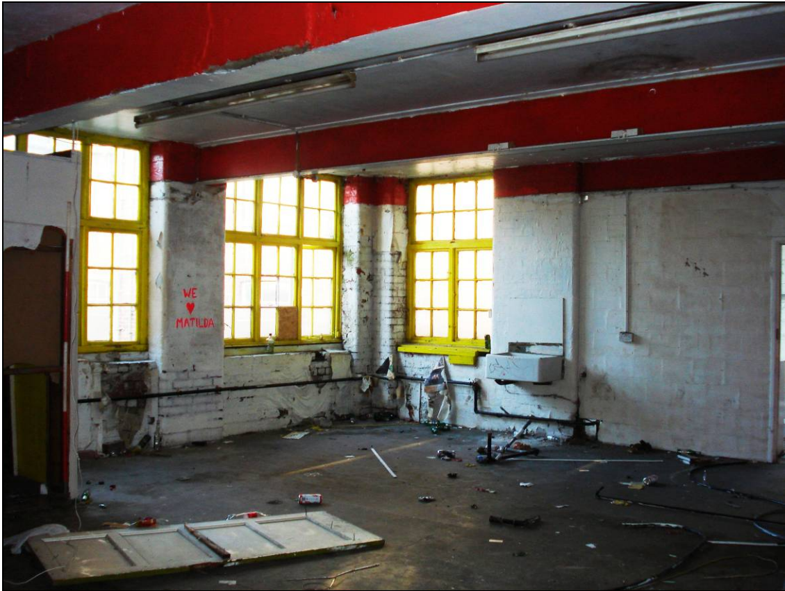
Figure 35: Main room of the eastern wing, looking north-west (scale 2m)
