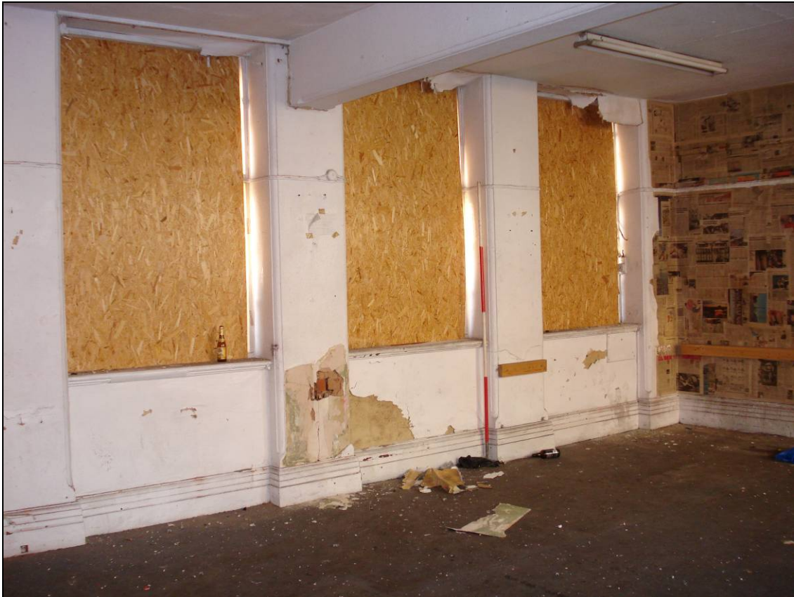
Figure 31: First floor of the southern wing, looking west (scale 2m)
