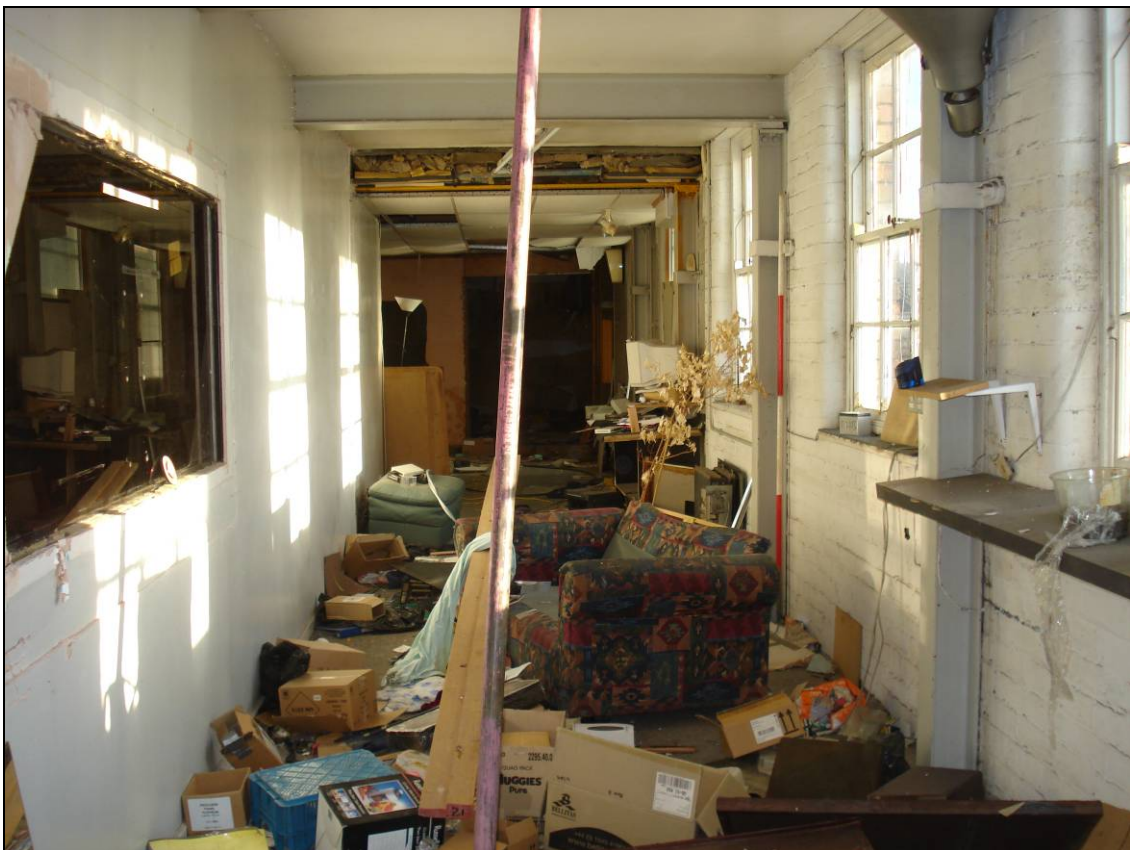
Figure 64: General view of the second floor, looking west (scale 2m)
