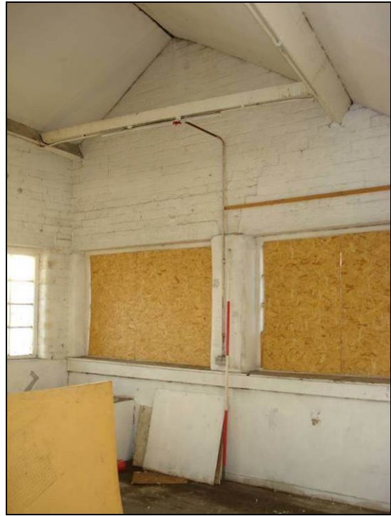
Figure 74: West gabled end (scale 2m)
