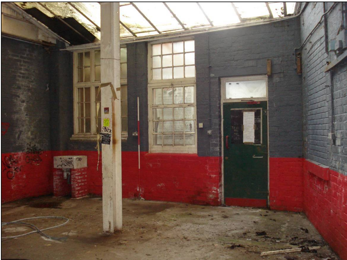
Figure 22: Northern room of the eastern wing, looking west (scale 2m)
