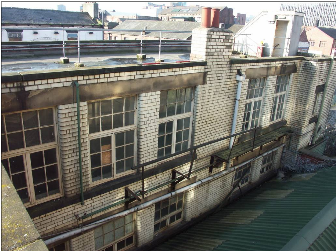
Figure 11: North elevation of Building 1, looking south-west (scale 2m)
