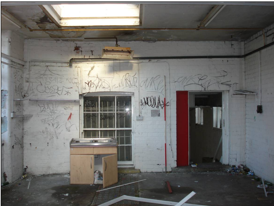
Figure 38: The northern end of the eastern wing leading to the adjoining Building 2, looking north (scale 2m)
