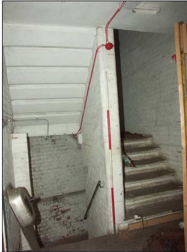
Figure 63: Staircase to the upper floor (scale 2m)
