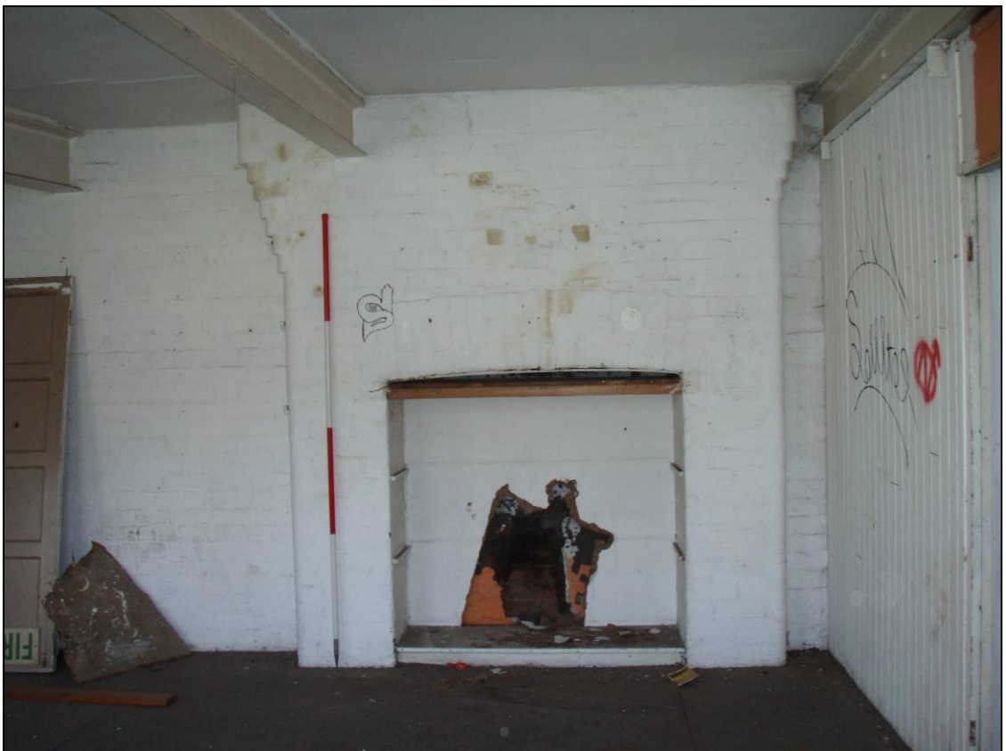
Figure 61: Former fire place within the western area of the first floor, looking north (scale 2m)
