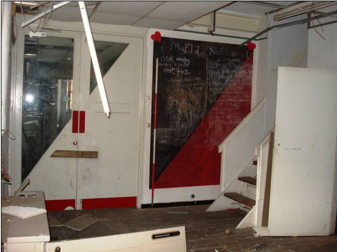
Figure 55: Detail of stud partition and quarter-turn staircase, looking west (scale 2m)
