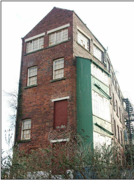
Figure 48: West elevation of Building 2
