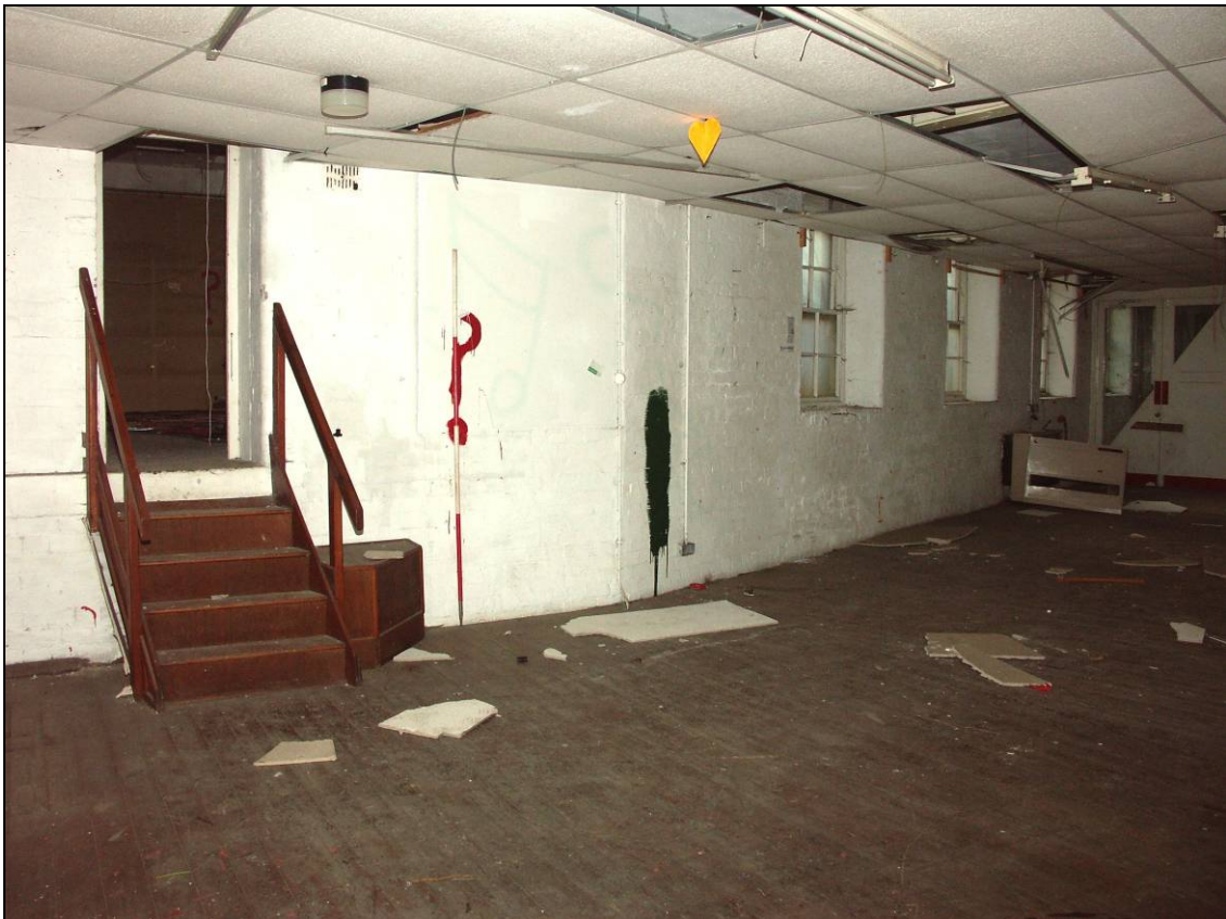
Figure 54: Ground floor of Building 2, looking west (scale 2m)
