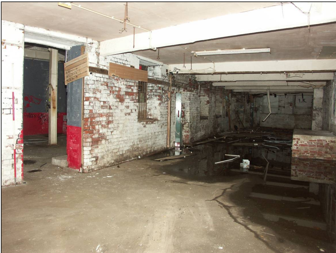
Figure 51: General view of the basement, looking west (scale 2m)
