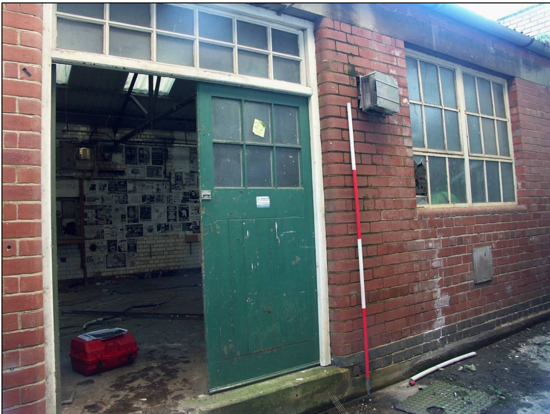
Figure 81: Main doorway within the north elevation (scale 2m)
