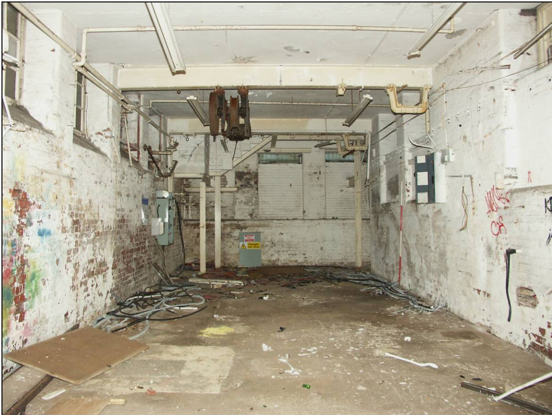
Figure 16: Basement within the southern wing, looking west (scale 2m)
