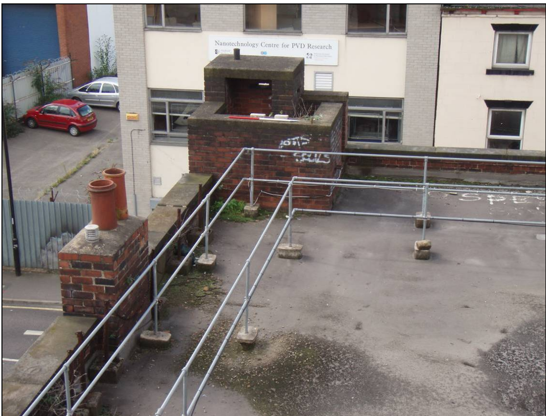
Figure 13: Flat roof with inserted brick-built pillbox, looking south (scale 1m)
