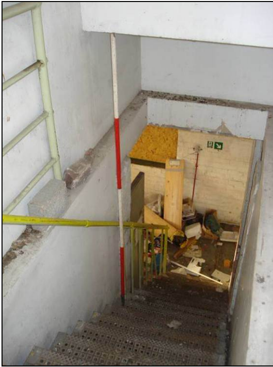
Figure 73: Staircase to the fourth floor (scale 2m)
