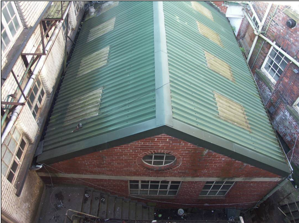
Figure 80: Aerial view of Building 3, looking west
