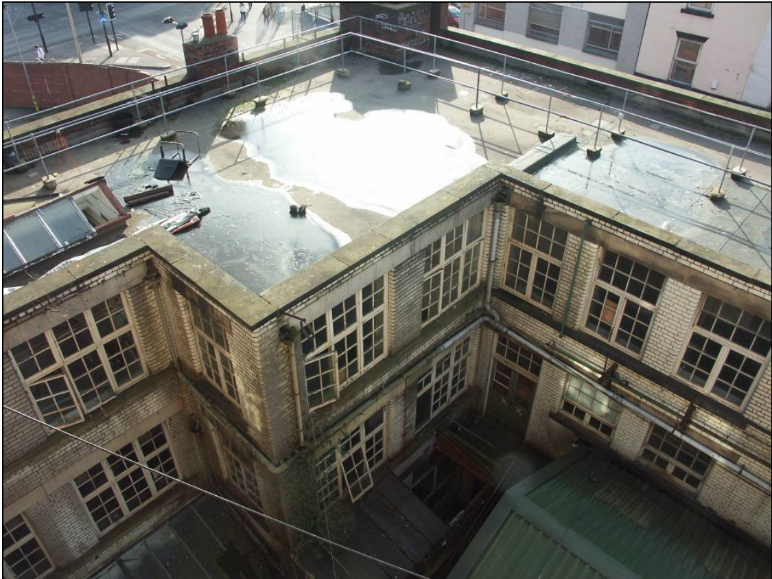
Figure 12: General view of the flat roof of Building 1, looking south-east
