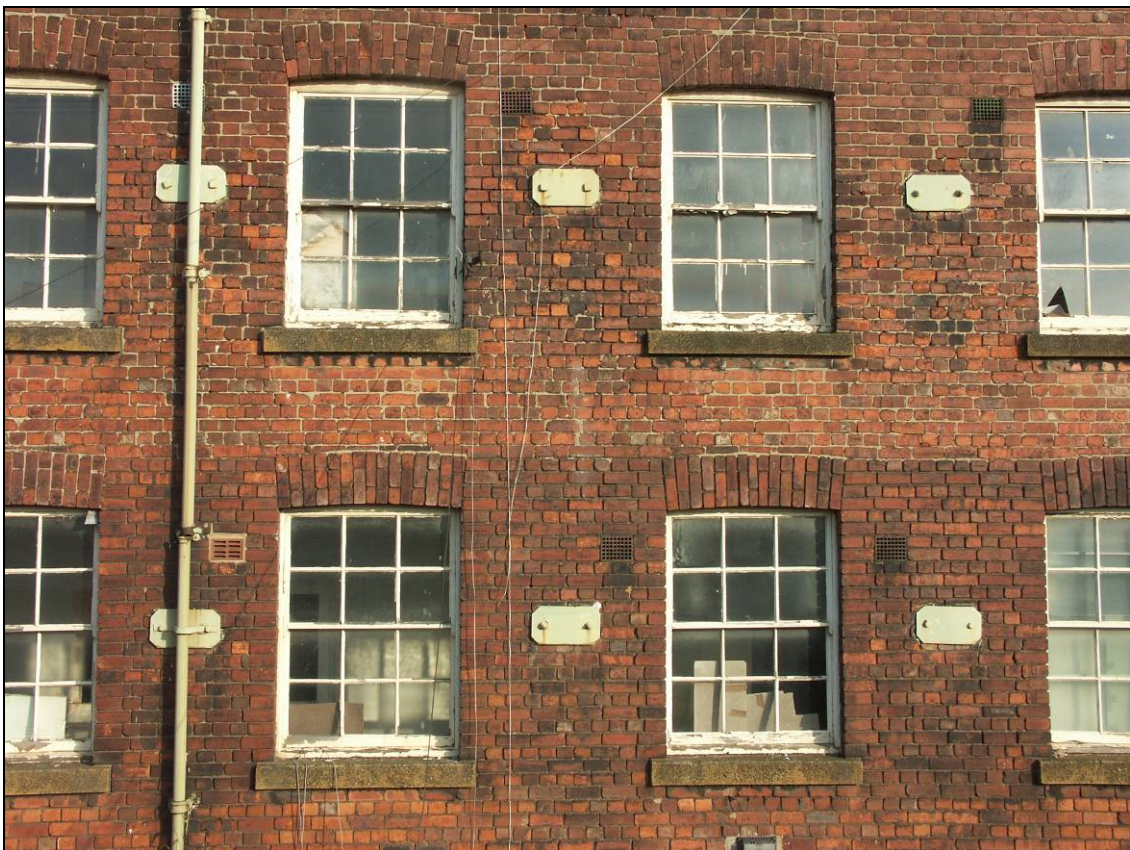
Figure 43: Detail of fenestration within the south elevation
