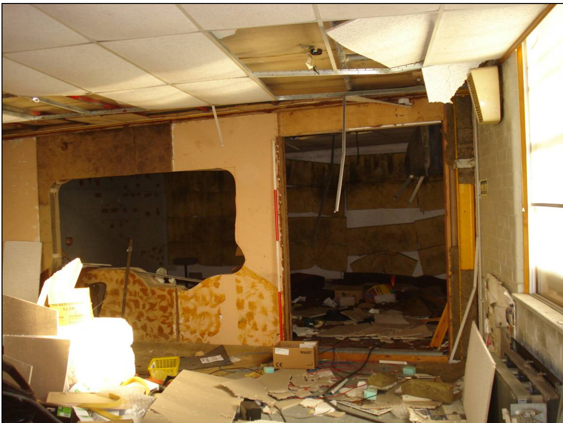
Figure 66: Eastern area of the second floor, looking east (scale 2m)
