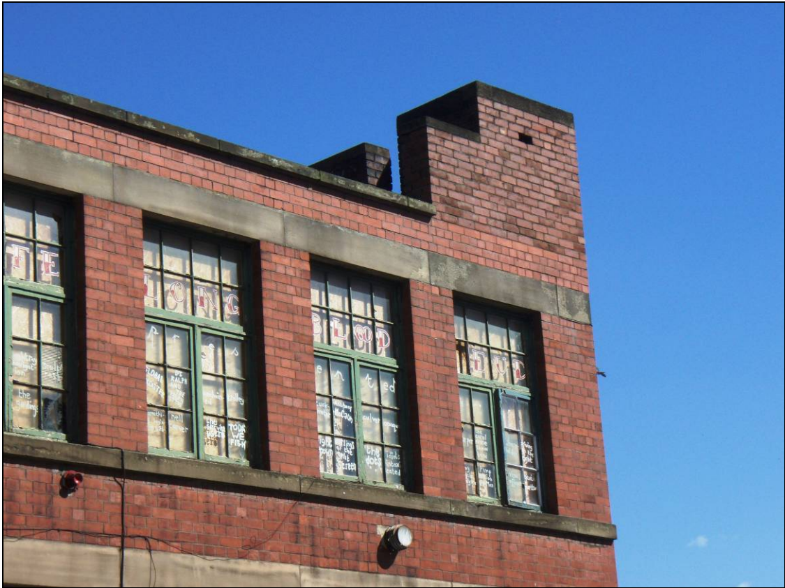
Figure 4: Detail of inserted pillbox over the roof, looking north-east
