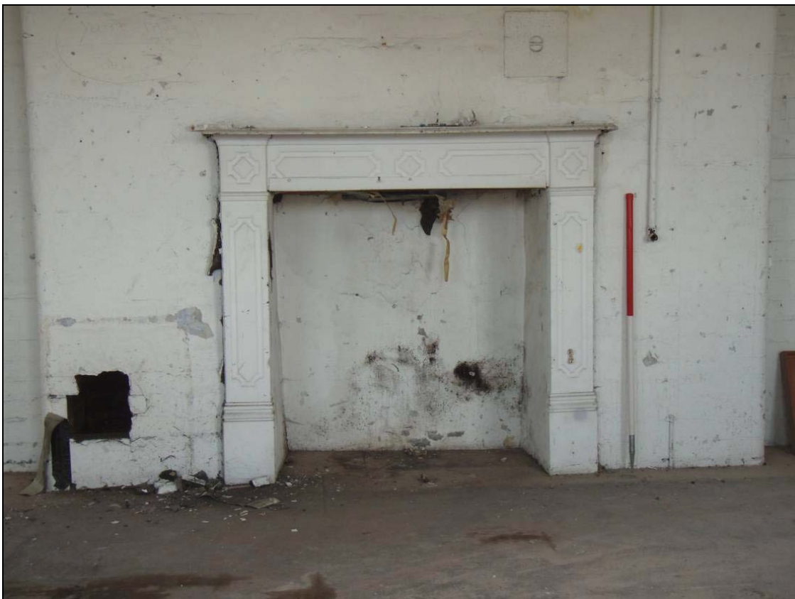
Figure 69: Detail of fire place, looking north (scale 1m)
