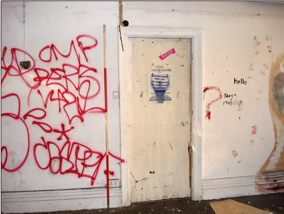
Figure 33: Detail of architrave and moulded skirting boards within the first floor of the southern wing
