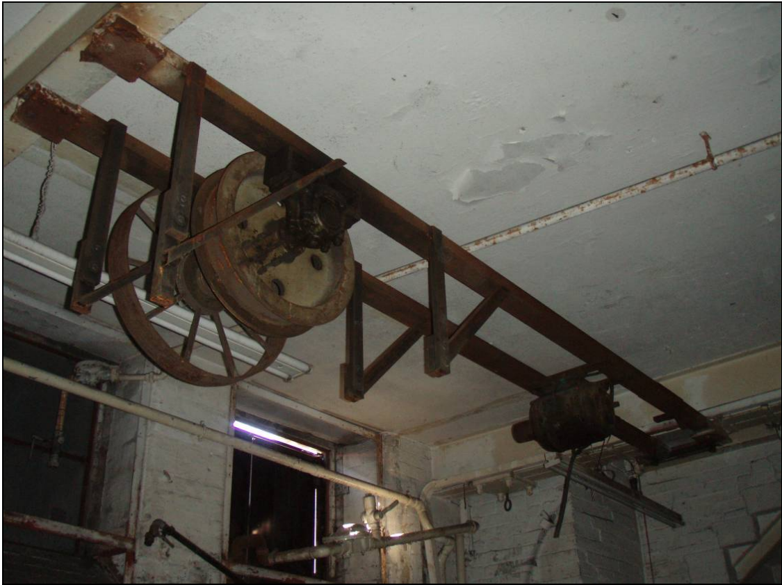
Figure 17: Detail of former motor, drive belt and flywheel, looking east
