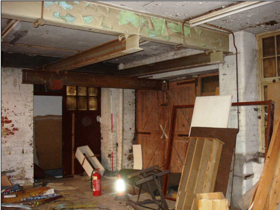
Figure 26: Loading bay with gantry above floor hatch, looking east (scale 2m)
