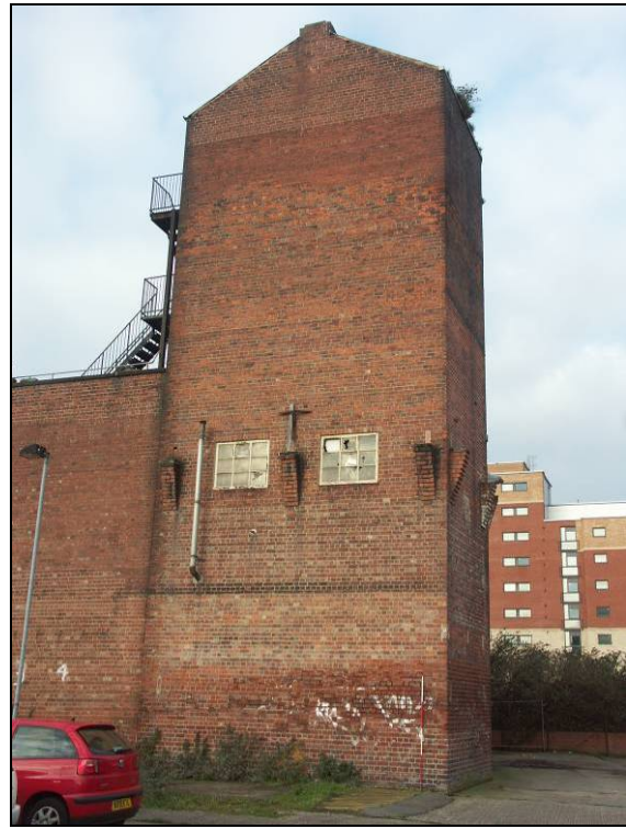
Figure 49: East elevation of Building 2 (scale 2m)
