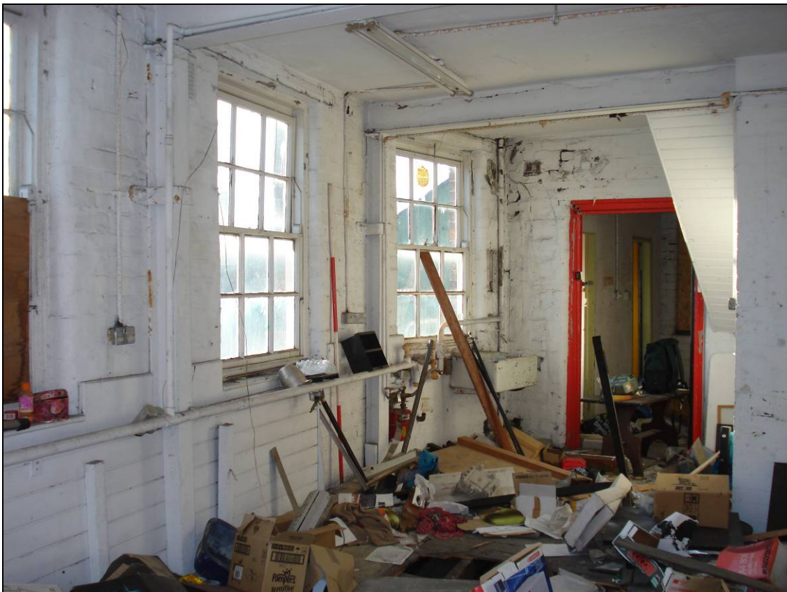
Figure 67: General view of the third floor, looking west (scale 2m)
