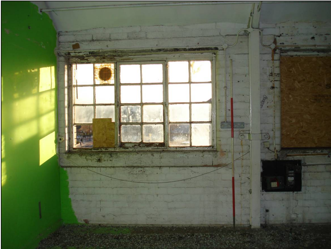
Figure 76: Detail of RSJ stanchion, looking south (scale 2m)
