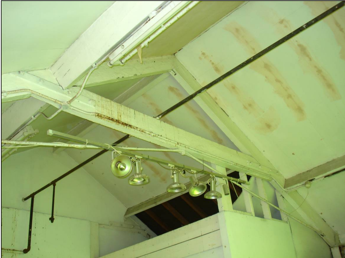
Figure 75: Detail of roof truss, looking west
