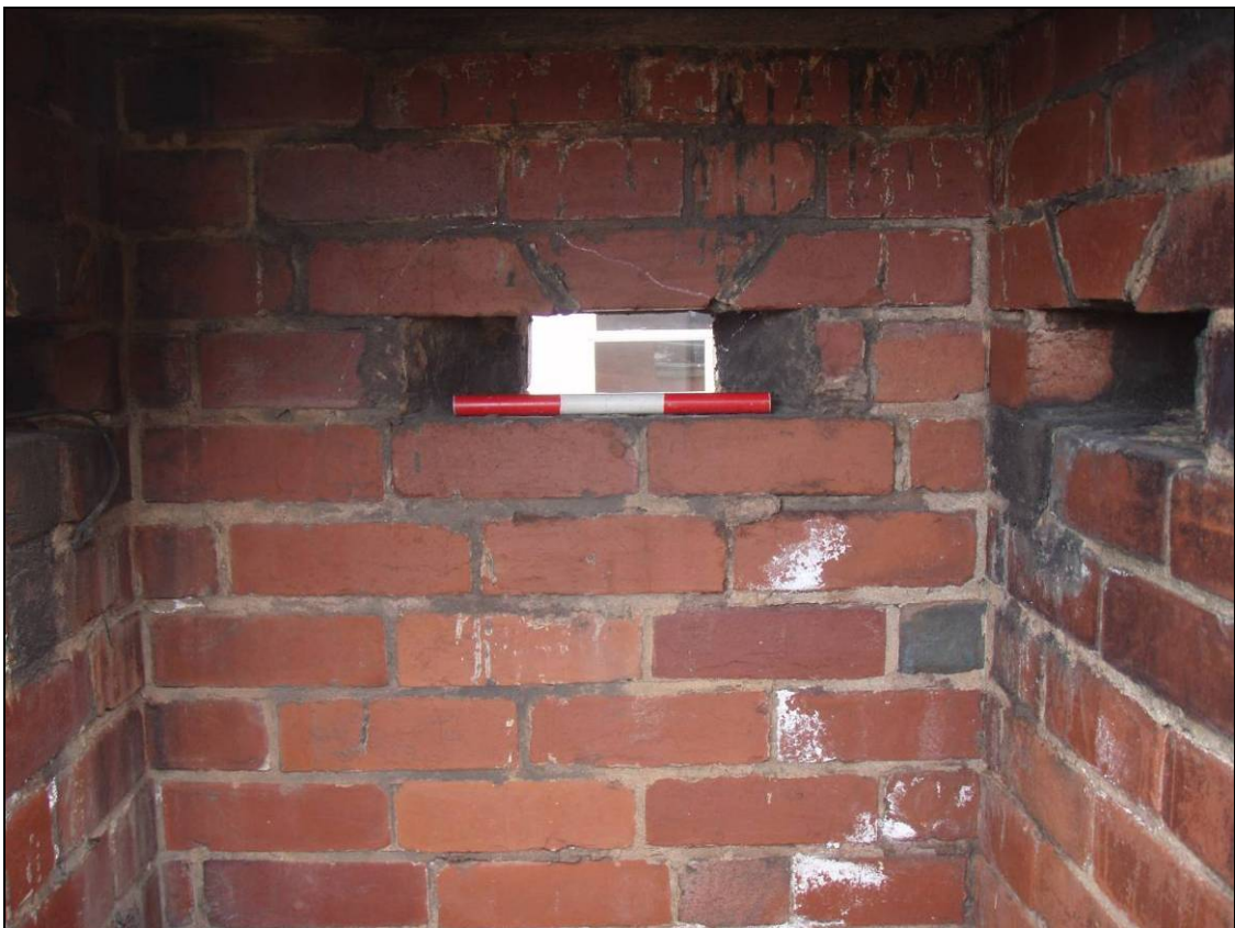
Figure 15: Detail of splayed aperture at eye level, looking south-west (scale 300mm)
