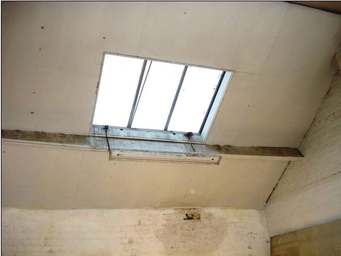
Figure 79: Skylight along the northern angled ceiling
