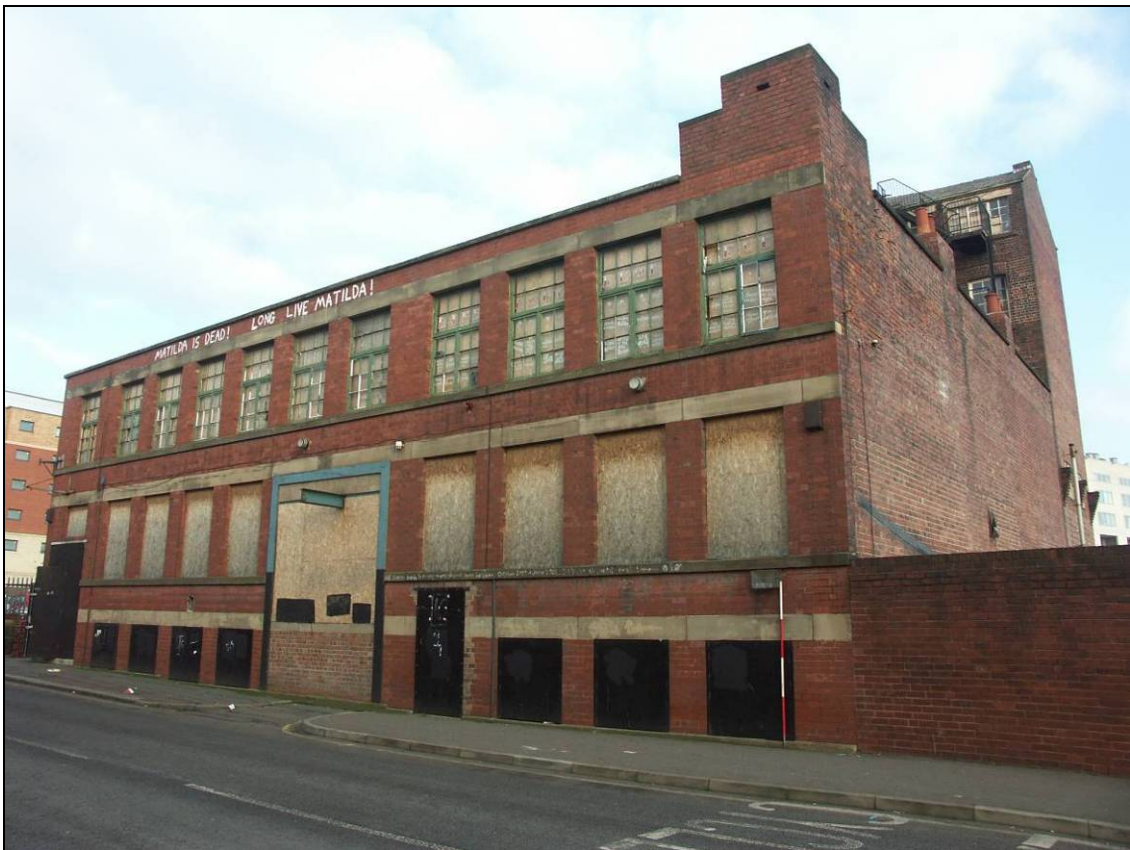
Figure 3: South elevation of Building 1 along Matilda Street, looking north-west (scale 2m)
