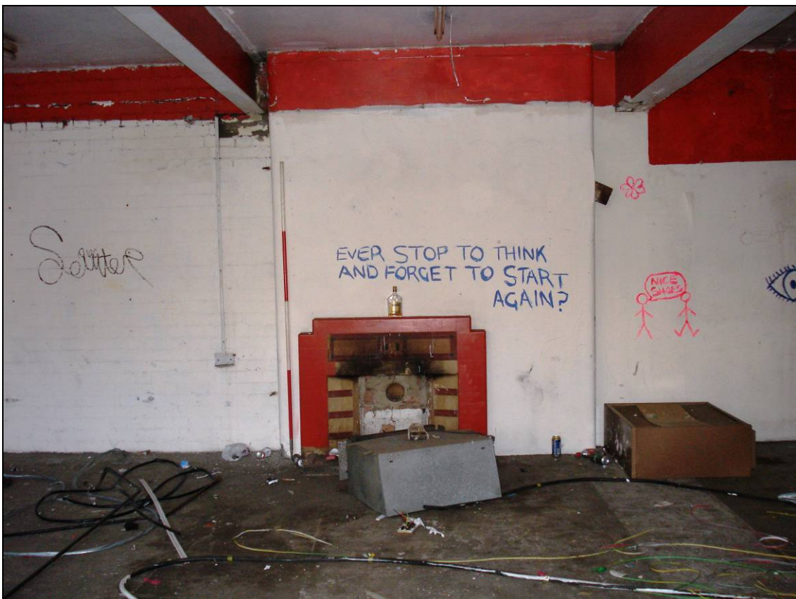
Figure 36: Fire place within the central room of the eastern wing, looking east (scale 2m)
