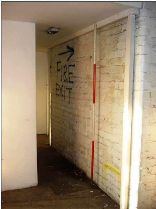
Figure 77: Bricked-up fire place (scale 2m)
