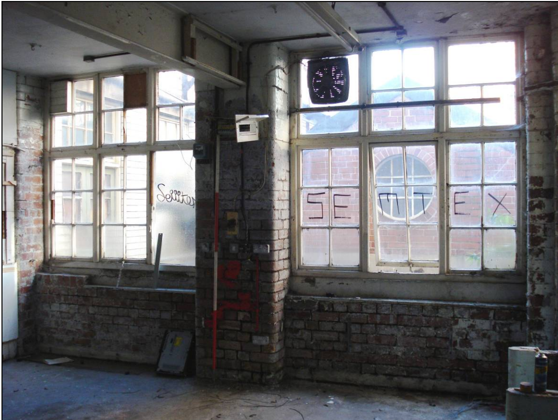
Figure 28: Eastern wing, looking west (scale 2m)
