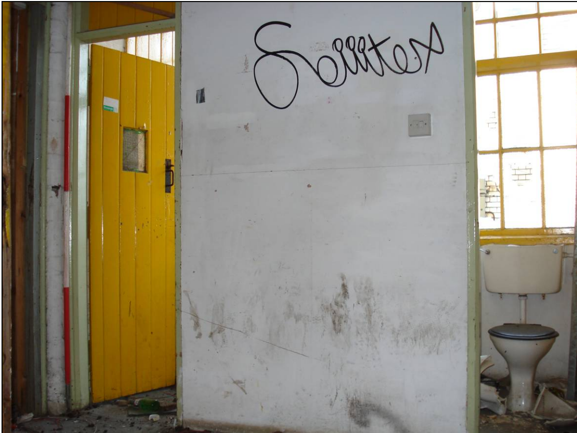
Figure 62: Lavatories, looking south (scale 2m)
