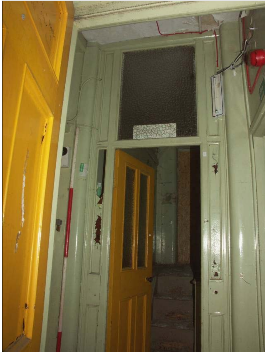
Figure 30: First floor's lobby of the southern wing, looking south (scale 2m)
