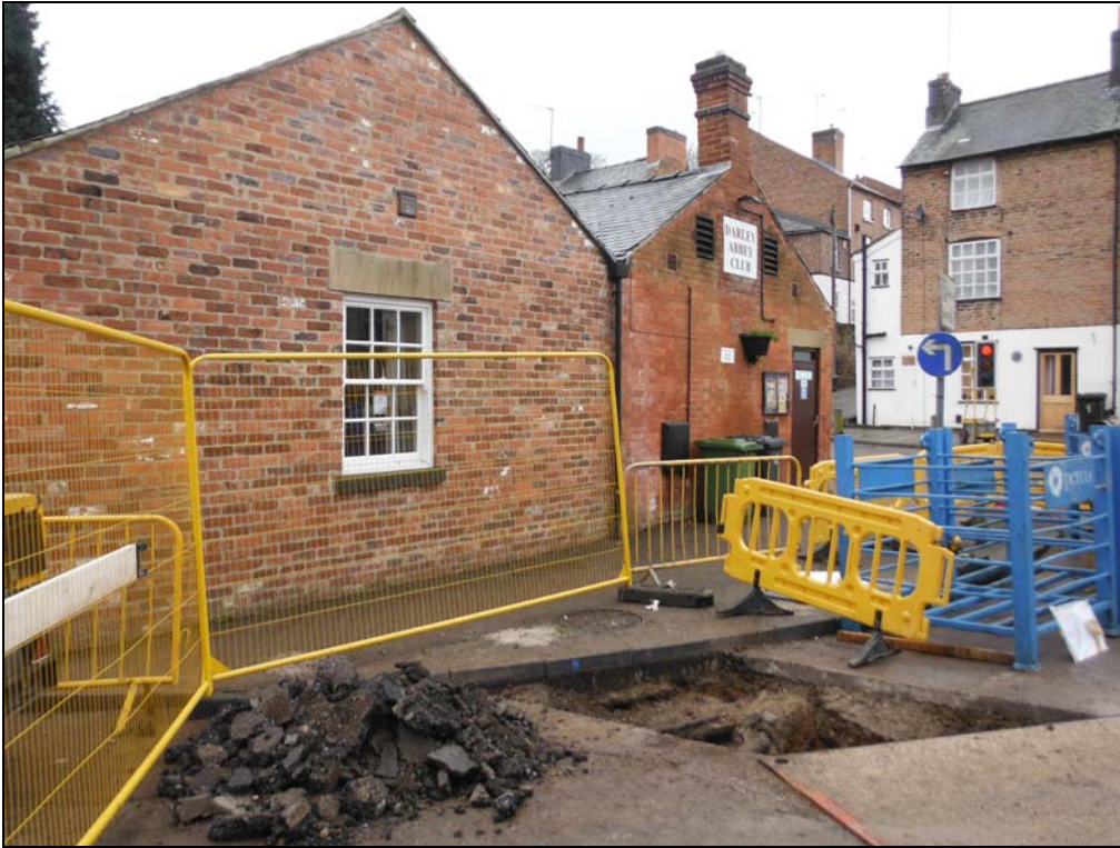
Figure 10: Trench 5 to the north of Darley Abbey Club, looking south-west
