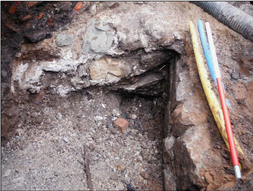
Figure 12: Wall (502) and later abutment wall (503), looking east (scale 1m)
