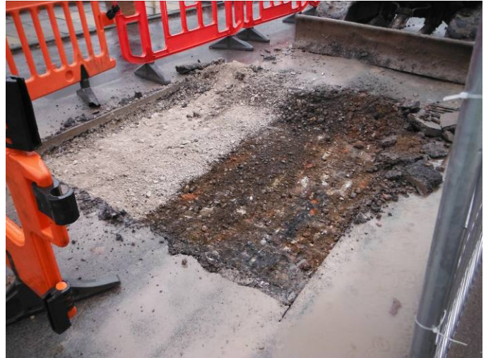
View of excavation area, trench 2
