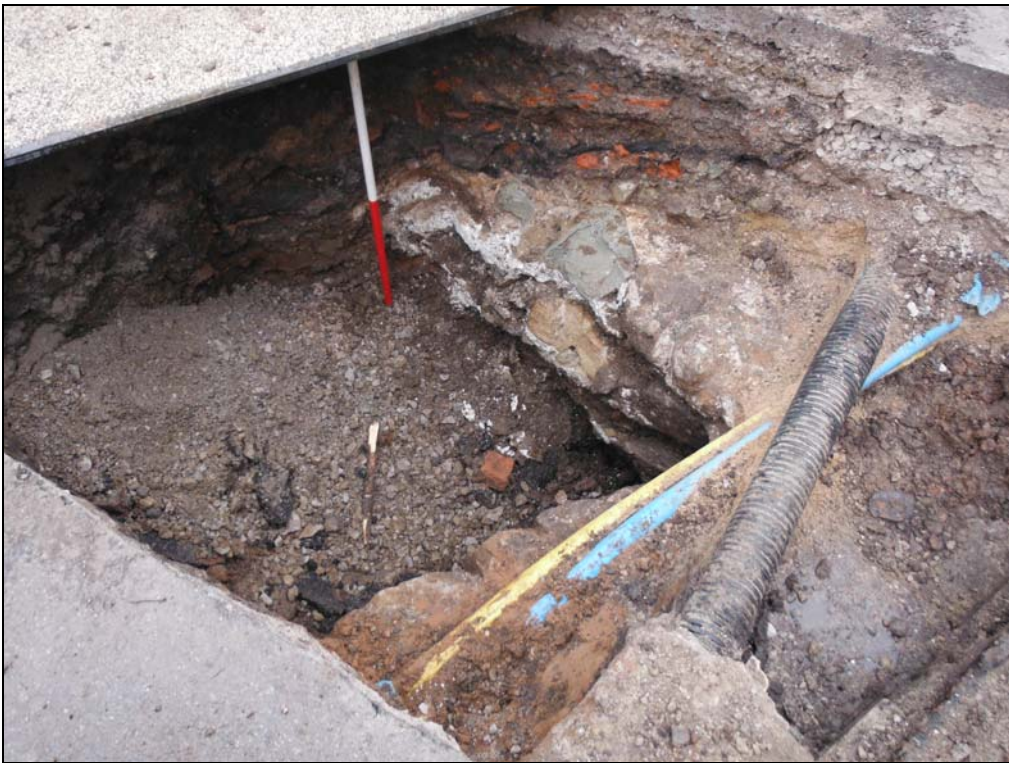
Figure 13: Wall (503), looking north-east (scale 1m)
