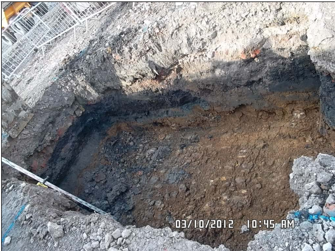
Figure 3: Foundation trench along the southern boundary of the site, looking west
