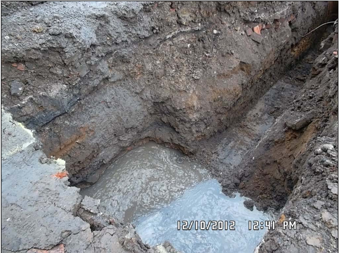
Figure 4: Foundation trench within the northern area of the site, looking north
